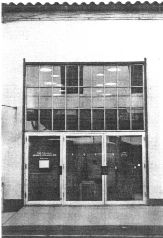
Storefront installed in the opening of a large door in Building A.
