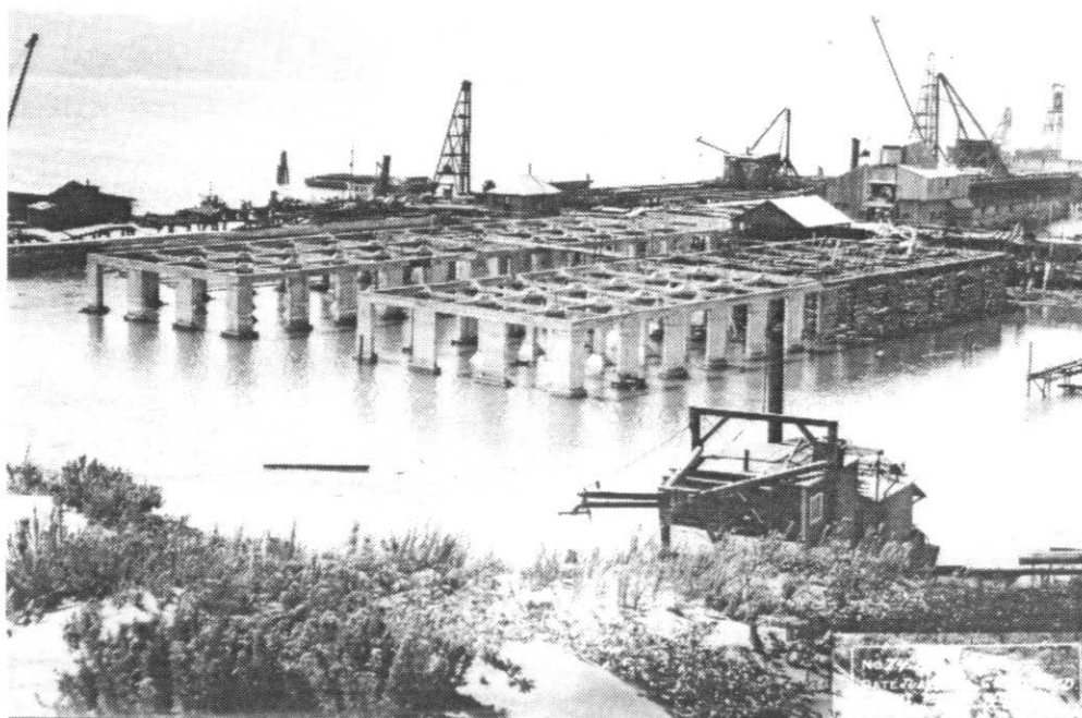
Warehouse foundations before backfilling, July 1, 1910
