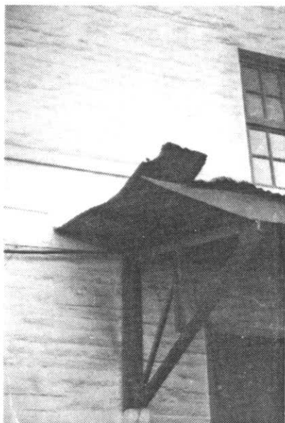
Damaged awning on Building 314
