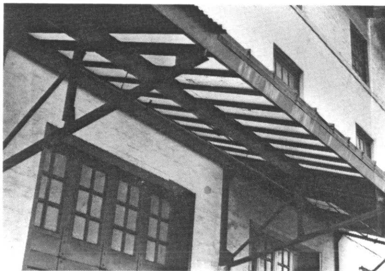
Translucent panel installed in awning.
