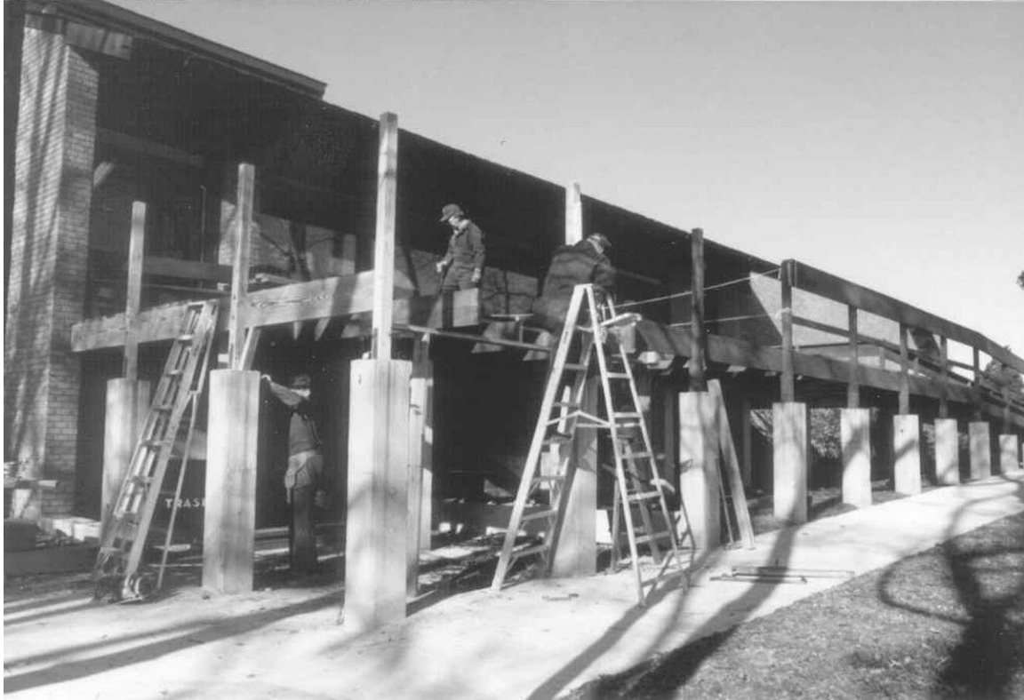
Image 46: The Visitor Center under construction in 1976, view from Popes Creek.
