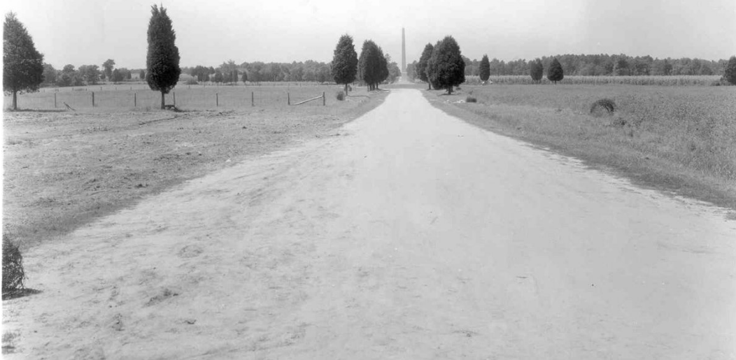
Image 22: Approach road, ca. 1931.
