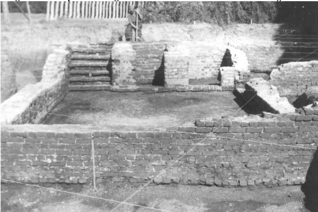
Image 12: Building X uncovered, ca. 1936.
