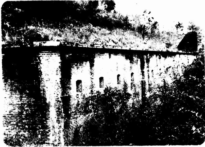
Lower part of masonry structure was in poor condition and repair to those parts was not reported until the late 1920's. It is proposed removal of the upper portion of structure to reduce excessive pressure on the masonry walls and to provide for the proper operation of the dam.
