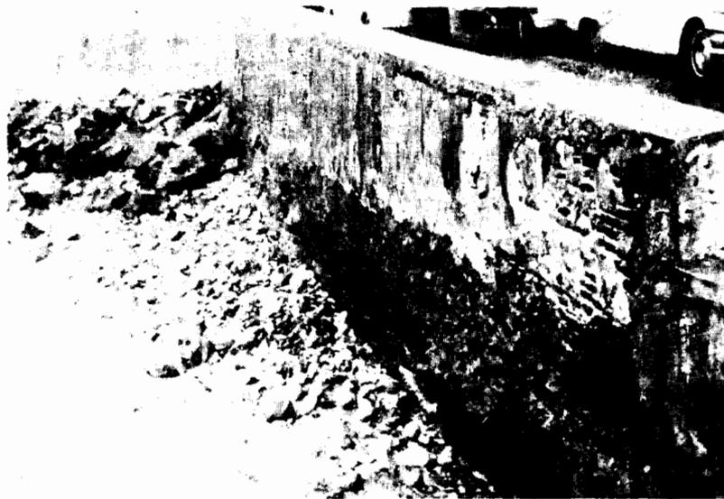
The erosion of the plaster from the face of the City Wall leaves the brick and stone work exposed to destructive weathering.
