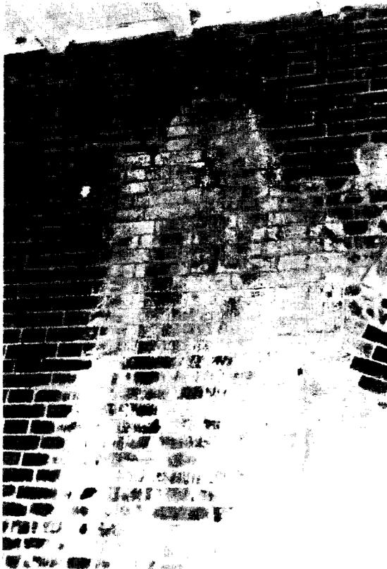
Conditions such as this have been caused by water entering from the terrace and roof. Waterproofing and flashing repair is needed.
