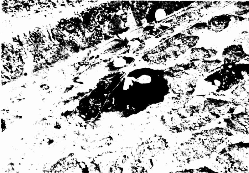
The softer stones used in the construction of San Cristobal have completely disintegrated. The extensive growth of vegetation also contributes to the present condition.
