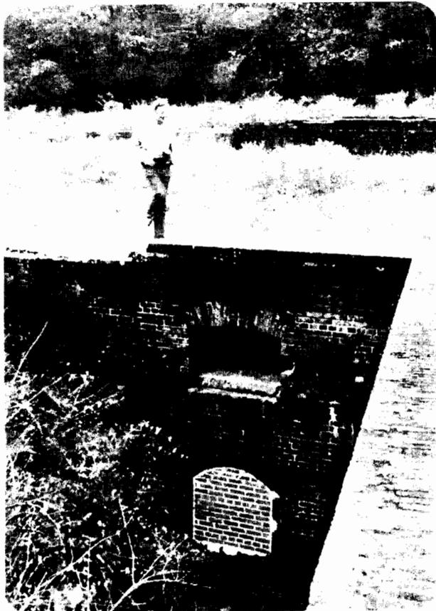
One of the lower spillways has been closed to prevent flooding of the dam. It will be opened and restored. Spillways will be built where shown on plan.
