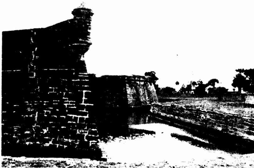
Cracking of the comina walls is undoubtedly due to foundation failure or movement over the years. The more serious areas will require repair and reinforcement to the foundation, in other areas repair and repointing will be sufficient to correct this damage.
