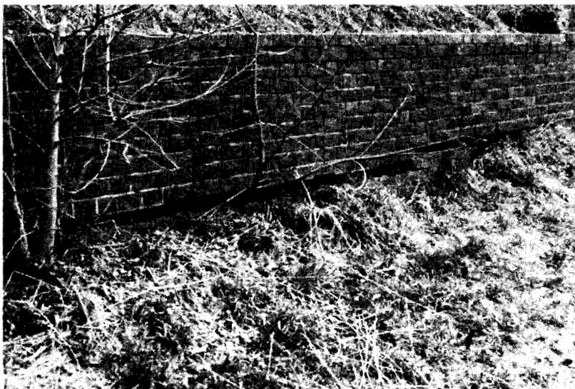
Note missing brick in east wall of southeast flank bastion.
