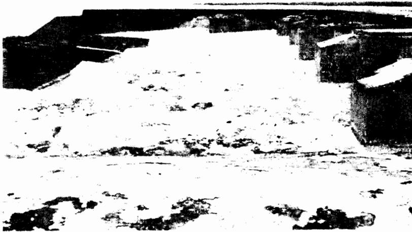
The exposed second floor, now acting as the roof, must be waterproofed and repaired if deterioration of the historic fabric is to be stopped.
