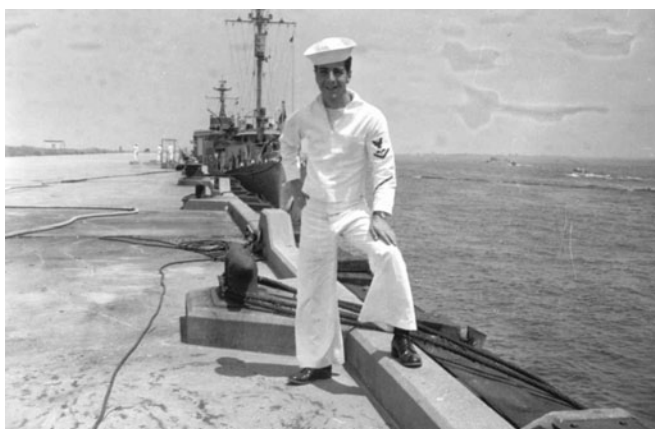
Figure 1.89: The marginal wharf with its concrete bulkhead and iron cleats, view looking east with Rockaway Inlet to the right, from a later photograph, c.1950. The identity of the sailor is not known. (Uncatalogued maintenance file photograph, Floyd Bennett Field, Gateway National Recreation Area.)
