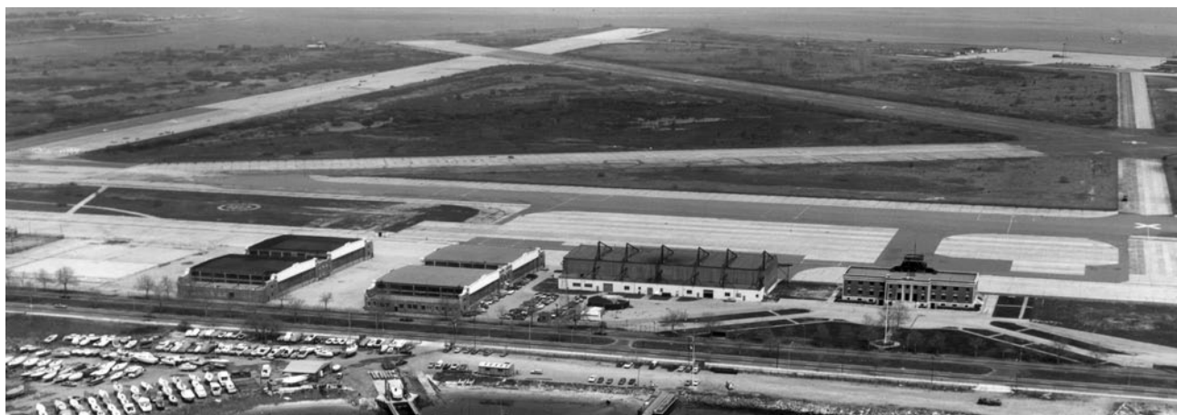
Figure 1.101: Looking east across Hangar Row showing the Air National Guard's nose hangar (265) built between the Administration Building and hangars 5-6 in 1965, from a later photograph, c.1992. In the rear is the apron that was enlarged by paving over turf between the taxiways most likely as part of the hangar construction. The World War II-era wing on the Administration Building was removed in c.1979. (Photograph 18888, Gateway National Recreation Area Museum Collection.)
