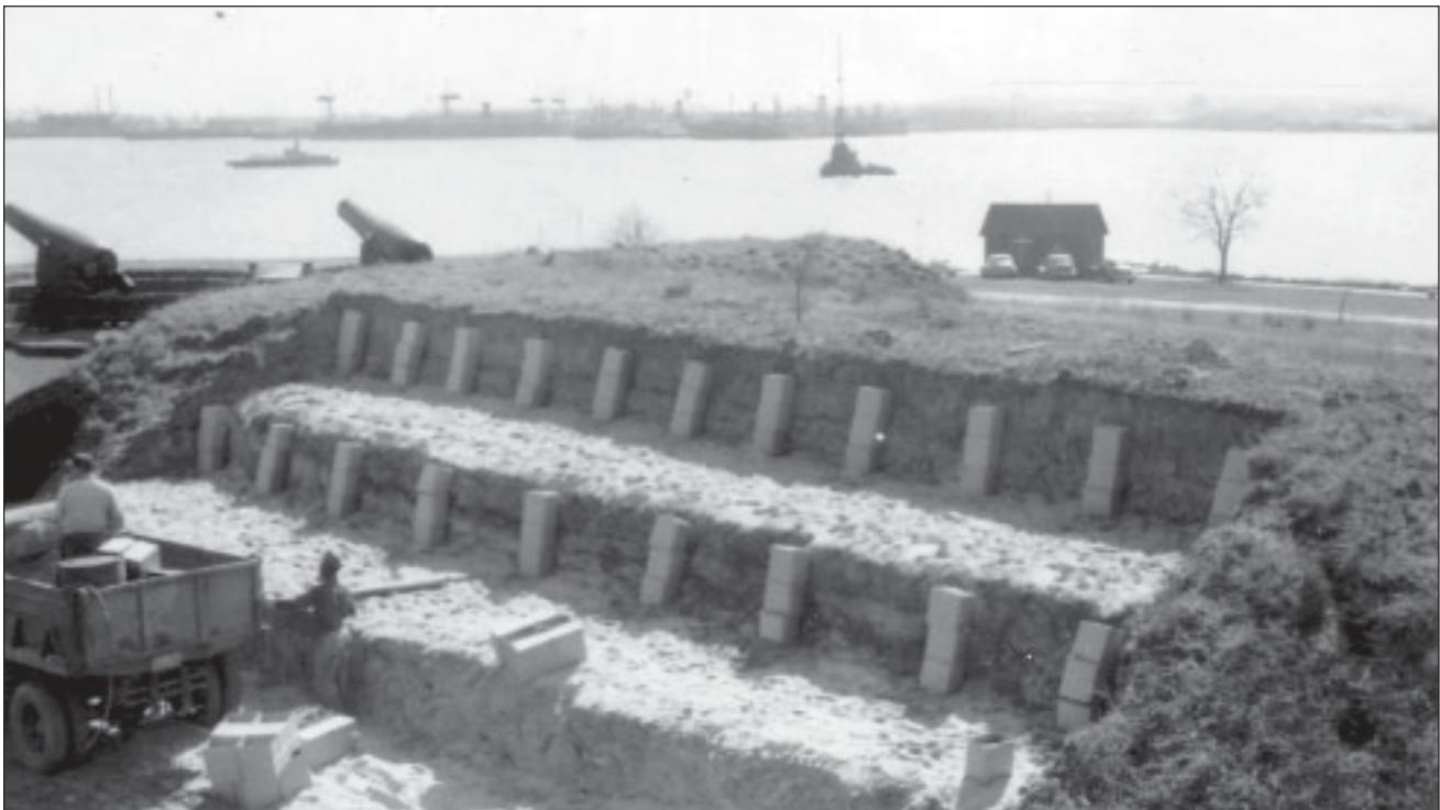
Figure 5.13. View of repairs and drainage improvements to fill covering Magazine 3, April 1950. This image shows the installation of interior drainage structures intended to reduce soil moisture. Small building at upper right is thought to be a temporary construction office. From, “Final Report on Repairing Slides in the Outer Ramparts...” 9 May 1950. Fort McHenry Library Special Collections.
