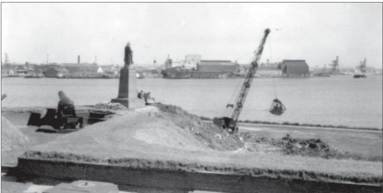
Figure 5.12. View of repairs underway to slope of exterior battery, April 1950. From, “Final Report on Repairing Slides in the Outer Ramparts...” 9 May 1950. Fort McHenry Library Special Collections.
