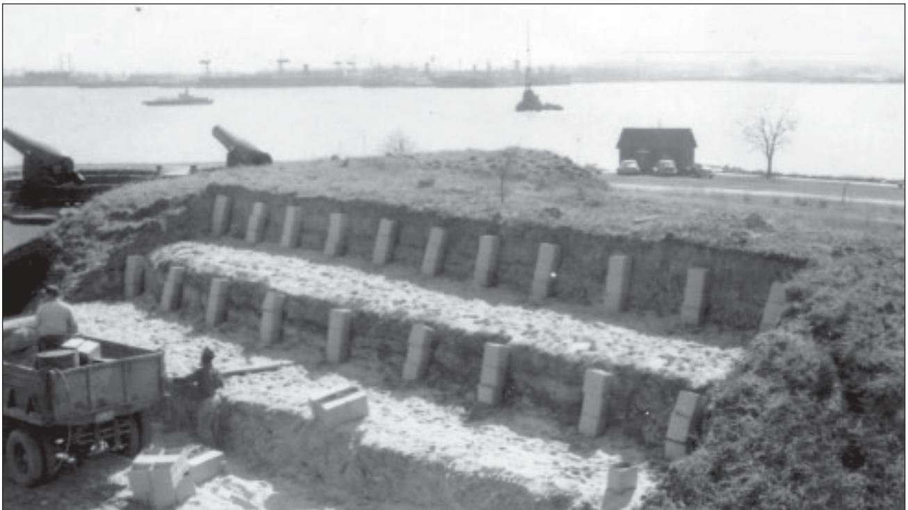
Figure 5.13. View of repairs and drainage improvements to fill covering Magazine 3, April 1950. This image shows the installation of interior drainage structures intended to reduce soil moisture. Small building at upper right is thought to be a temporary construction office. From, "Final Report on Repairing Slides in the Outer Ramparts..." 9 May 1950. Fort McHenry Library Special Collections.
