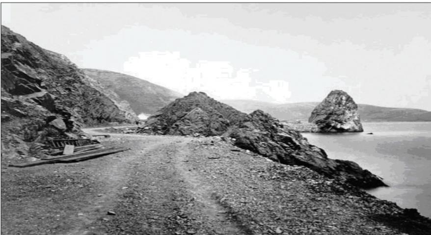
Once Engineer's Camp, the wharf and road were completed, the principal task before Mendell was to create a staging area for construction of the fort which would require a cut 230' deep on the face of a 250'-high cliff. Blasting at Lime Point was carried out in 1868-1869. Over twenty-five tons of gunpowder was used to remove the immense quantity of rock, estimated by Lt. Col. Mendell to amount to over one million cubic yards.<sup>17</sup>
