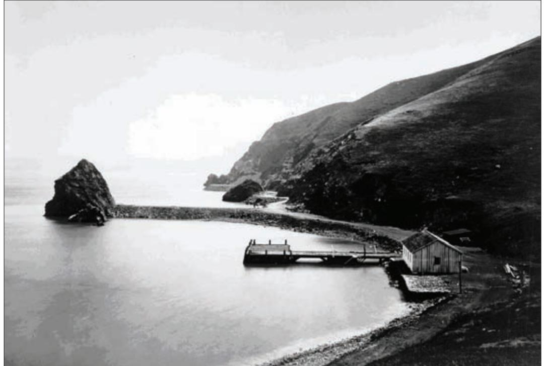
some protection to the cove from the currents of the open bay. Within this protected area, a small wharf was constructed which had a sixty-foot front of crib work covered with plank. (Photo SH1) Supplies and materials were barged in from San Francisco and unloaded at the wharf, and a steamer was used to transport personnel.<sup>15</sup>
