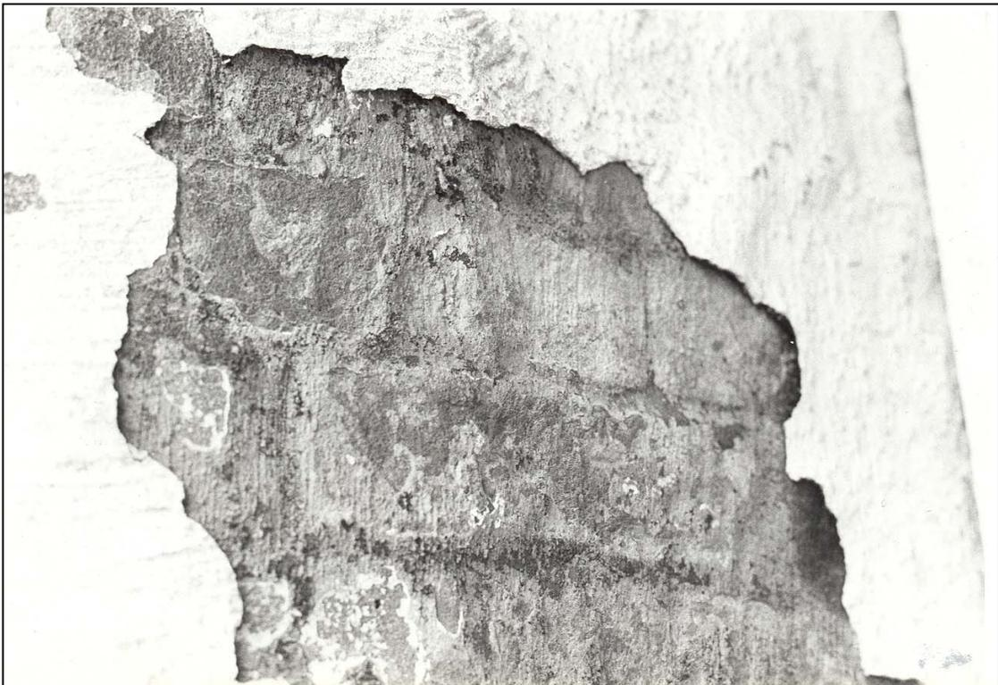
**Figure 104.** Tower interior: deterioration of wall whitewash (1982).
