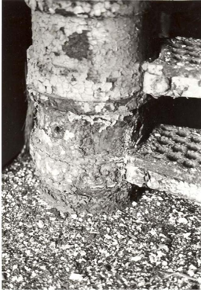
**Figure 145.** Tower interior: central column corrosion (1983).
