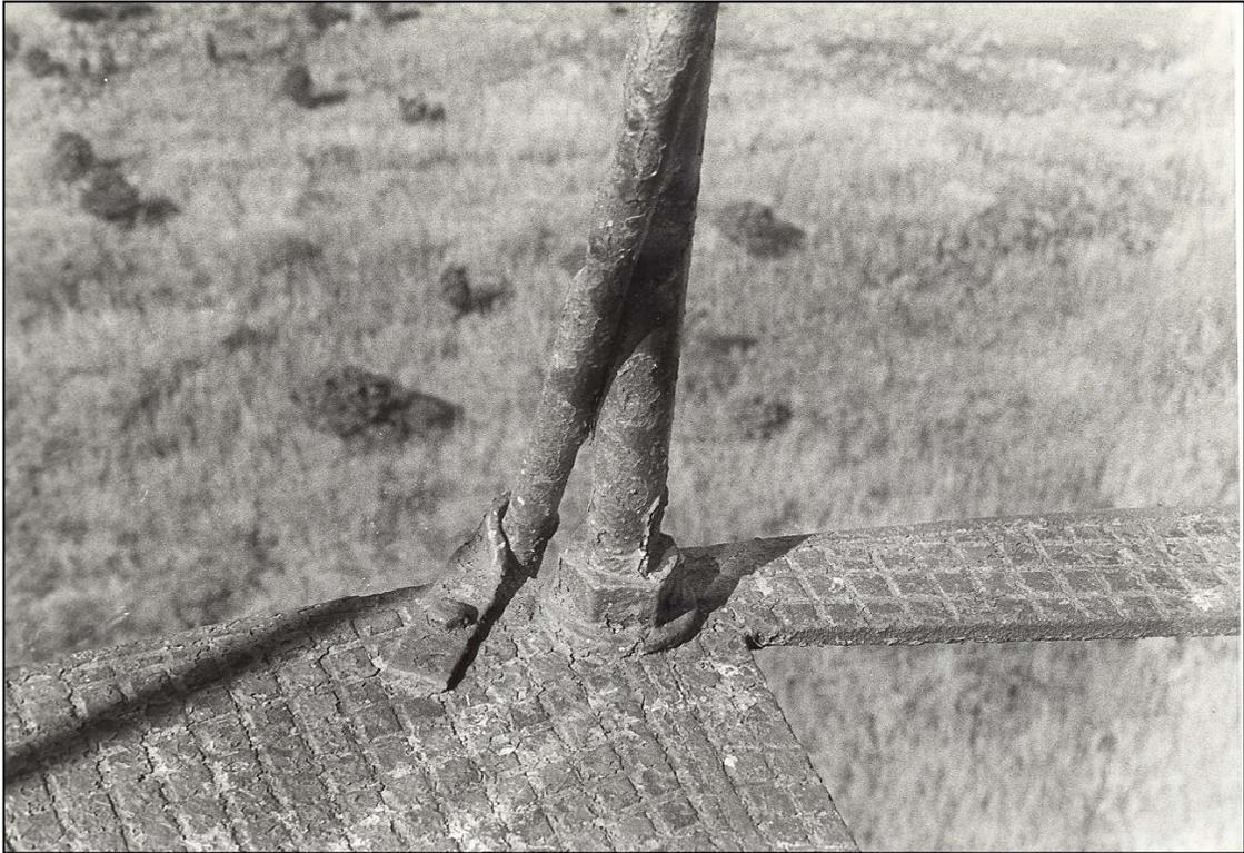
**Figure 198.** Tower exterior: diagonal brace tied to deck of upper balcony (1983).
