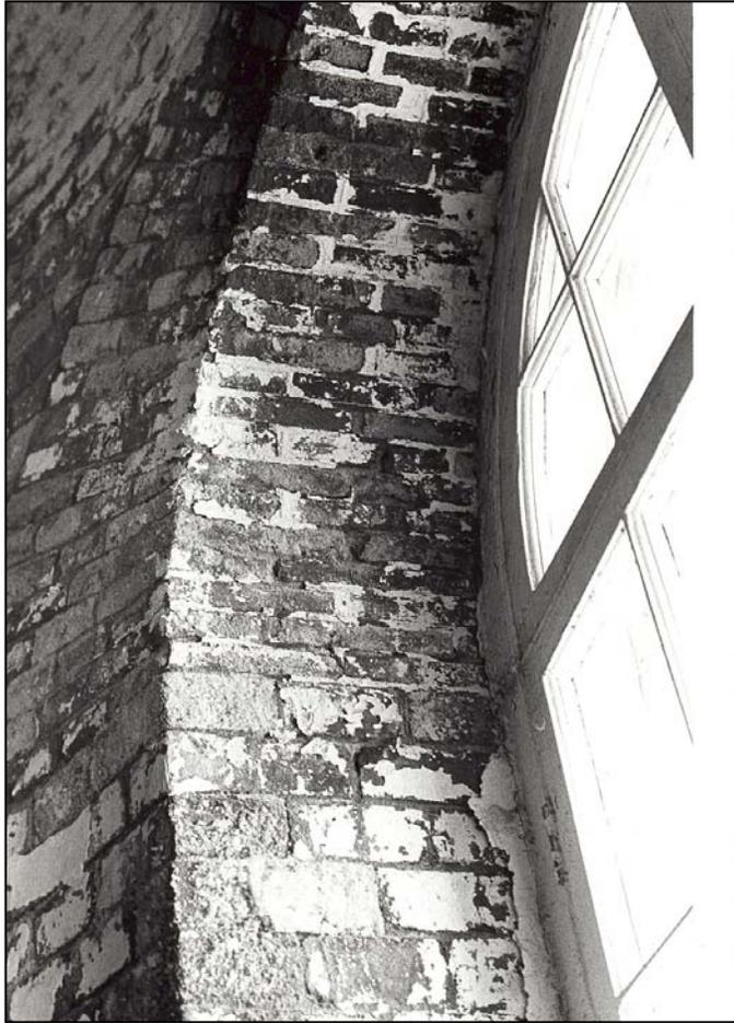
**Figure 102.** Tower interior: efflorescence of wall brickwork (1983).
