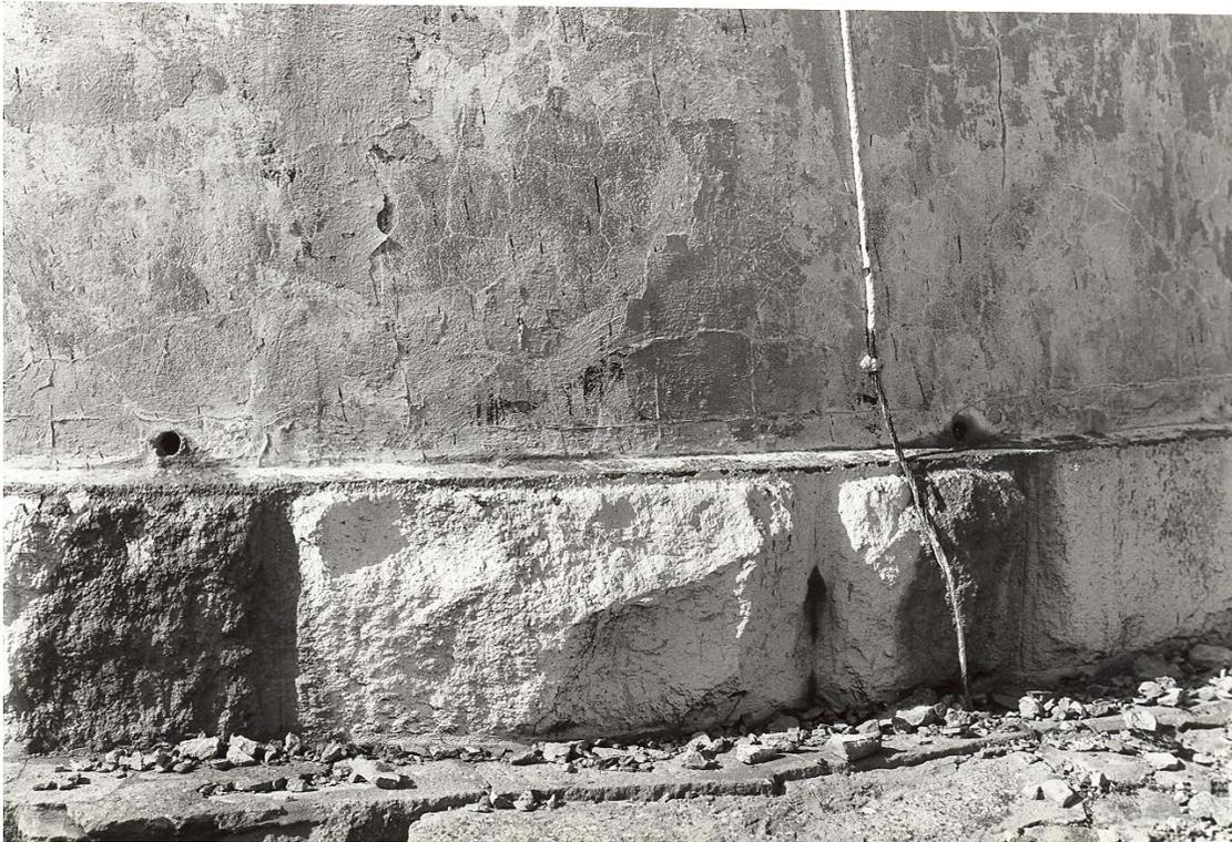
**Figure 206.** Tower exterior: lightning-rod cable at tower base (1983).
