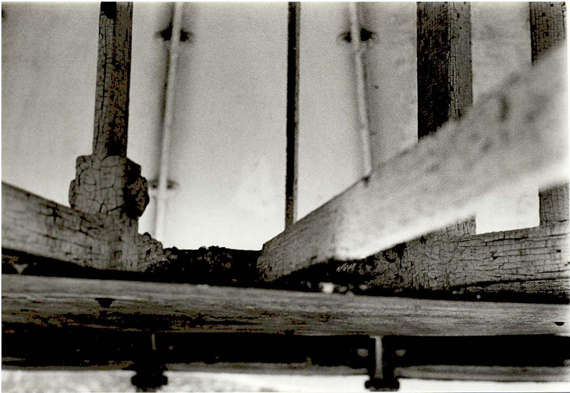
**Figure 191.** Tower interior: lantern roof, with lower frame, tie rods, and hub above plywood disk (1982).
