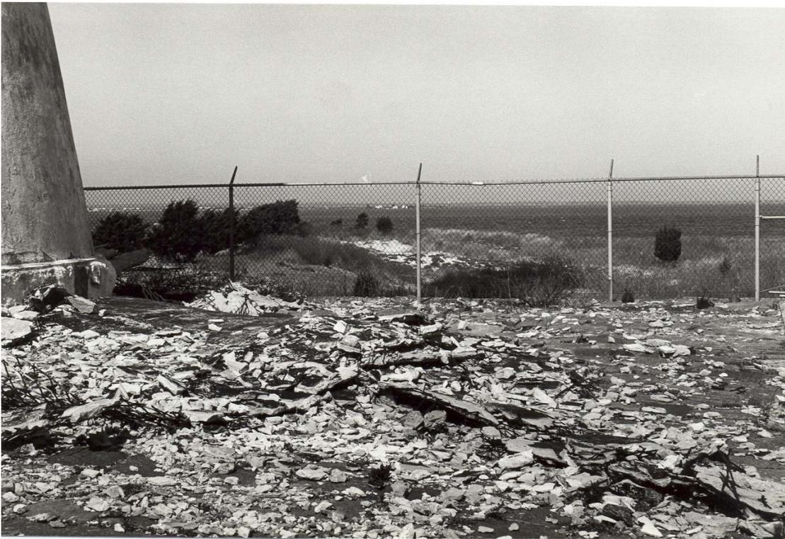
**Figure 89.** Tower exterior: protective coating debris at base of tower (1983).
