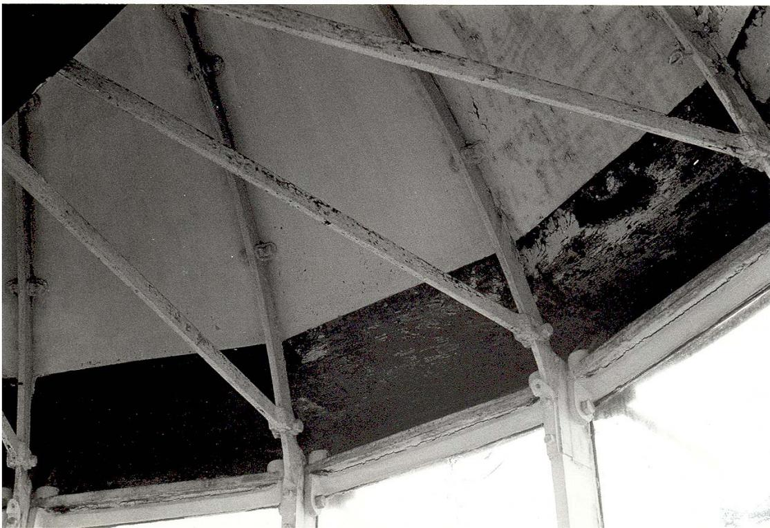
**Figure 189.** Tower interior: lantern roof, junction of spider frame and lower frame (1982).
