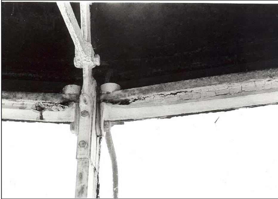
**Figure 193.** Tower interior: lantern cornice area, deterioration of fittings (1983).
