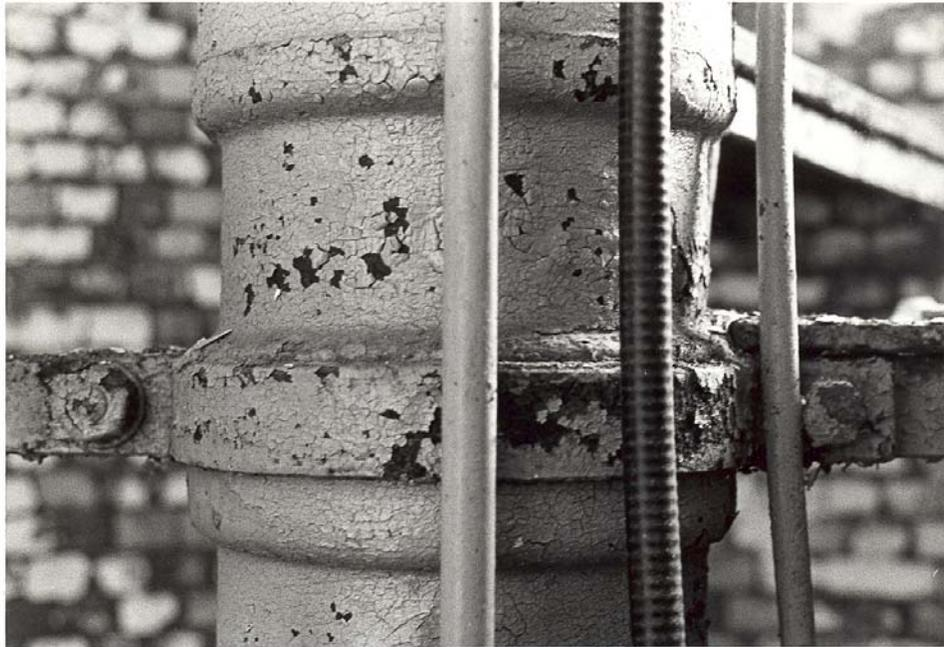
**Figure 153.** Tower interior: conduits along central column (1983).
