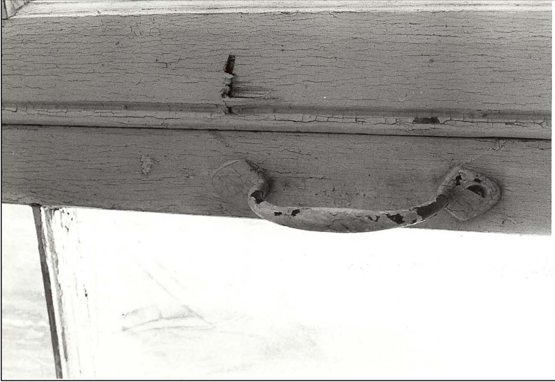
**Figure 177.** Tower interior: typical sash pull for exterior storm sashes (1983).
