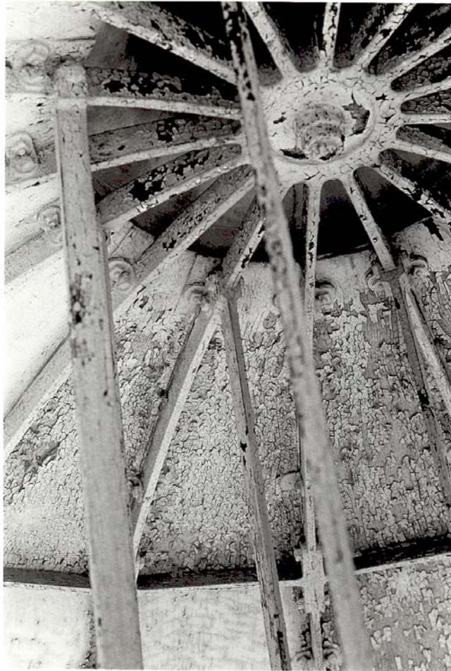
**Figure 190.** Tower interior: lantern roof, spider frame, and suspension rods (1982).
