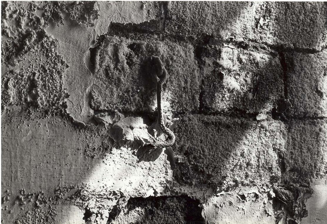
**Figure 179.** Tower interior: typical hook to hold sashes open (1983).
