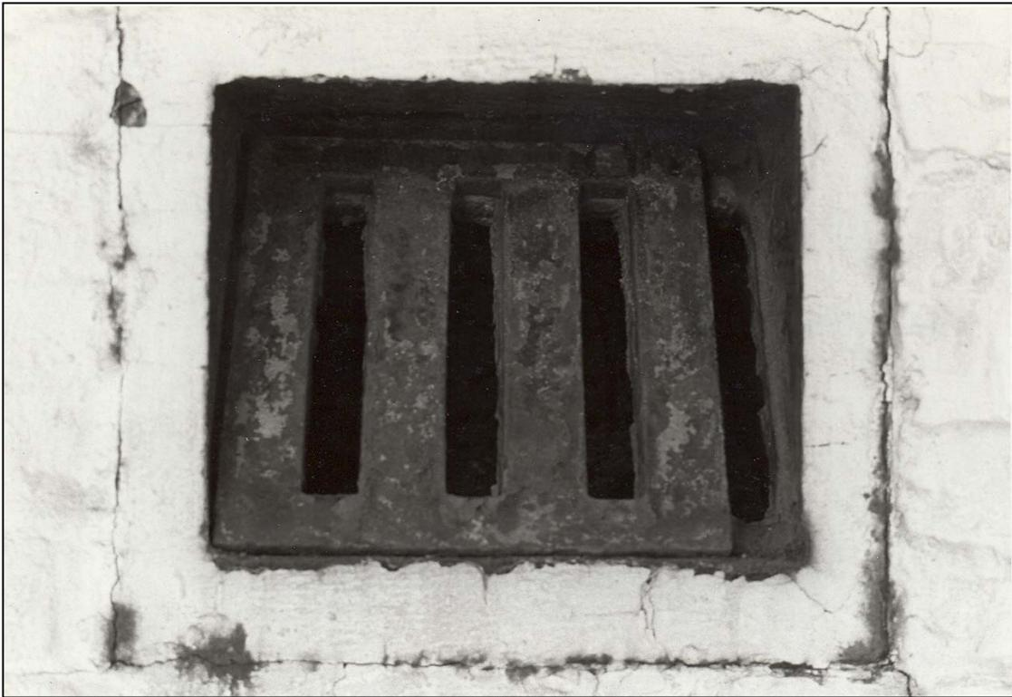
**Figure 100.** Tower interior: Watch Room vent box, open (1983).
