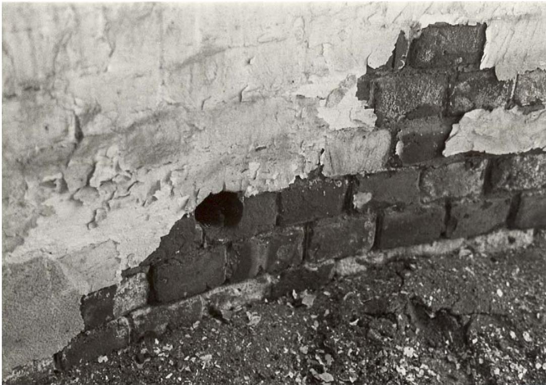
**Figure 95.** Tower interior: wall ventilation holes at ground level (1983).
