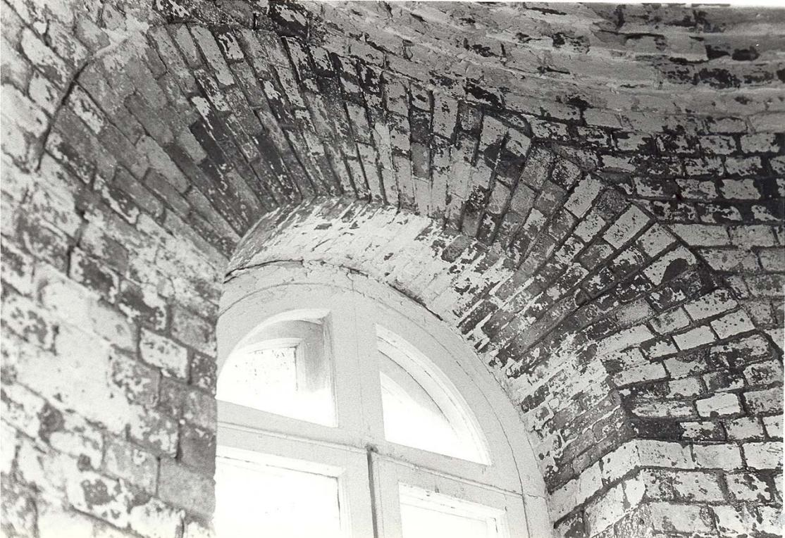
**Figure 98.** Tower interior: typical brick arch over windows (1983).
