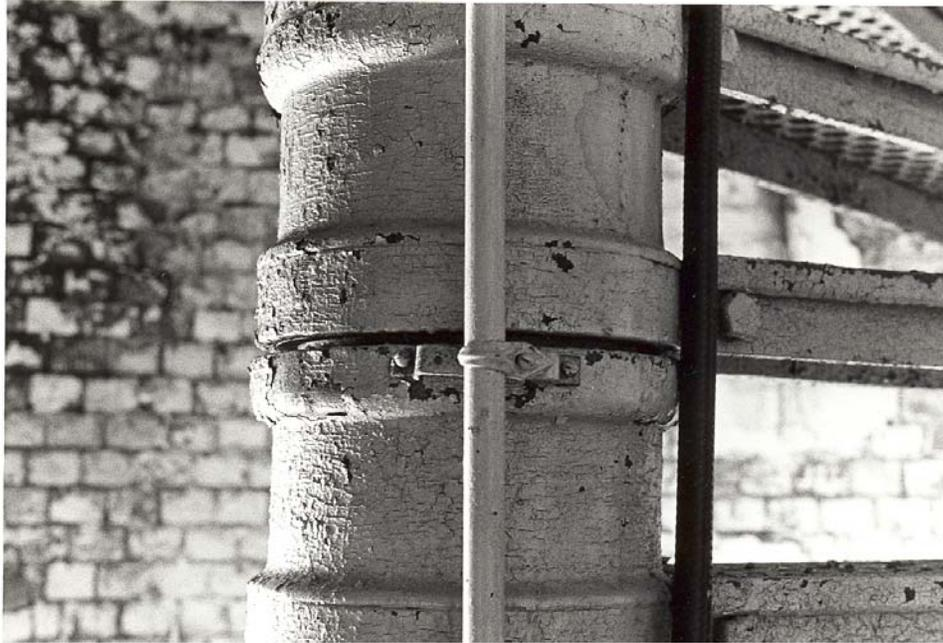
**Figure 146.** Tower interior: central column, seam separation (1983).
