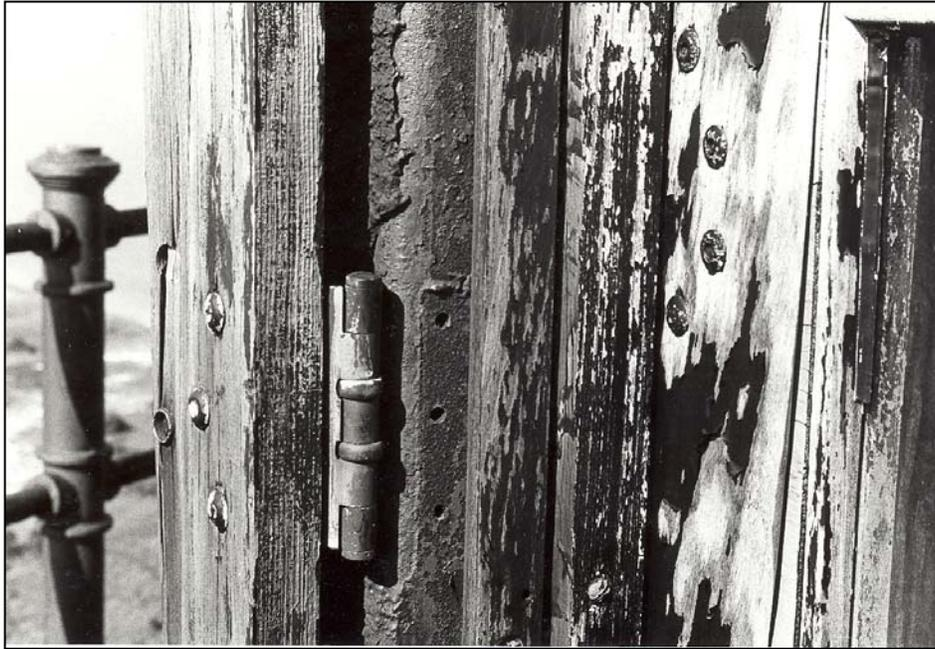
**Figure 170.** Tower exterior: lower balcony doorway to Watch Room, with iron frame and evidence of early hardware (1983).
