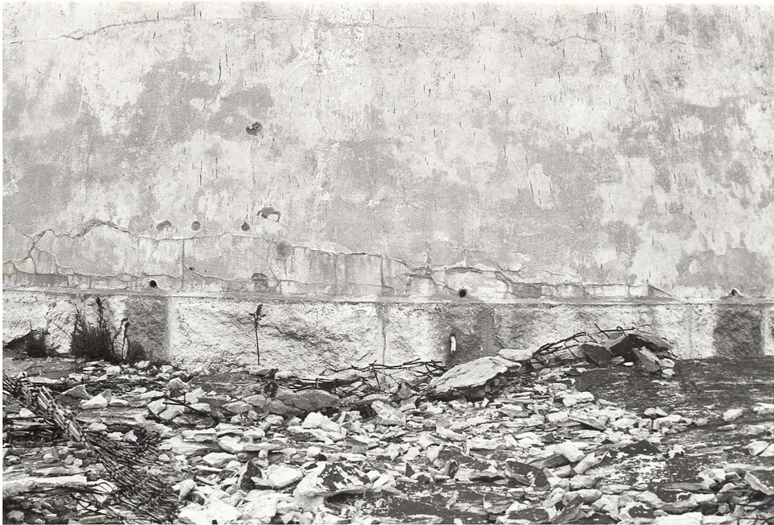
**Figure 80.** Tower exterior: plinth with ventilation holes (1983).
