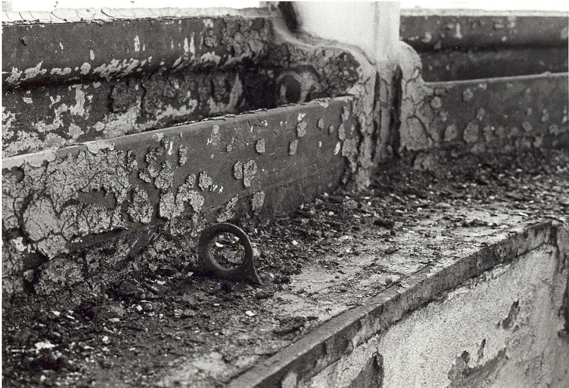
**Figure 127.** Tower interior: opening in lantern floor, traces of former trapdoor (1982).
