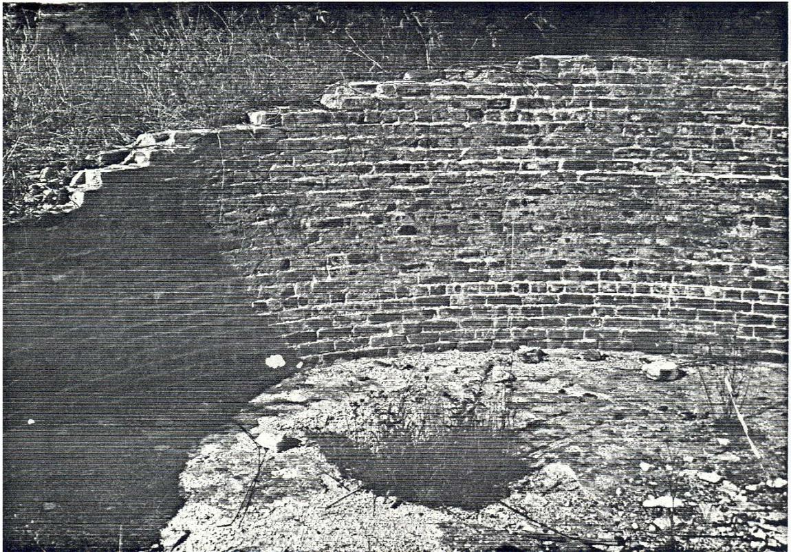
**Figure 5.** First Fire Island lighthouse: brick interior wall.
