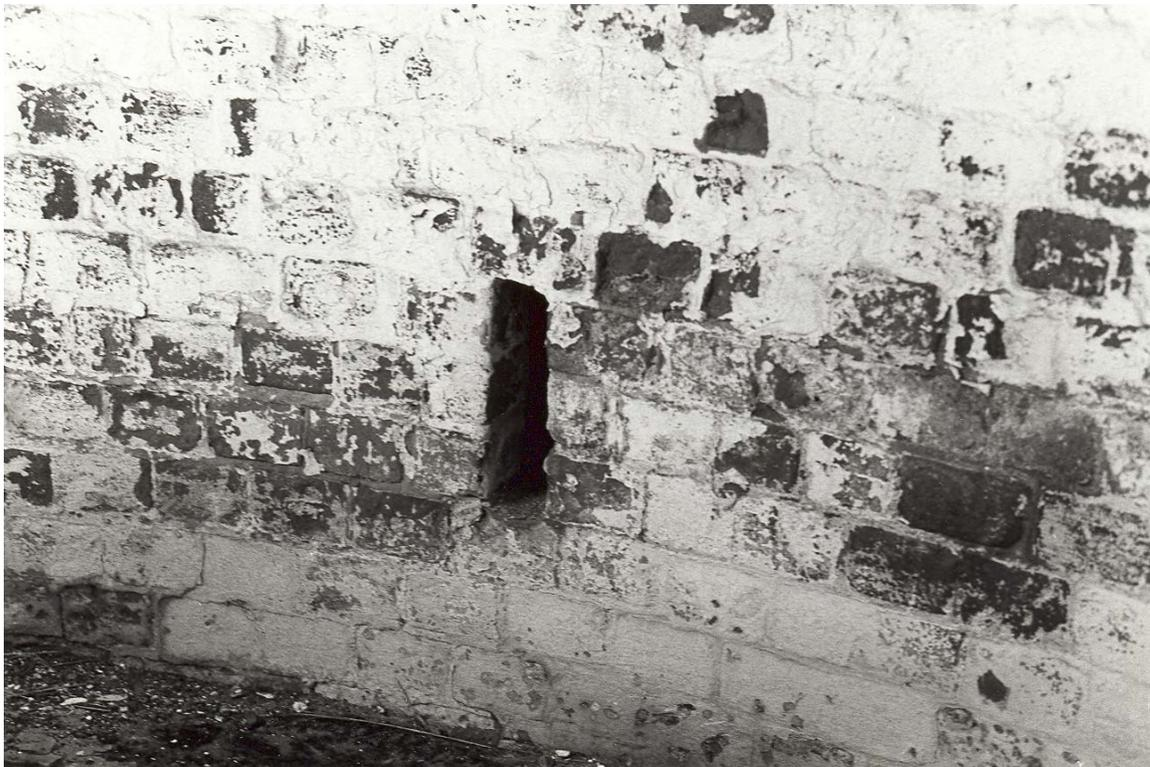
**Figure 96.** Tower interior: wall ventilation slots at upper levels (1983).
