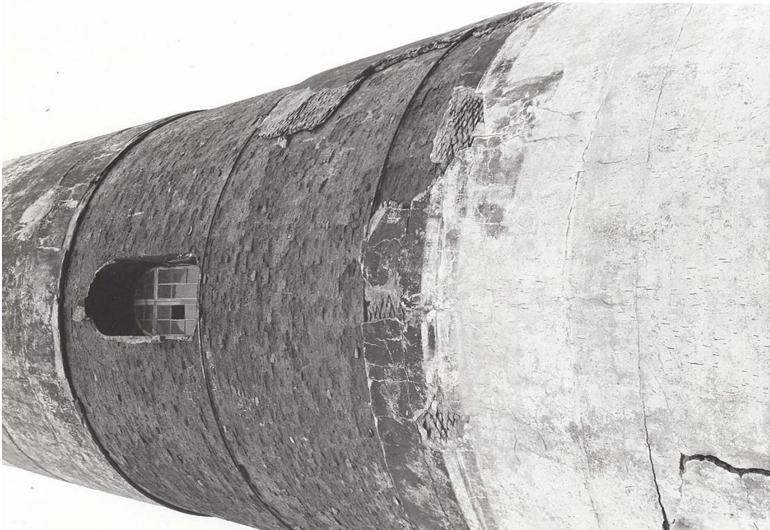
**Figure 86.** Tower exterior: deteriorated coating and exposed brickwork (1982).
