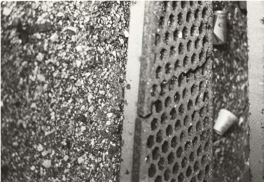
**Figure 135.** Tower interior: main stairway, deterioration of steps (1983).
