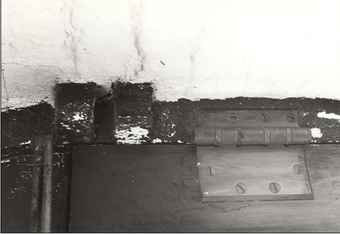
**Figure 169.** Tower interior: Watch Room doorway to lower balcony, with early pintles and later hinges (1983).
