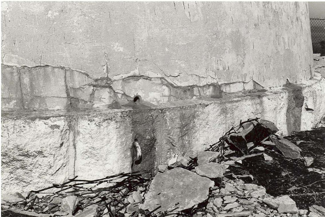
**Figure 81.** Tower exterior: plinth, ventilation holes, and anchor (1983).
