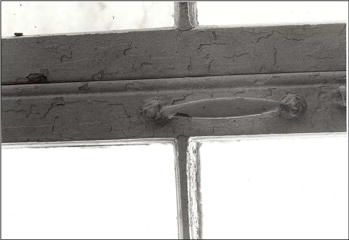
**Figure 176.** Tower interior: typical sash pull for interior sashes (1983).
