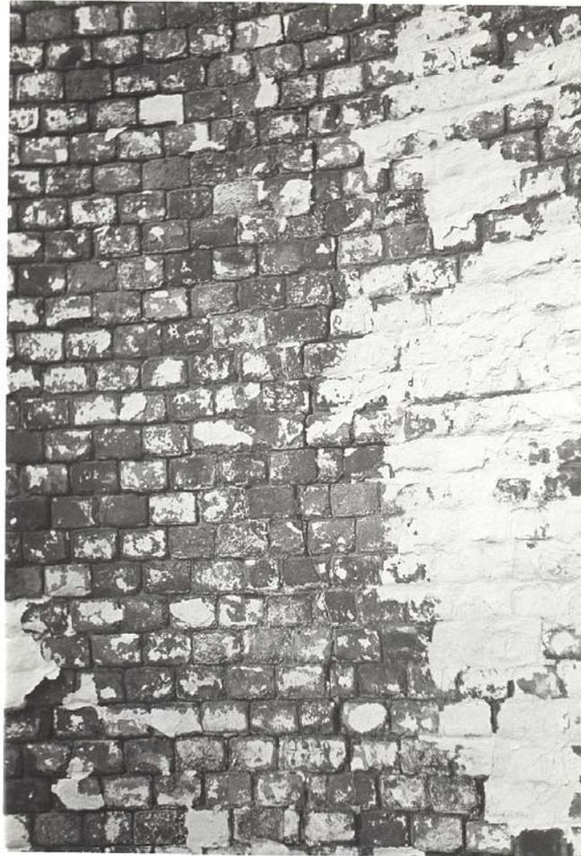
**Figure 105.** Tower interior: vertical crack in wall brickwork (1983).
