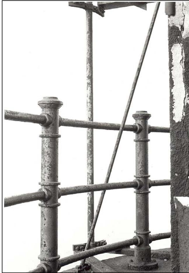
**Figure 197.** Tower interior: diagonal brace at lower balcony (1982).
