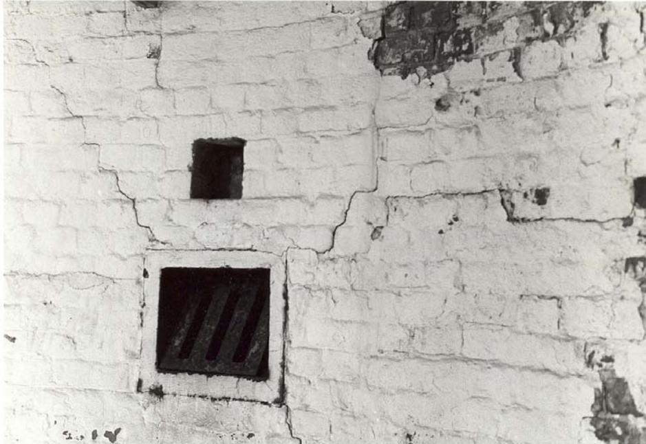
**Figure 106.** Tower interior: Watch Room, cracks in wall brickwork (1983).
