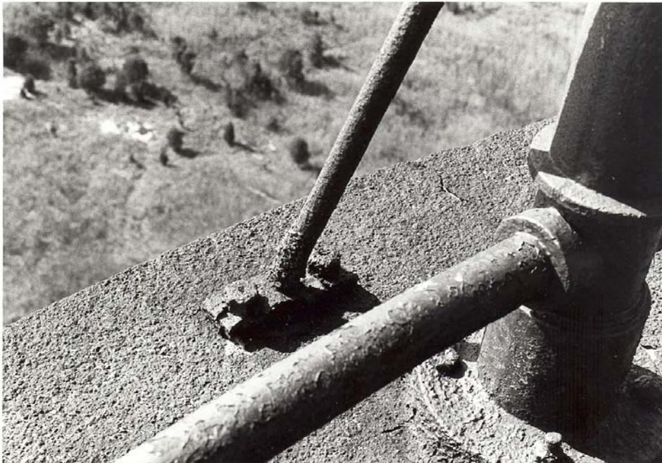
**Figure 196.** Tower interior: diagonal brace bolted to deck of lower balcony (1983).
