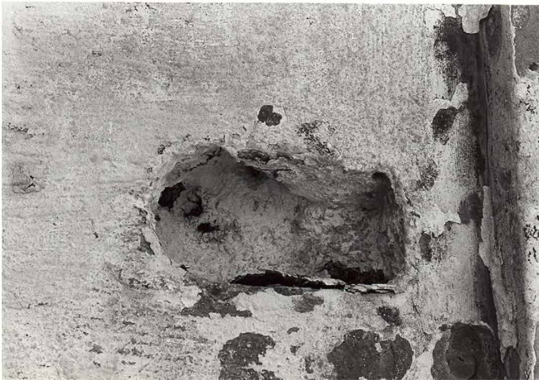
**Figure 162.** Tower interior: entrance doorway, east jamb area recessed for doorknob (1983).
