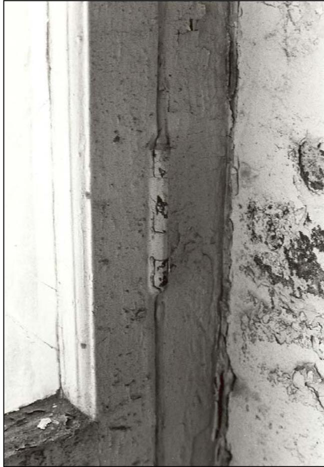
**Figure 175.** Tower interior: typical butt hinge for interior and exterior storm sashes (1983).
