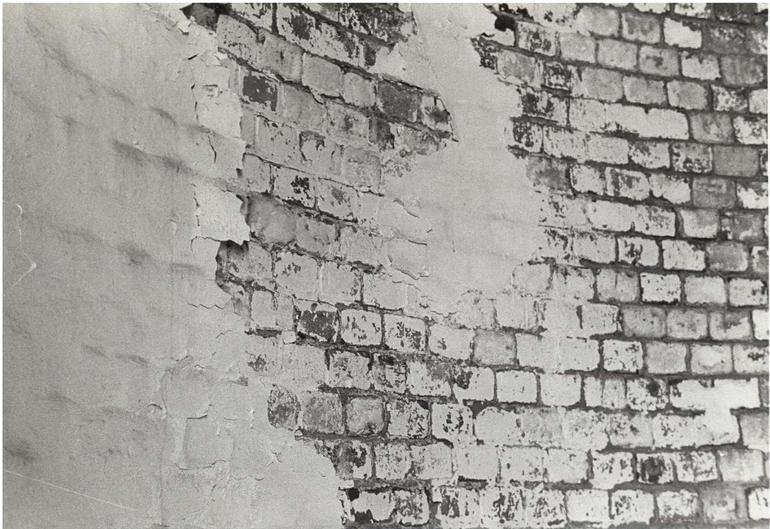
**Figure 103.** Tower interior: deterioration of wall whitewash (1982).
