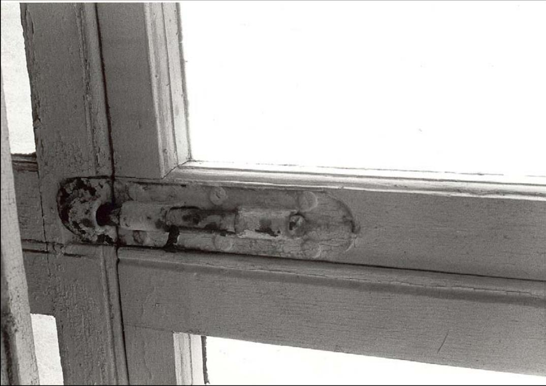
**Figure 180.** Tower interior: bolt latch at top of exterior storm sashes (1983).
