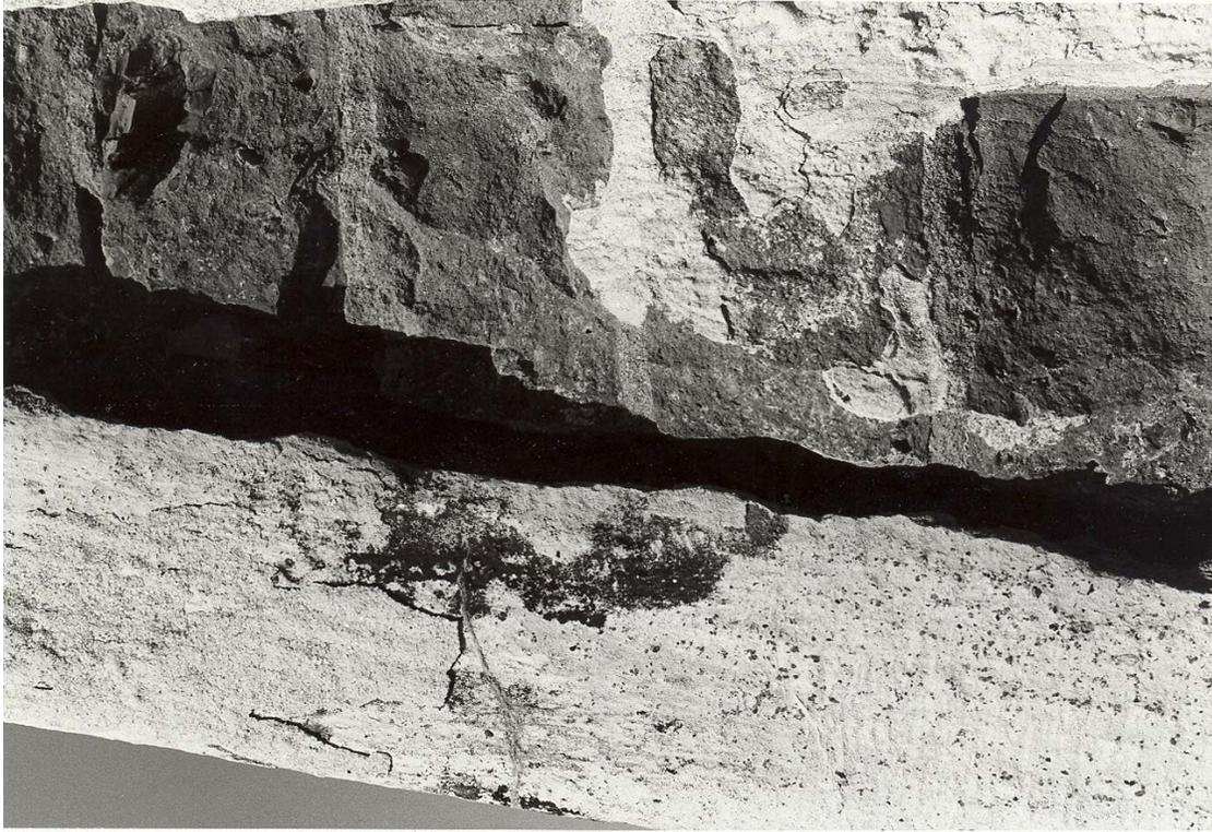
**Figure 87.** Tower exterior: coating separating from brickwork at entrance (1983).
