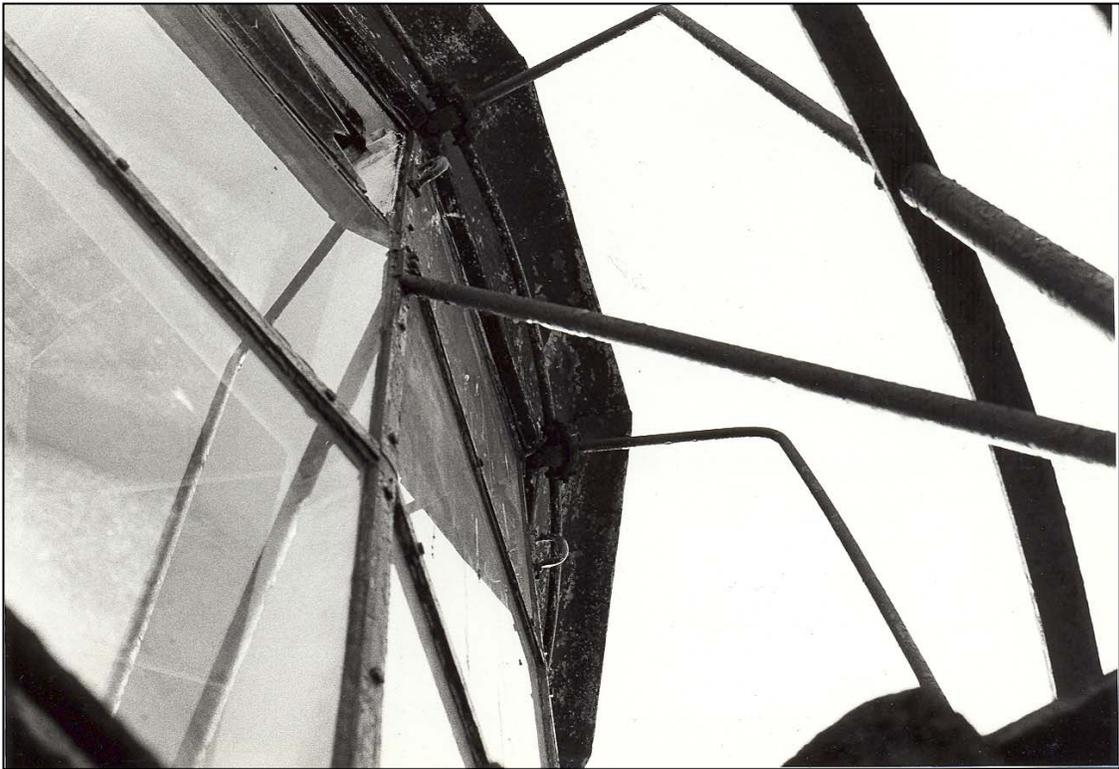
**Figure 199.** Tower exterior: diagonal brace bolted to side of lantern, and railing of upper balcony (1983).
