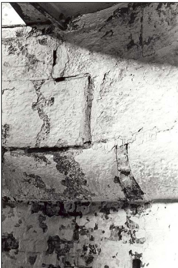
**Figure 94.** Tower interior: granite cornice in Service Room (1983).
