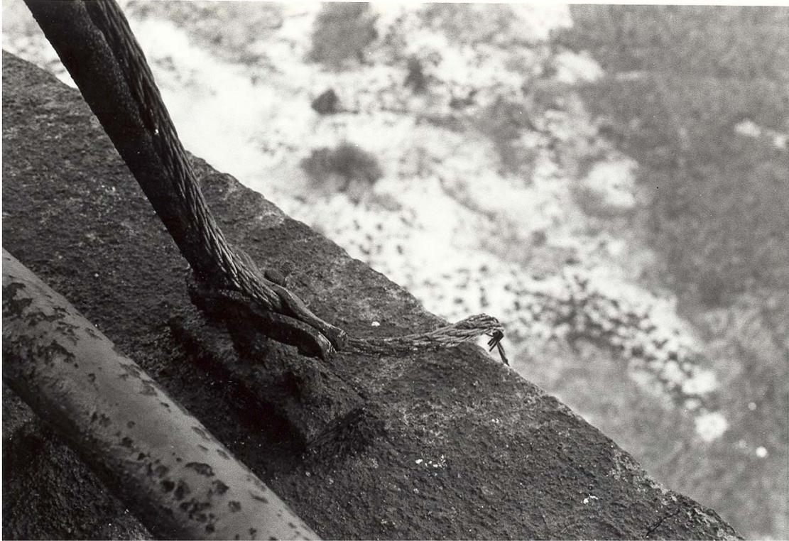
**Figure 205.** Tower exterior: lightning-rod cable at lower balcony (1983).
