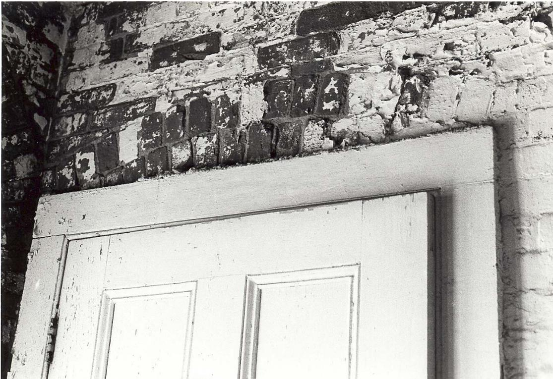
**Figure 97.** Tower interior: brick arch over doorway in sixth-landing room (1983).
