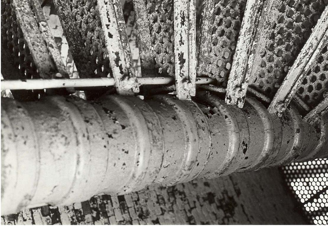
**Figure 136.** Tower interior: main stairway, deterioration of paint (1983).
