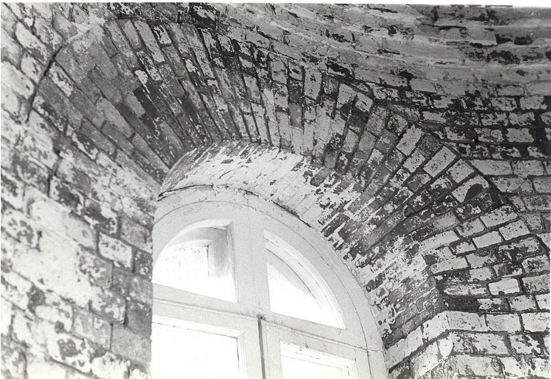
**Figure 98.** Tower interior: typical brick arch over windows (1983).
