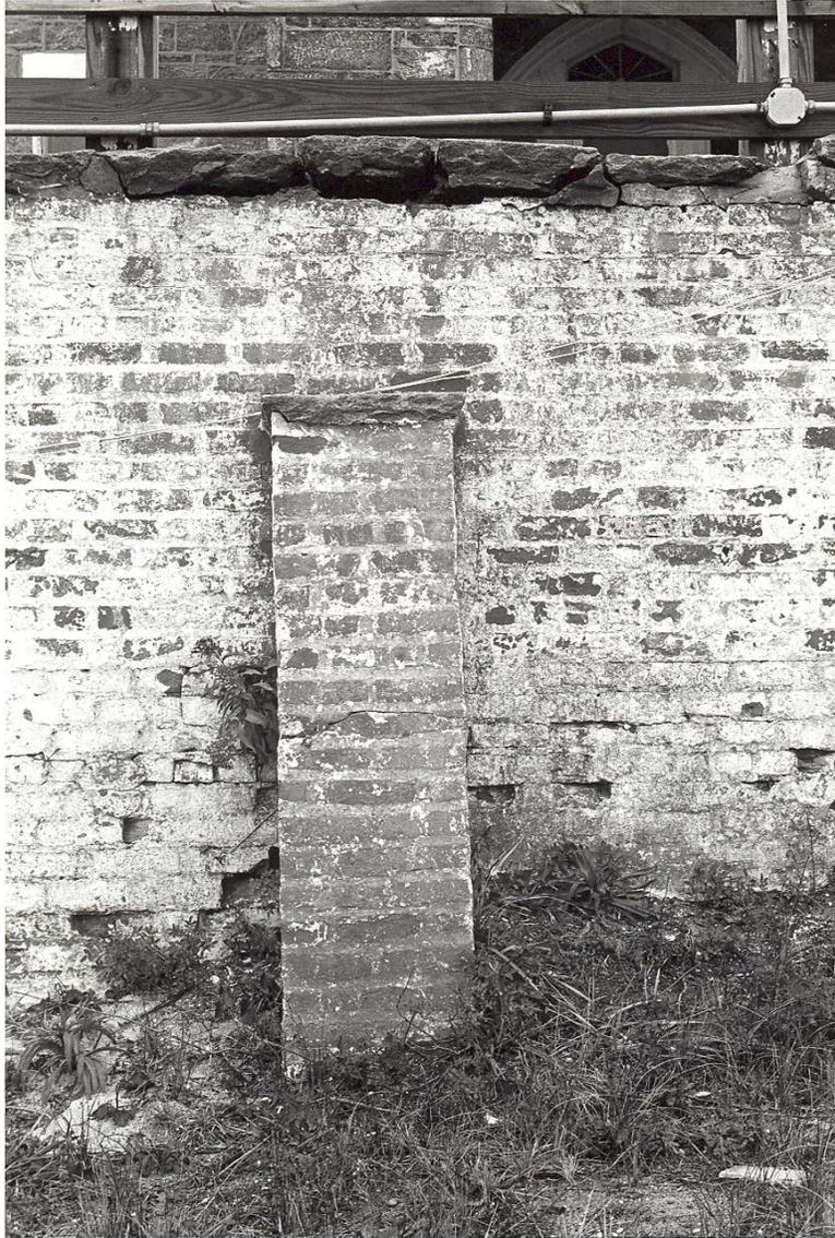
**Figure 52.** Terrace: south embankment wall, brick buttress (1983).
