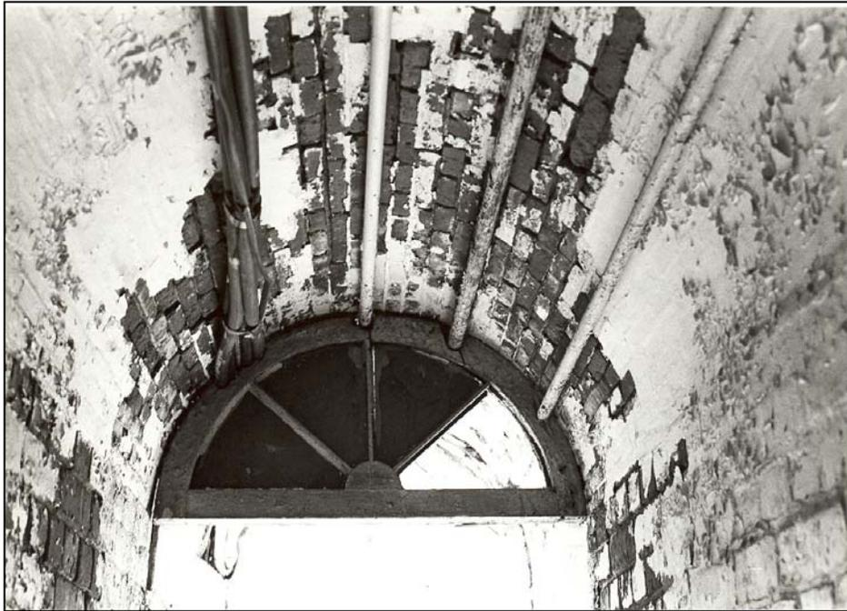
**Figure 151.** Tower interior: conduits entering through entrance-doorway fanlight (1983).
