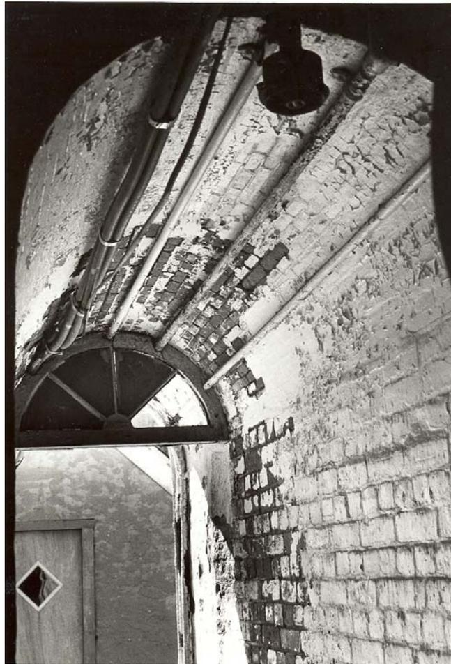
**Figure 152.** Tower interior: conduits at ceiling of entrance hallway (1983).
