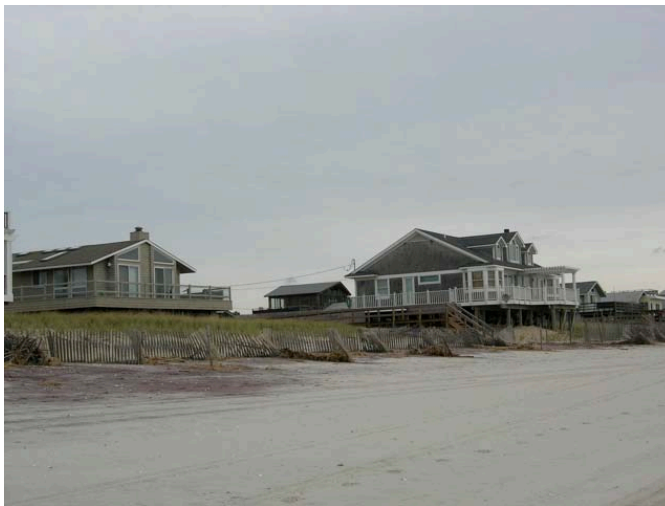
Figure 3-2: Oceanfront houses on Fire Island atop the area where the dune should be. The presence of the buildings has prevented the dune from forming and leaves them exposed to severe damage in the next storm.
