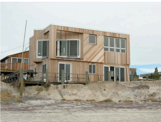
Figure 3-3: A nonconforming building being constructed on Fire Island atop the dune line, amid storm damage. The scoured beach directly in front of the house is evidence of a recent storm.
