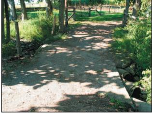
Figure 2.98. The pipe culvert bridge between Farms #1 and #2 is historic but has exacerbated erosion by channeling water. (Photo by OCLP, 2005)
