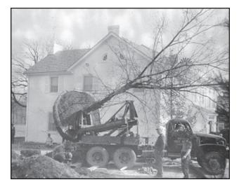
Fig. 2.59. Installation of elm with a large tree spade north of house. (Walter West collection, EISE NHS files, #1123)
