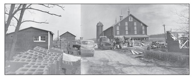
Figure 2.13. Stockpiling materials near the Redding garage for use during construction, view from the south toward the barn, spring 1954, two images combined into one panorama. (Gettysburg Times, EISE NHS files, #2784 & #2789)
