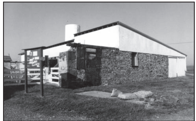
Figure 4.12. Remains of bank barn on Farm #2. (Photo by OCLP, 2002)
