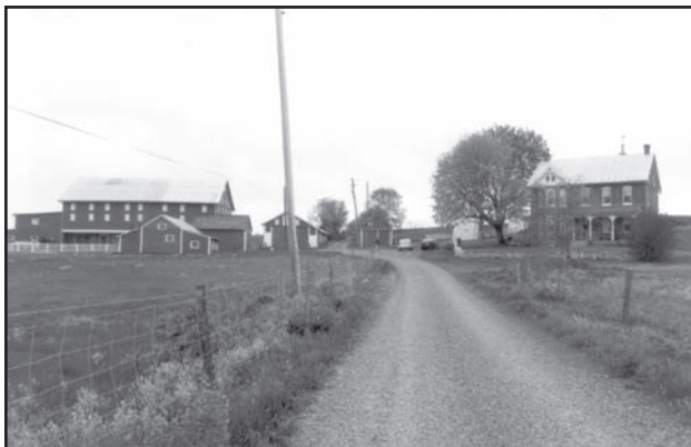
Figure 4.24. Entry lane leading to the Clement Redding Farm. (Photo by OCLP, 2002)
