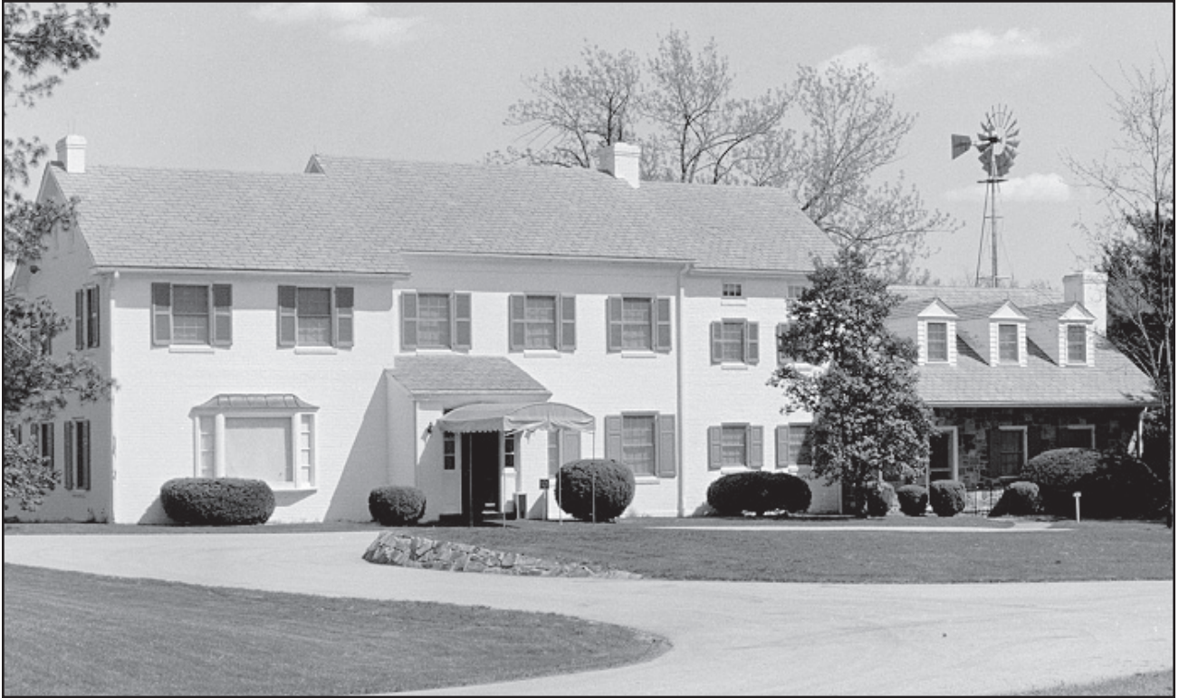
Figure 4.10. Front elevation of the Eisenhower home with the black locusts still missing from the front lawn circle, view toward southeast, spring 1988. (EISE NHS files, #3589)
