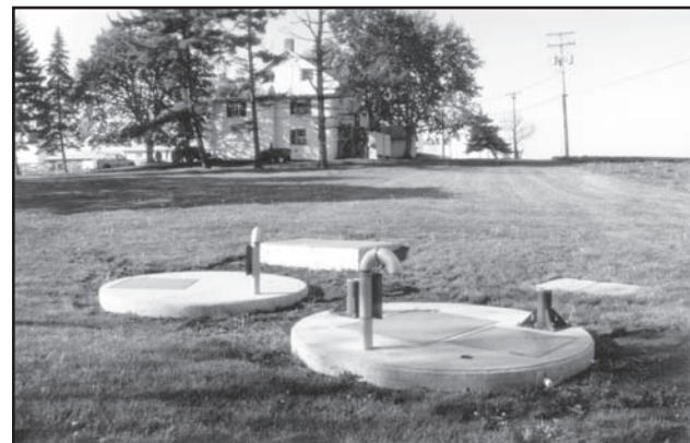
Figure 4.16. Detail of new septic system installed on Farm #2. (Photo by OCLP, 2002)
