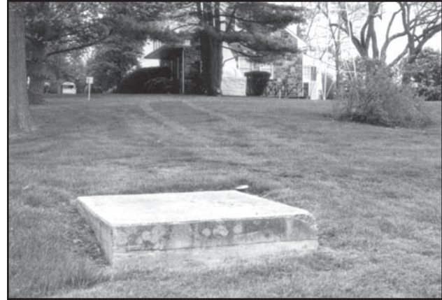
Figure 4.2. Detail of concrete pad where south guardhouse had been on Farm #1. (Photo by OCLP, 2002)
