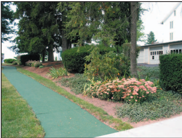
Figure 4.5. Detail of asphalt path north of house, (Photo by OCLP, 2005)
