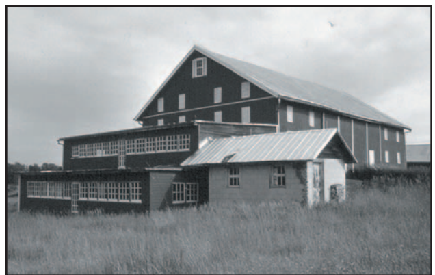
Figure 4.28. View looking northwest at the Bank Barn. (Photo by OCLP, 2002)
