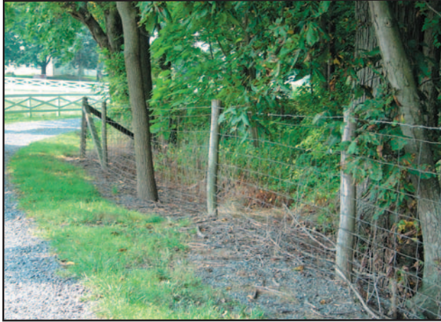
Figure 4.17. Detail of new (replacement-in-kind) post and wire fencing installed between Farm #1 and Farm #2. (Photo by Carol Hegeman)
