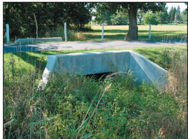
Figure 2.99. The box culvert along Nevins Lane would be an appropriate solution along the path between Farms #1 and #2. (Photo by OCLP, 2005)
