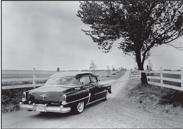
Figure 1.13. Wooden fence at entry gate, looking south, 1 August 1954. (US Navy, EISE NHS files, #2928)
