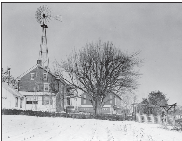
Figure 1.9. Allen Redding farmhouse from south, ca. 1952. (Lane Studio, EISE NHS files, #2874)
