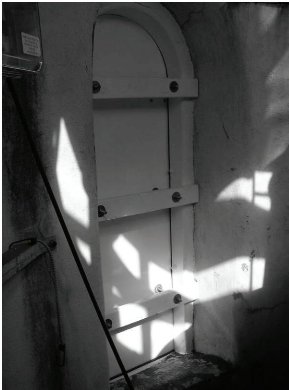
Figure 60. The original arched iron door has been recently removed and replaced with a plywood insert.
