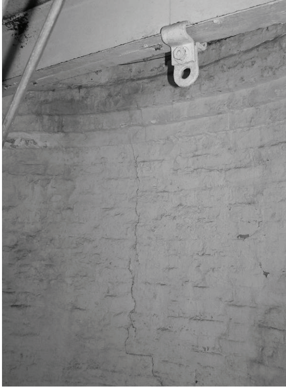
Figure 57. Vertical crack extending down from Watch Room level floor plate.
