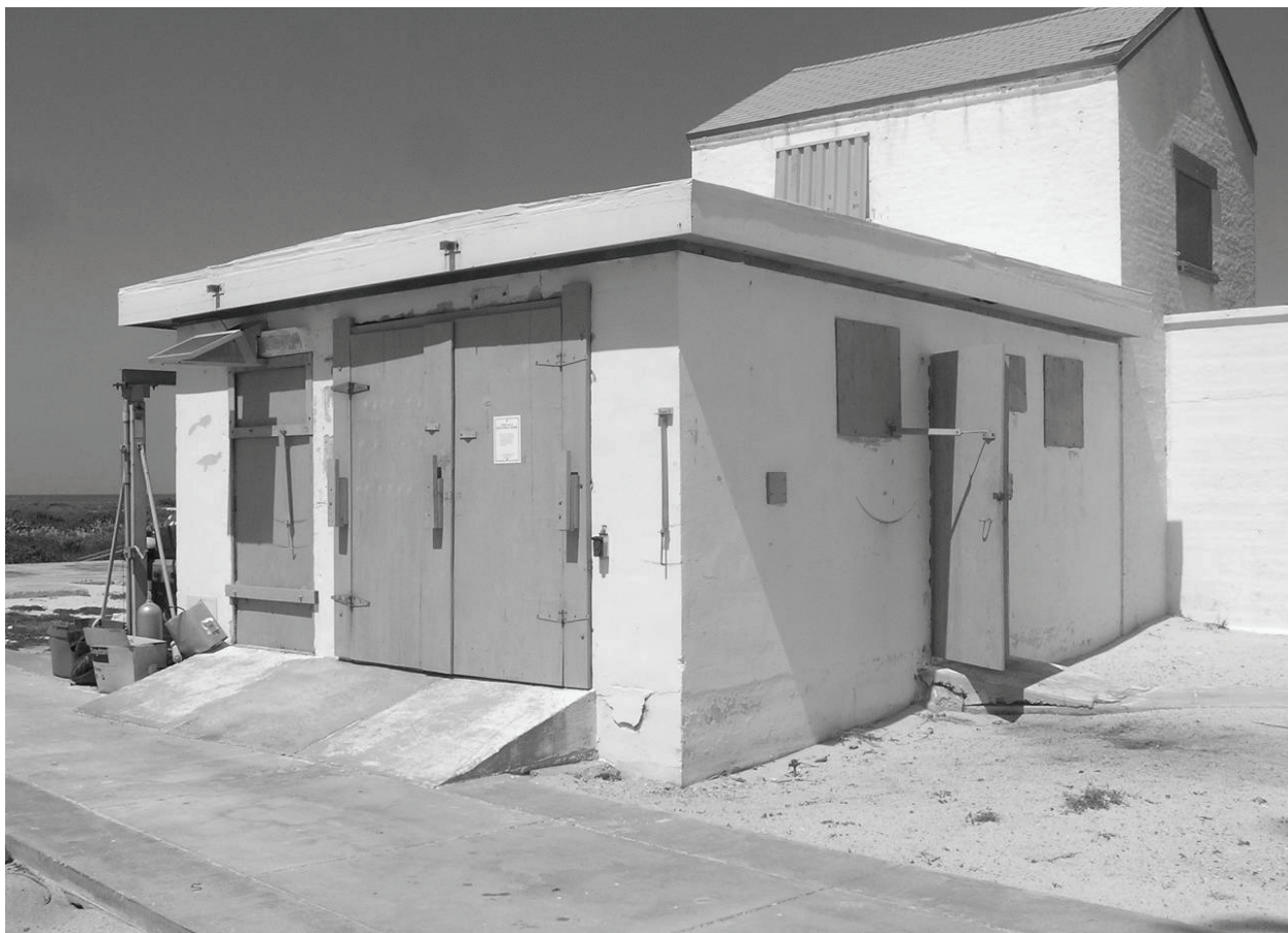
Figure 85. Concrete block addition constructed in 1982 by the crew of the USCG vessel White Sumac . When originally constructed the addition did not have any openings.
