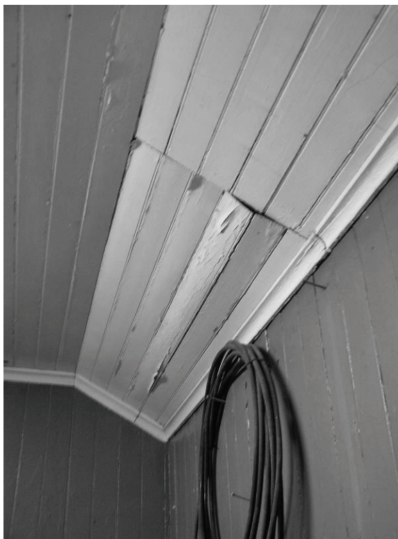
Figure 72. Image showing interruption of second floor ceiling finishes in the southeast corner of the room where the chimney for the fireplace would have penetrated the roof.
