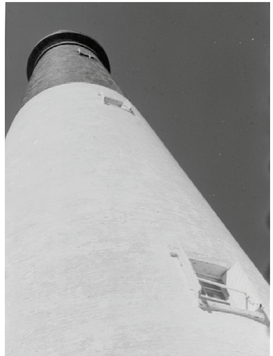
Figure 91. Pre-1967 image showing four-over-four, double hung windows with shutters.
