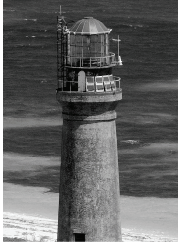
Figure 46. 2009 image of Lantern following repairs (Photo Courtesy of Enola Contracting Services Inc.).
