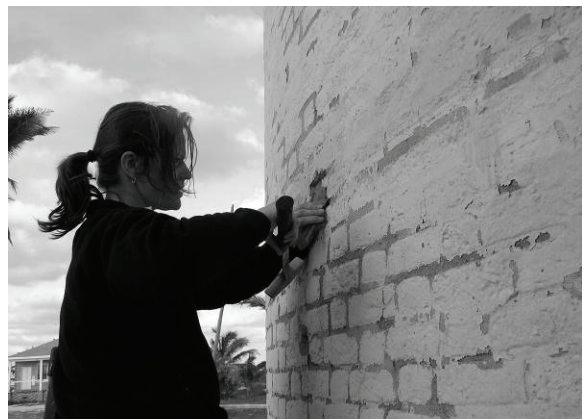
Figure 35. Dorothy Krotzer of Building Conservation Associates Inc. (BCA) works to remove a sample of the original mortar from the base of the Lighthouse.
