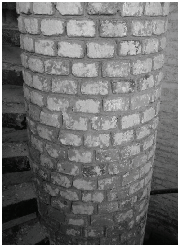
Figure 53. Hollow masonry "newel" at center of stair tower.
