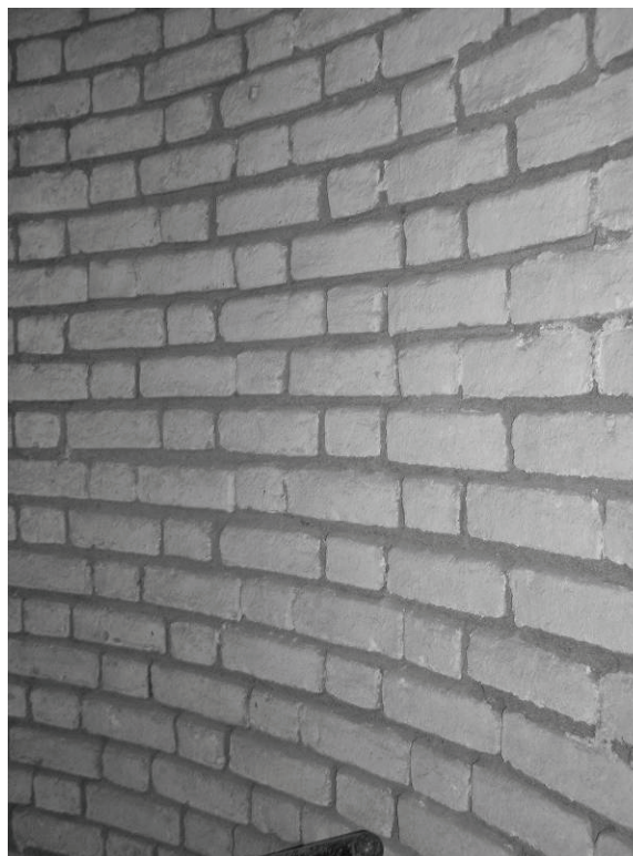
Figure 55. Typical view of interior wall surface showing deterioration of mortar. Note the paint is adhering well to the brick but has failed at the mortar joints.
