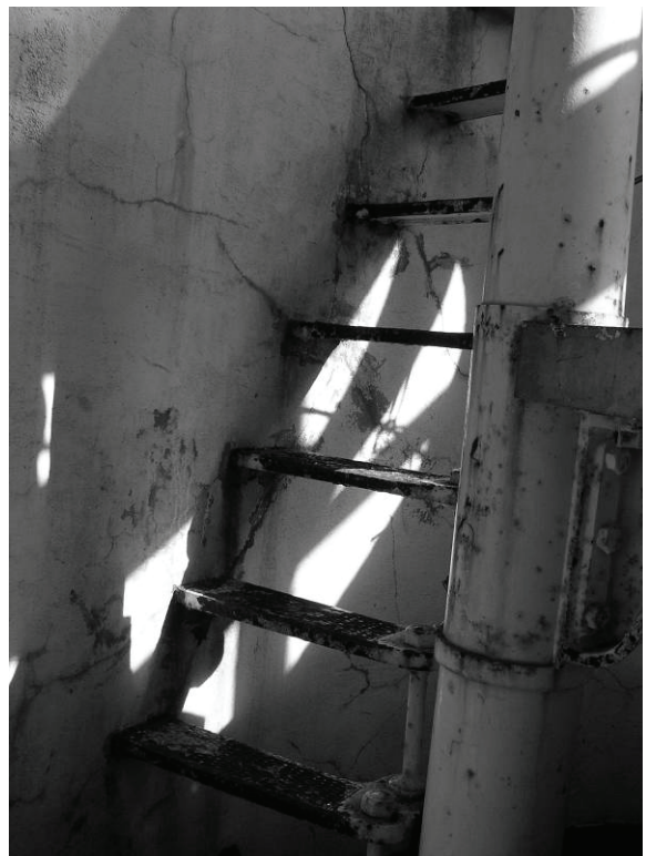
Figure 62. Iron stair between Watch Room and Lantern.
