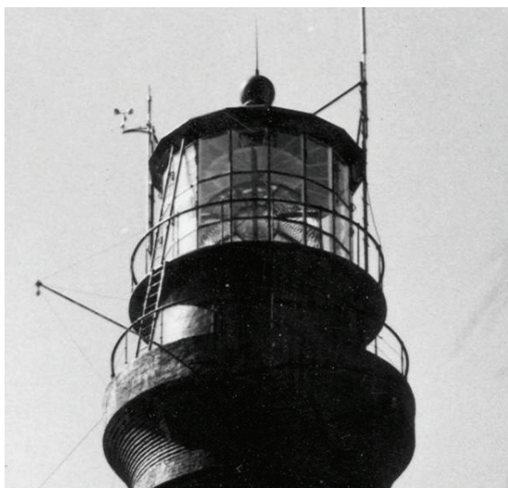
Figure 50. Undated image of the Lantern showing the second order bivalve lens in place. Note also the original ladder and pipe railings on the Lantern and Watch Room-level galleries.
