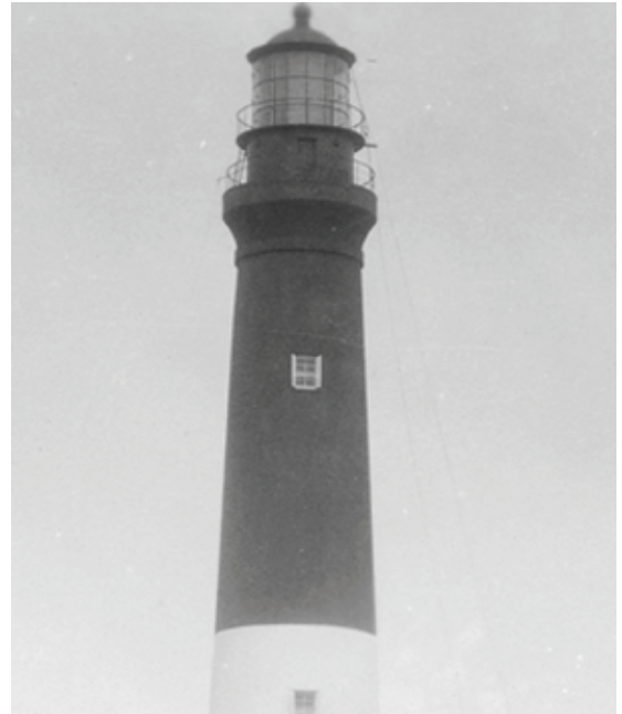
Figure 90. Undated view of the Lighthouse showing four-over-four double-hung windows and wood shutters.
