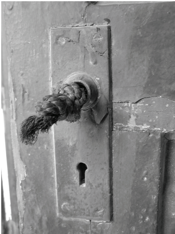
Figure 44. This escutcheon plate and the mortise lockset are the only remaining hardware components.
