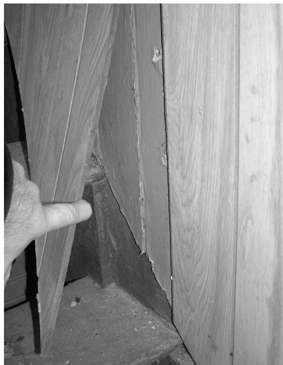
Figure 78. Image showing bead board wall finishes below wood paneling.
