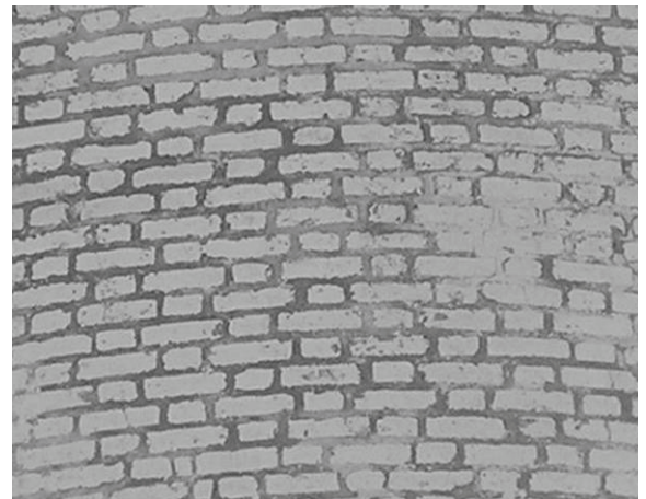
Figure 38. Close-up view of paint deterioration on exterior wall.
