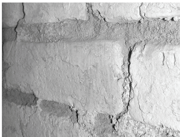
Figure 54. Close-up view of deteriorated mortar joints of stair tower walls. Almost universally the surface of the mortar has become friable, falling from the wall as powder.
