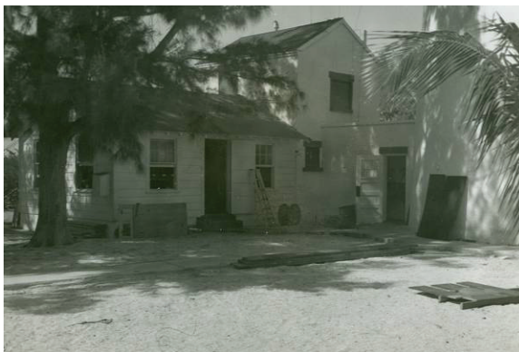
Figure 28. Image of wood-frame addition to Oil House constructed between 1943 and 1951.
