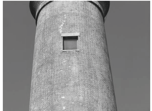
Figure 37. Vertical crack extending from head of fifth-level window.
