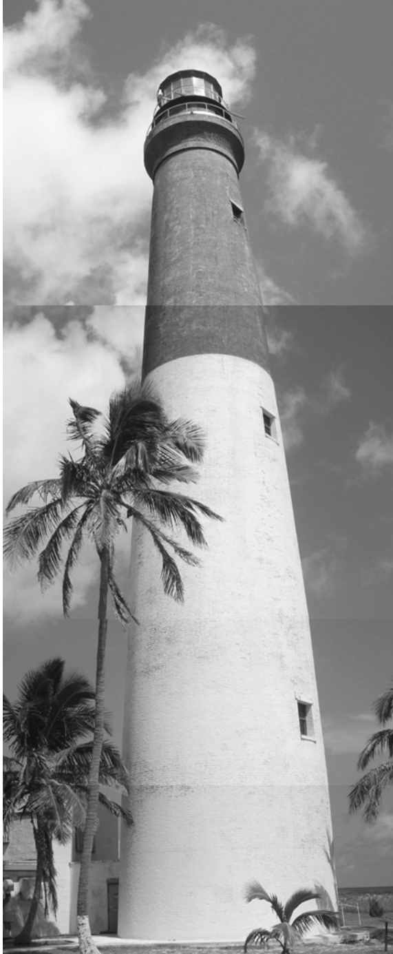
Figure 36. 2008 view of Lighthouse looking north. The painted finish of the tower is showing signs of weathering and deterioration. There is no discernable pattern to the paint loss.
