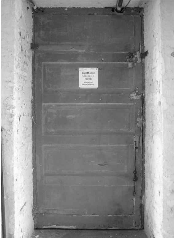
Figure 43. Five-panel wood entry door to tower.
