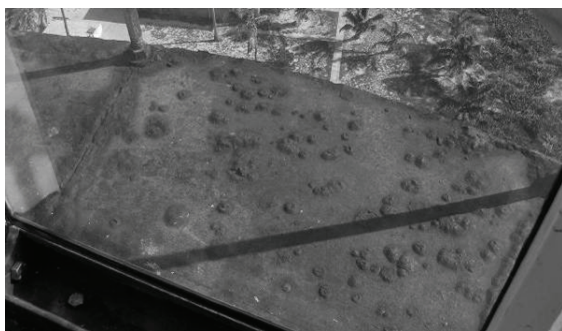
Figure 49. Image showing pitting corrosion on Lantern gallery floor plates.
