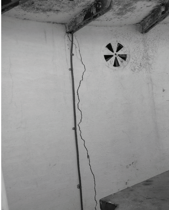
Figure 59. Vertical crack in watch room wall extending down from Lantern level floor plate.
