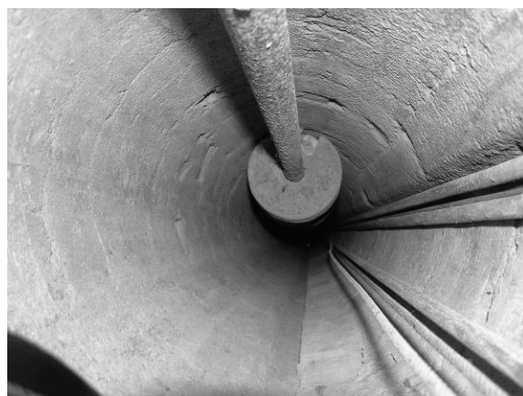
Figure 56. The hollow shaft within the central masonry newel accommodated weights that drove various components of the lamp and lens apparatus.
