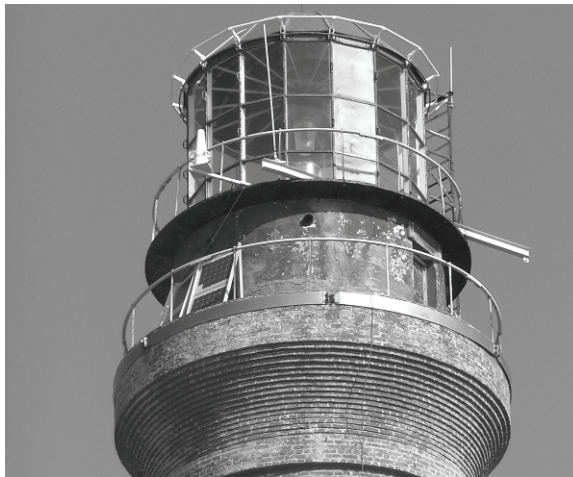
Figure 33. View of Lighthouse Lantern and corbelled masonry supporting the Watch Room gallery.
