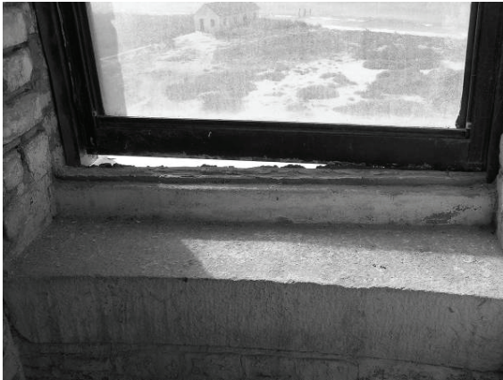
Figure 42. A concrete sill has been formed on top of the original granite sill at each window location to accommodate the installation of the modern aluminum sash.
