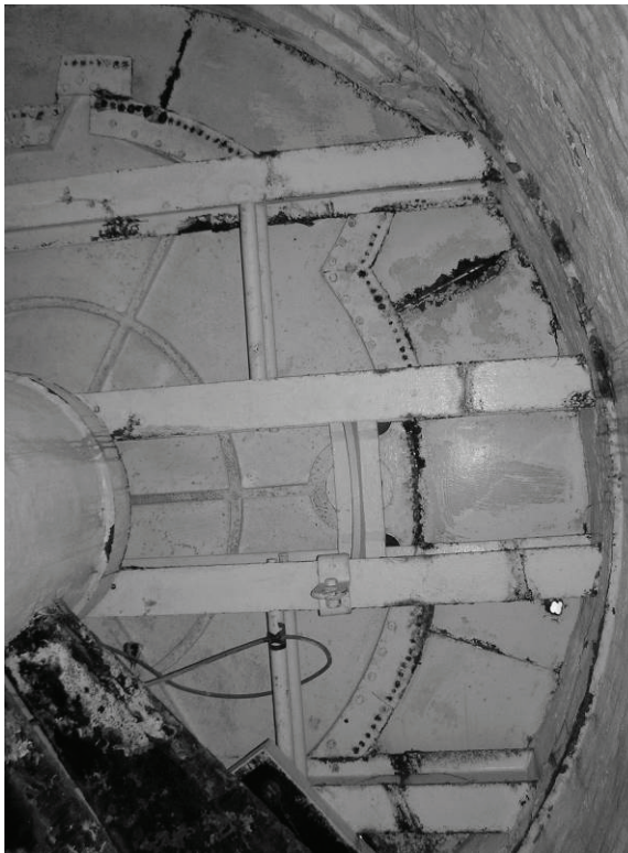
Figure 58. View looking up at the I-beams supporting the Watch Room level floor plate.
