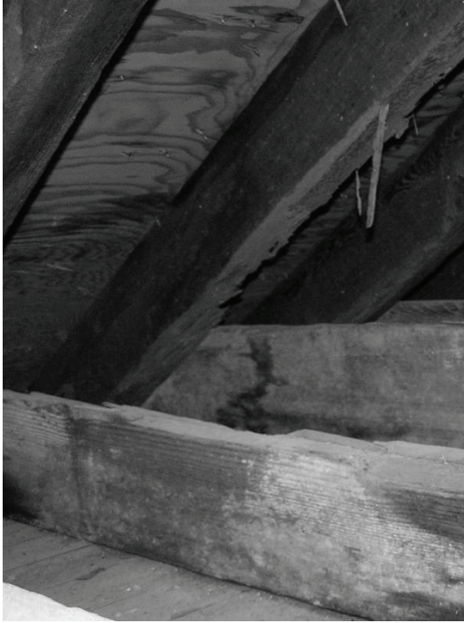
Figure 71. Image of roof framing members taken in attic of Oil House. Note evidence of moisture, minor termite damage and the different patina of the members.
