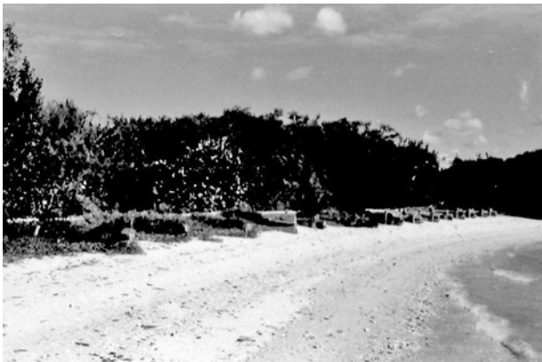
FIGURE 56. Log groins in place to control beach erosion, January 1959. (DESO Files)
