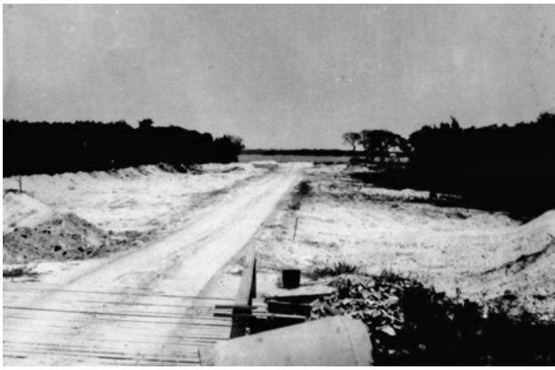
FIGURE 55. Dike completed at edge of mangrove in preparation for pumping hydraulic fill, June 1950. (DESO Files)
