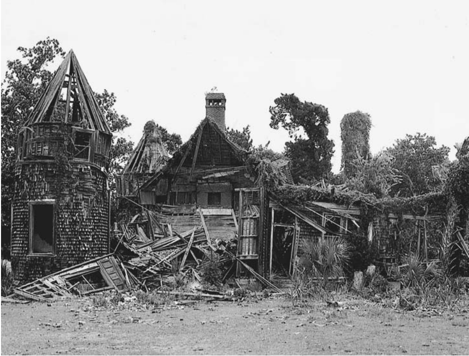
Fig. 6.3. During the 1980s and 1990s the magnificent Recreation House collapsed due to weather and termite damage.
