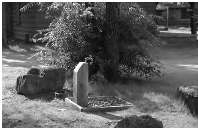
Figure 9-1. Existing hydrant type with stone drainage area at base in Cold Springs Campground.
