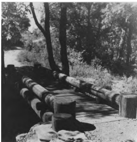
Figure 9-23. Historic bridge design, unknown location in park, circa 1935. Bridges were constructed of large, peeled, creosote-impregnated logs, atop stone abutments.
