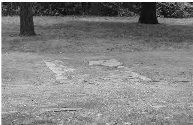
Figure 9-31. Drainage crossing at Flower Park, 2002. These will be redone as part of the trail reconstruction project in 2003 and 2004.
