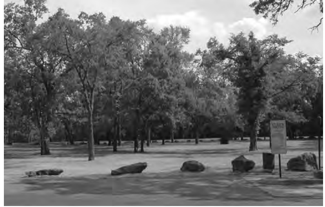
Figure 9-16. Boulder roadside barrier. Notice that recently installed boulders are placed at grade, and not embedded in the soil.
