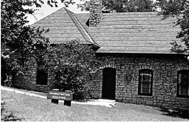
Figure 5-39. Administration Building (Leeper House), circa 1960.
