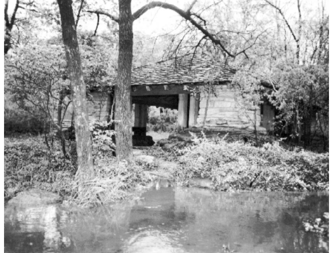
Figure 5-44. Pavilion Springs after the 1953 flood.
