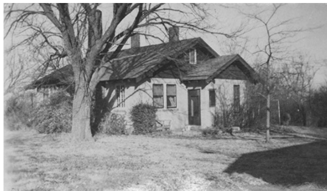
Figure 5-36. Residence #4, today's Building #2, circa 1950.
