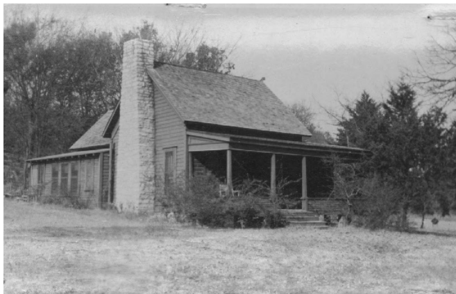
Figure 5-33. Residence #3, near Panther Falls, circa 1950. This building was removed sometime prior to 1969.
