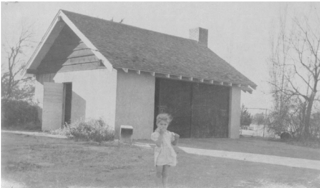
Figure 5-30. Front of the garage and laundry building, 1950.
