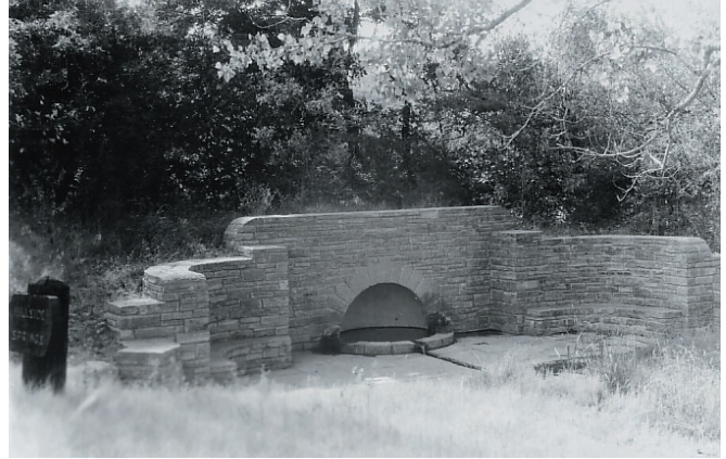
Figure 5-40. Hillside Springs, circa 1950. Note half-log sign at entrance.
