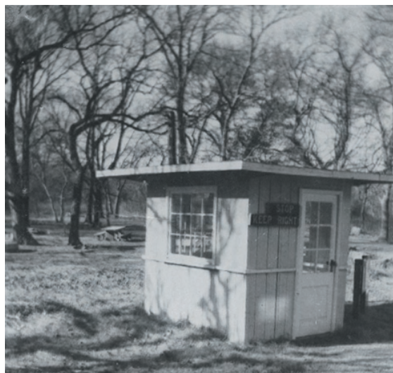
Figure 5-67. Checking Station at Rock Creek Campground, 1954.
