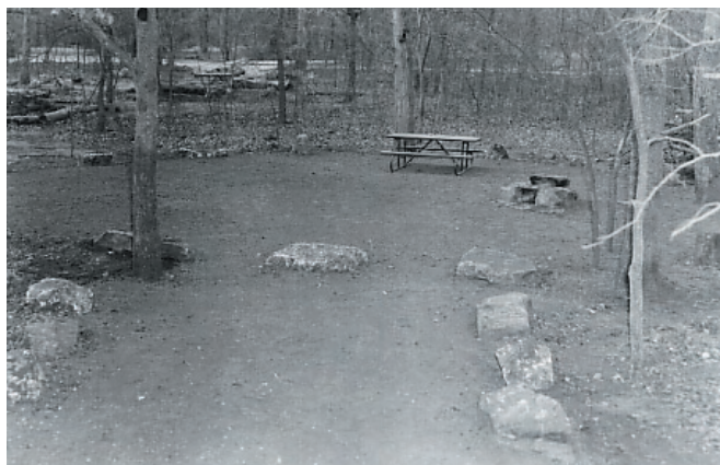
Figure 5-49. Finished repairs at Cold Springs Campground, 1963.
