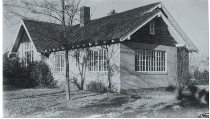
Figure 5-29. Rear of Superintendent's Residence, 1950.
