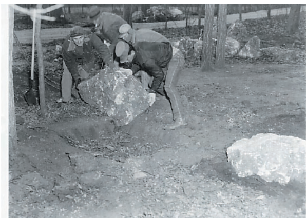
Figure 5-50. Campsite reorganization at Cold Springs Campground, 1963. Note how boulders are being embedded below grade.
