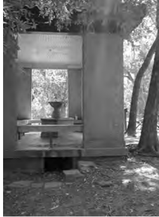
Figure 11-35. Comparison of original elevation and current conditions. Note five jets in original drawing and extant crawl space under pavilion.
