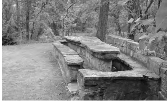
Figure 11-99. Elements at the large picnic area, such as the flaking table top, seats, and walls shown here, should be repaired with new flagstone, using historic masonry techniques.
