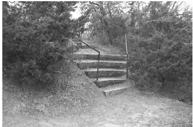
Figure 11-25. Existing concrete steps at the Bromide Hill overlook are inaccessible, and small overlook structure should be added up the trail to provide access to the view.
