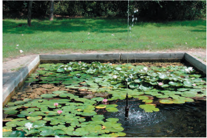
Figure 11-14. Lily pond with jet, existing conditions. Pool should be repaired and grass joints should be replaced on flagstone coping.
