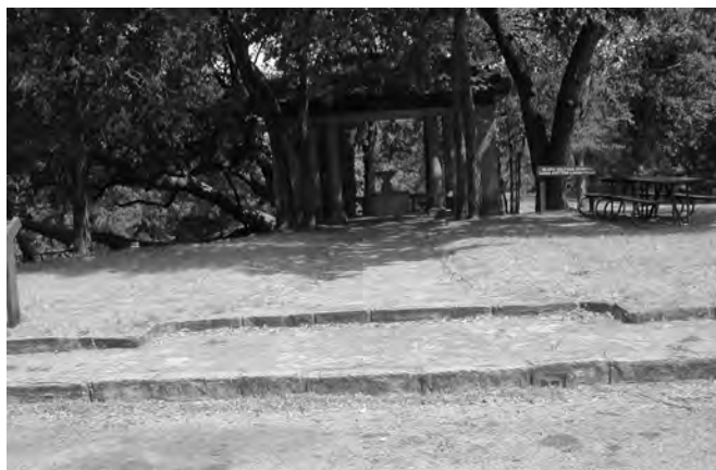
Figure 11-41. Two low curbs at the entry to the pavilion are barriers to ADA accessibility. While the lower curb can be easily surmounted by constructing a ramp at the north end of the parking area, the second curb is still a barrier. A long-term solution of ramping between the second curb and the grade of the pavilion is proposed.
