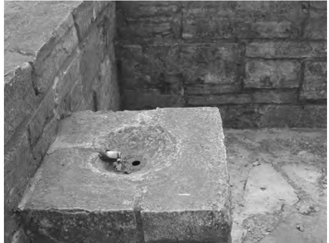
Figure 11-19. Detail of drinking fountain to be replaced at the 12th Street Fountain. New plumbing and fixtures will be required.
