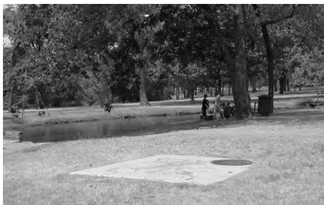
Figure 11-53. Large concrete siphon covers and manholes without regular maintenance needs could be placed below grade, but only when infrastructure is replaced in the future.
