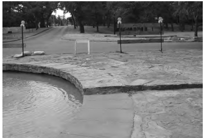
Figure 11-20. Concrete coping along southern half of pool edge should be replaced with flagstone to match the other half. Flagstone terrace should be maintained by sweeping and weed removal.
