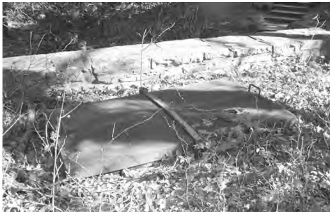
Figure 11-74. Lid on the spring container is rusted, and should be replaced.
