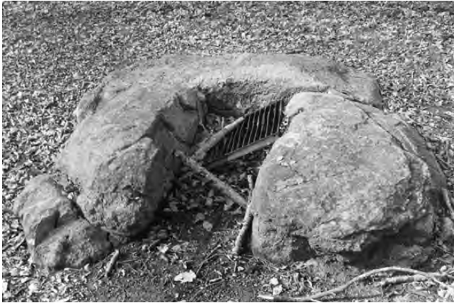
Figure 11-27. Second of four firepits to be repaired. This structure may not support firebrick interior.
