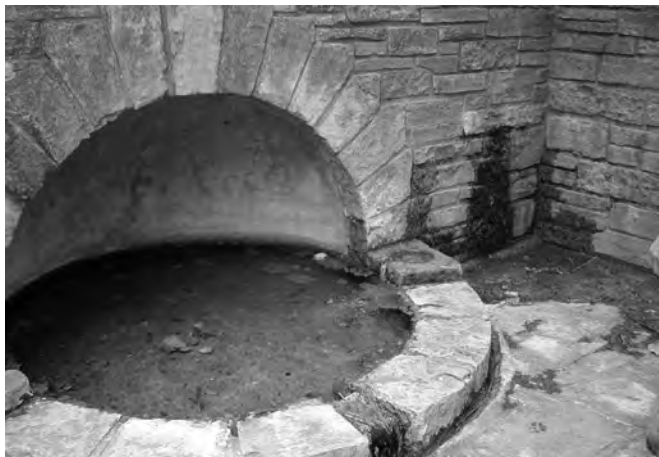
Figure 11-73. In addition to cleaning the pool, the lack of flow from the spring's bubblers should be investigated, and pipes leading to them cleaned or replaced. Note seepage from spring through wall to the right.
