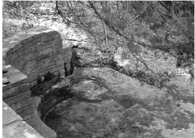
Figure 11-72. Algae covers not only pools, but masonry. Regularly scheduled cleaning, plus increasing the sun in the area should help make the area less damp and more pleasant.
