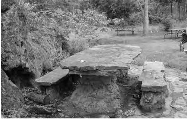
Figure 11-100. Table at the “End of the World” should be repointed and its cracked bench repaired.
