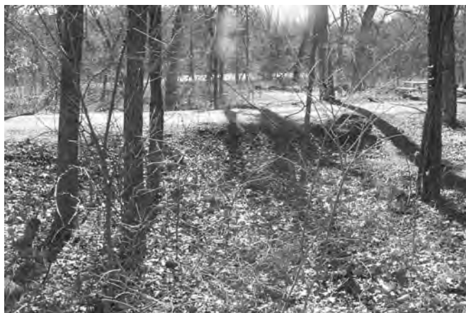
Figure 11-92. Clogged culvert in campground is just one issue contributing to poor drainage in Cold Springs Campground. Culvert should be cleared.
