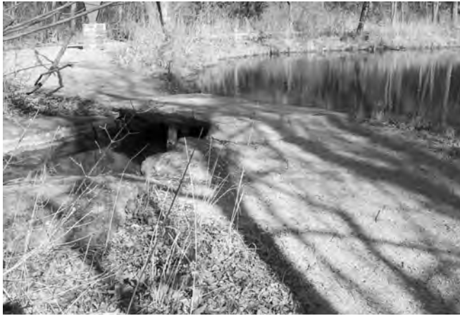
Figure 11-111. Stone bridge at lowermost crossing should be reset and made level. A fully ADA-accessible bridge in this location is not recommended.
