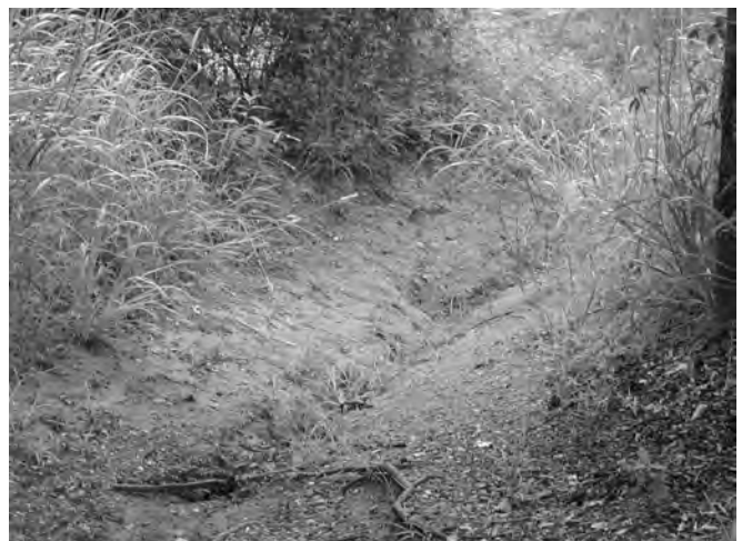
Figure 11-5. Eroded path near causeway steps should be revegetated and protected with temporary fencing.
