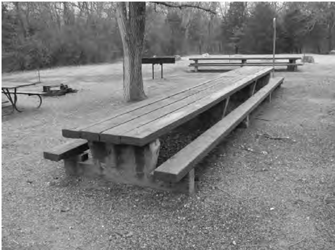
Figure 11-97. Large picnic tables in Cold Springs need repairs to wooden planking and concrete bases.
