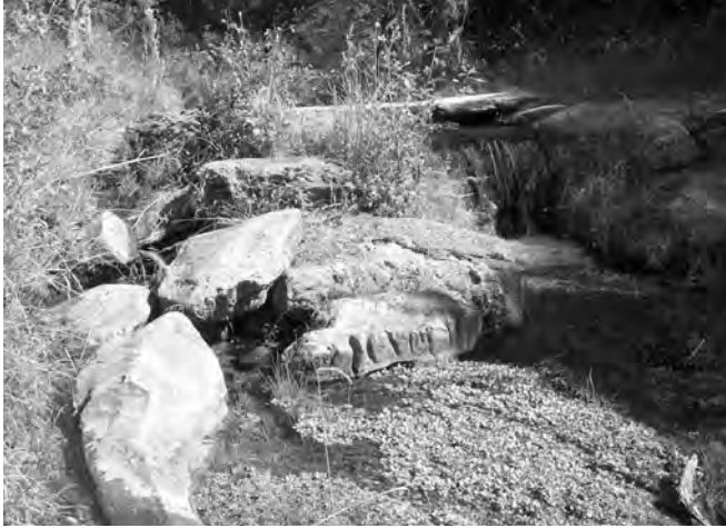
Figure 11-110. Lost tree at the uppermost dam at Antelope Springs has caused minor breach; this should be repaired.
