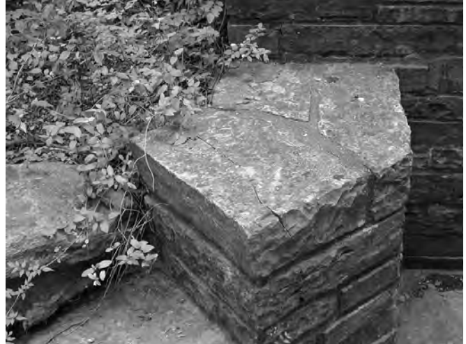
Figure 11-76. Stone at entry wall is cracked and should be repaired before it is lost or further damaged. Masonry throughout the district should be annually inspected for these types of issues.
