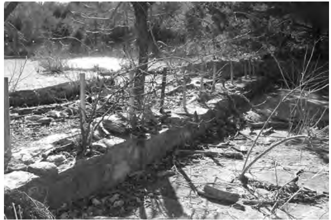
Figure 11-58. The Buffalo Pasture dam is spalling, cracking and being undercut. Masonry repairs are needed.
