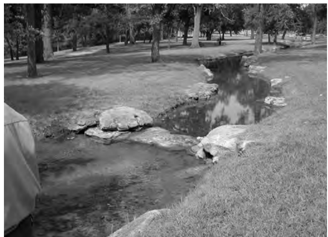
Figure 11-45. Stream and pool edges are being undercut in some locations and should be stabilized as needed. Edges should be carefully reinstated to match historic conditions (Figure 10-44).
