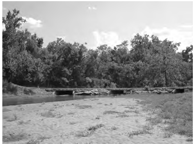
Figure 11-39. Undercutting of bridge occurs due to silt and sand build up and blockage of western waterway under causeway. Removal of sand will improve these conditions and help reinstate former favorite swimming beach.
