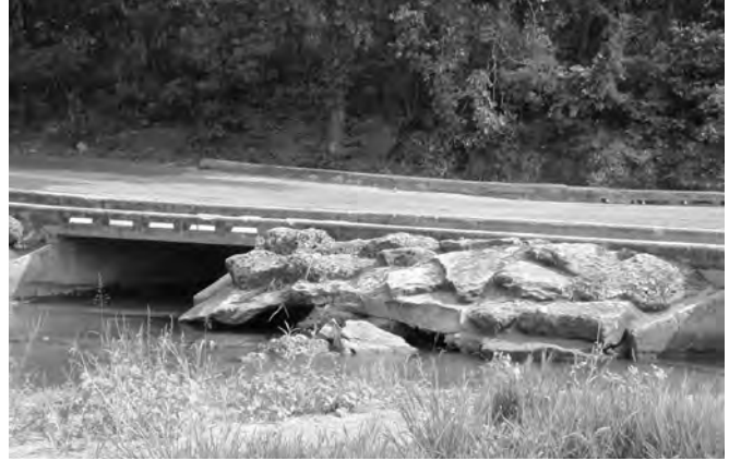
Figure 11-38. Dark areas at base of stones indicate places where stream is undercutting causeway. Masonry repair is required.
