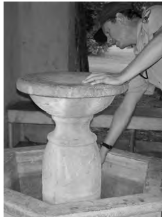
Figure 11-36. Comparison of original fountain elevation and current conditions. Note filled basin and lack of fountain jets.
