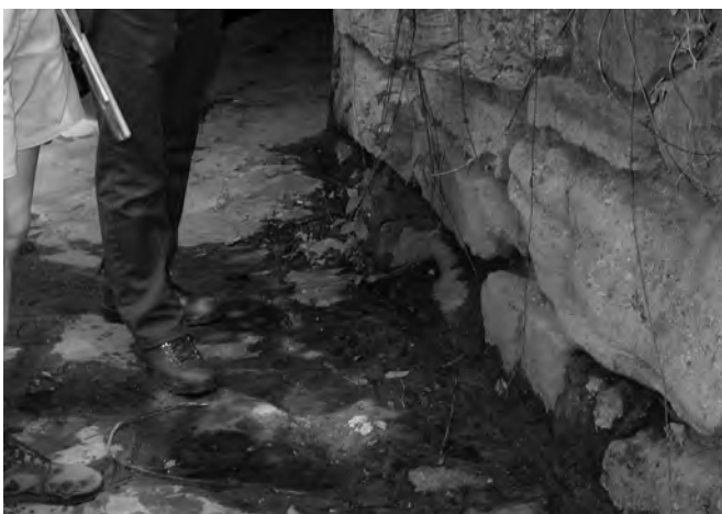
Figure 11-71. Seepage from springs behind underpass wall should be redirected via minor masonry repairs.
