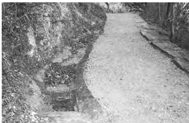
Figure 11-23. Clogged gutter and drain on Bromide Hill. Adding grates over the inlets may help reduce erosion and the need for periodic trail resurfacing.
