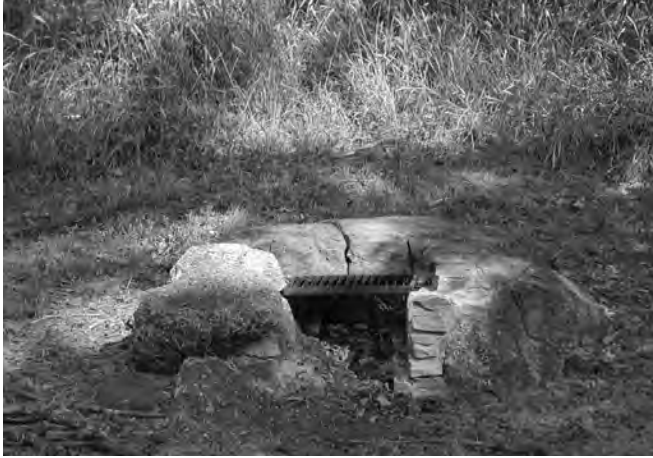
Figure 11-26. One of four firepits to be preserved at Walnut Grove. Obtrusive fire brick should be removed, and replaced. Grills should be repaired or replaced and chained or cabled to structure.
