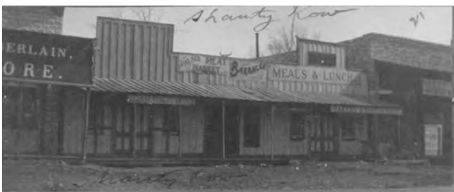
Figure 2-9. “Shanty Row,” circa 1901. Town buildings were constructed of wood, logs, or stone and were located in close proximity to one another. Joseph Swords Collection, courtesy of the Oklahoma Historical Society, negative 2153.25.
