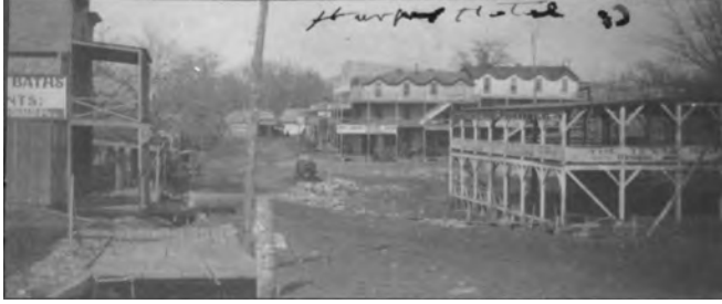
Figure 2-7. View of Sulphur Springs, looking north down Main Street toward the Harper Hotel (in the center distance), circa 1900. The first pavilion over the springs is the white, two-story framed building on the right. Joseph Swords Collection, courtesy of the Oklahoma Historical Society, negative 2153.39.
