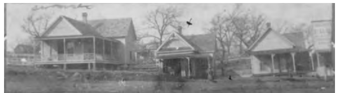
Figure 2-10. Three residential houses just outside of Sulphur Springs’ central “business district.” Note the larger lots and frame houses, as well as the large deciduous trees, probably oaks, behind the structures. Joseph Swords Collection, courtesy of the Oklahoma Historical Society, negative 2153.22.
