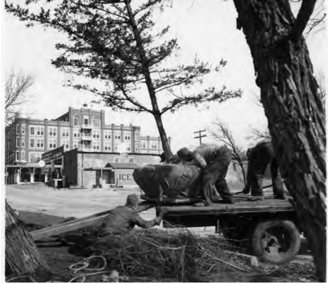
Figure 10-7. Red cedar being set at main entrance circa 1935.
