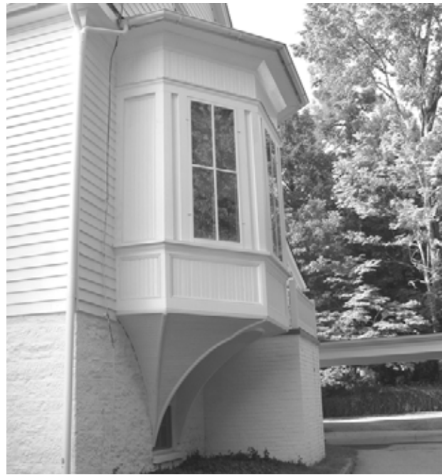
FIGURE 128. View of west bay window.(T. Jones, NPS-SERO-CR, 2004)
