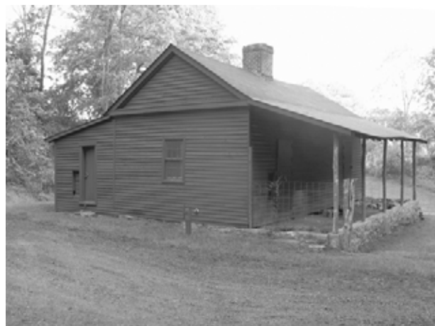
FIGURE 8. The so-called Buck House, probably built in the second quarter of the nineteenth century as an overseer's house. (T. Jones, NPS-SERO-CR, 2004)
