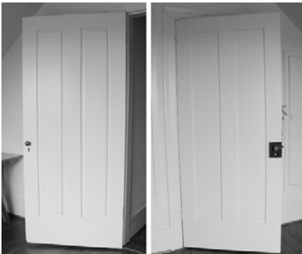
FIGURE 195. View of door at Crow’s Nest (207), typical of original bedroom doors on the second floor. (T. Jones, NPS-SERO-CR, 2004)
