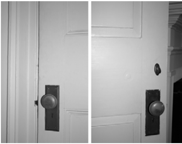
FIGURE 161. Both faces of D-36, presumed to be typical of original first-floor doors, but with hardware installed in 1924. (T. Jones,
