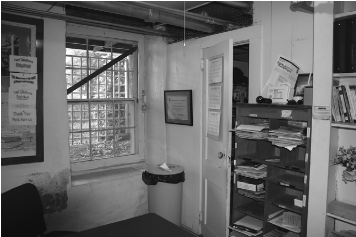
FIGURE 150. View southeast in Room 004. (T. Jones, NPS-SERO-CR, 2004)
