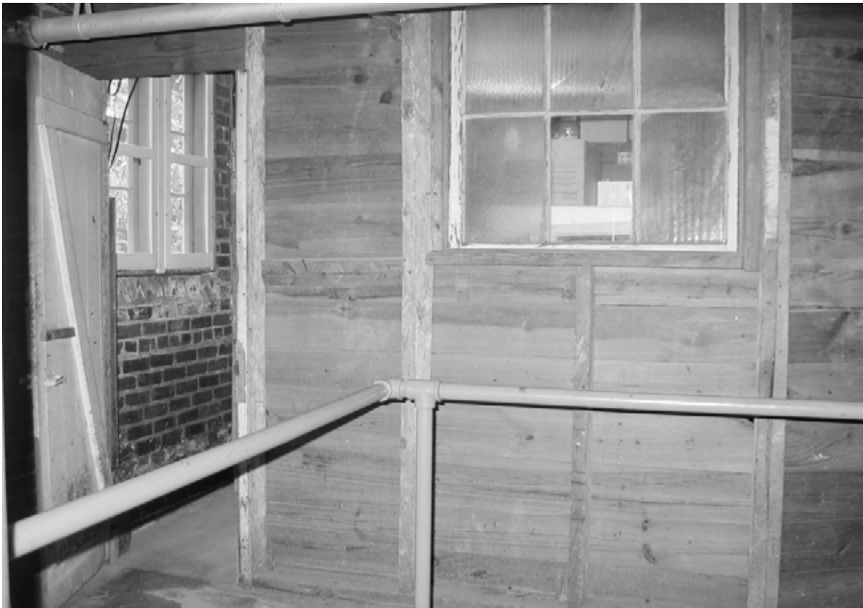
FIGURE 157. View southwest into Room 012. Window sash was probably salvaged by the Sandburgs when they demolished Smyth’s master bathroom where the west Porch is now located (T. Jones, NPS-SERO-CR, 2004)
