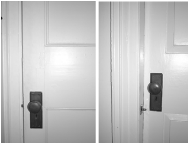
FIGURE 162. Both faces of D-48, antebellum but with slightly different panel molding (T. Jones, NPS-SERO-CR, 2004)
