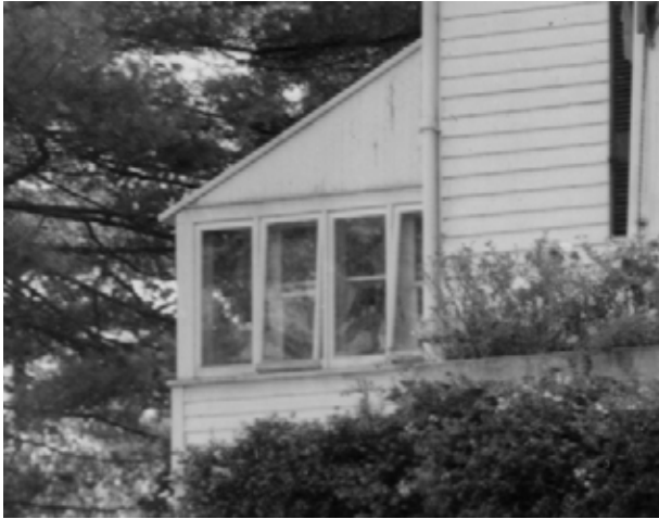
FIGURE 80. Detail of view of Connemara in 1938, showing Conservatory constructed by Smyth on east side of Front Room. (CARL3001/01/45P)
