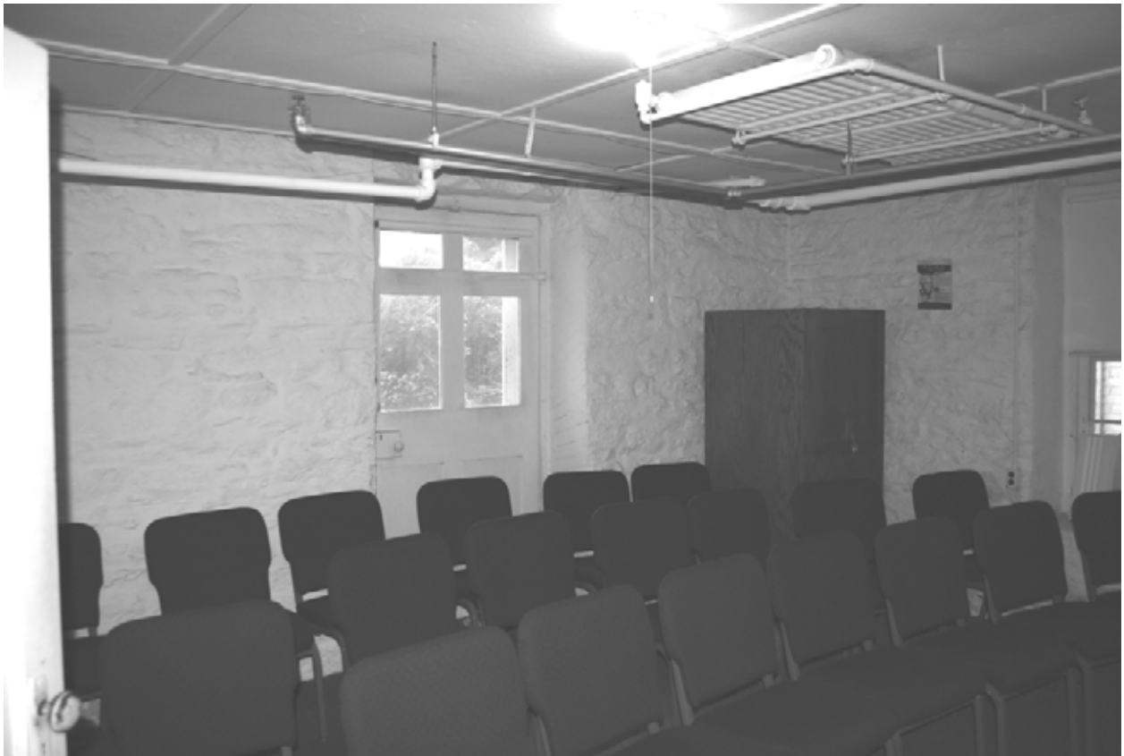
FIGURE 149. View northeast in Room 002. (T. Jones, NPS-SERO-CR, 2004)
