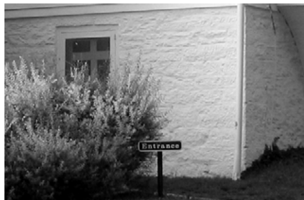
FIGURE 109. View of foundation at northwest corner of original house. (T. Jones, NPS-SERO-CR, 2004)
