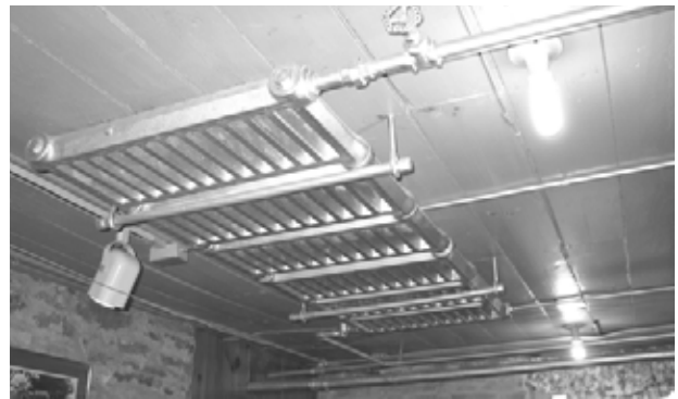
FIGURE 146. View of typical ceiling-hung radiator. (T. Jones, NPS-SERO-CR, 2004)
