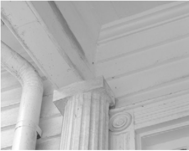
FIGURE 131. View of typical Portico details. (T. Jones, NPS-SERO-CR, 2004)
