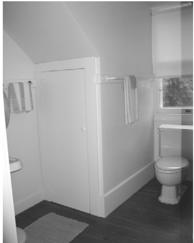
FIGURE 211. View southeast in Room 217. (T. Jones, NPS-SERO-CR, 2004)
