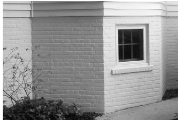
FIGURE 108. View of foundation at east end of 1920s rear addition. (T. Jones, NPS-SERO-CR, 2004)
