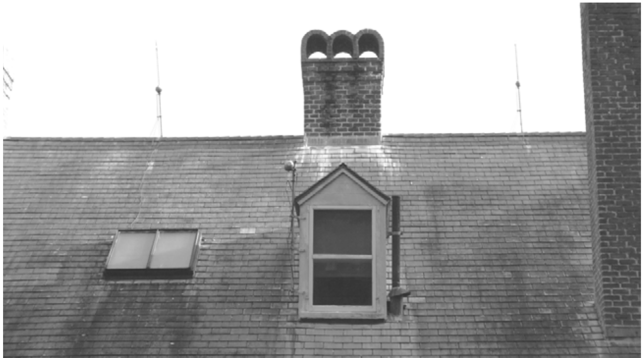
FIGURE 117. View of rear (south) shed of main roof, showing skylight, lightning rods, and typical dormer. (T. Jones, NPS-SERO-CR, 2004)
