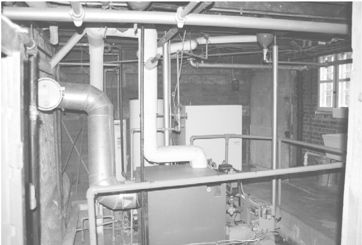
FIGURE 156. View to east in Room 011. (T. Jones, NPS-SERO-CR, 2004)
