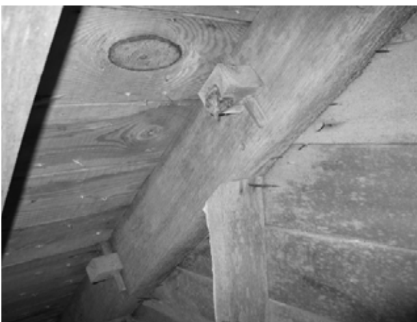
FIGURE 116. View of end rafter at west side of main roof, showing lookouts mortised and pegged in place. (T. Jones, NPS-SERO-CR, 2004)
