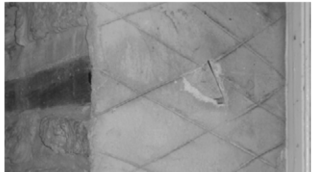
FIGURE 145. View of west jamb of Door D-1. Left of center is part of the wooden nailer inset into the masonry. (T. Jones, NPS-SERO-CR, 2004)
