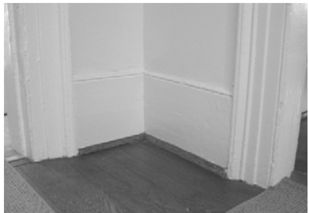
FIGURE 165. View of baseboard and casing at southwest corner of Hall (115). Casing at right is assumed to be original (1838) while casing at left dates to Memminger's remodeling in 1848. (T. Jones, NPS-SERO-CR, 2004)
