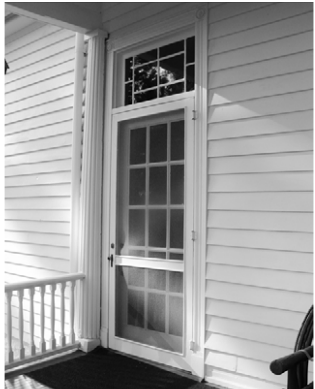
FIGURE 125. View of Door D-11, with original casing, mid-19th century transom, and c. 1924 French door and screened door. (T. Jones, NPS-SERO-CR, 2004)
