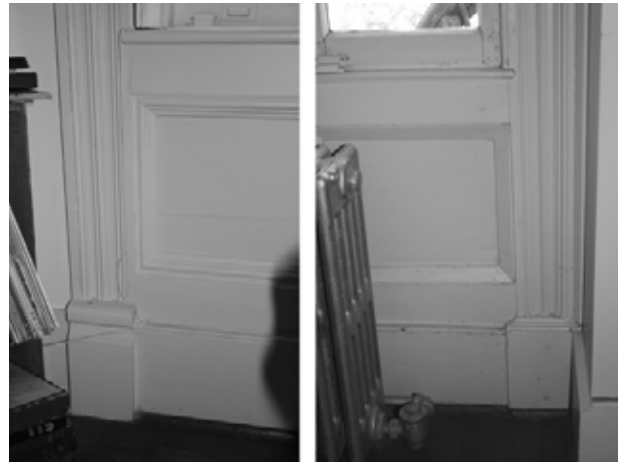
FIGURE 170. View of original window panels, right, and panels added c. 1890, left.(T. Jones, NPS-SERO-CR, 2004)
