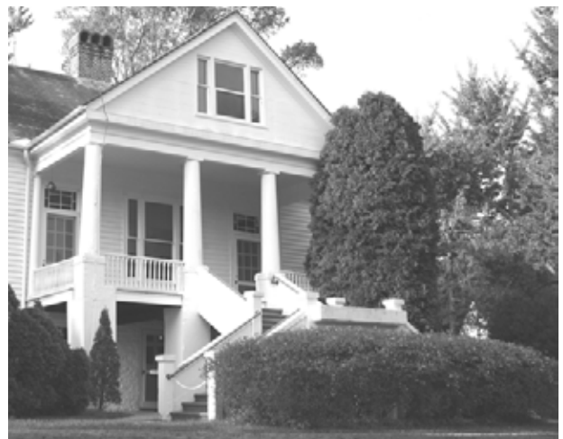
FIGURE 130. View of Portico.(T. Jones, NPS-SERO-CR, 2004)
