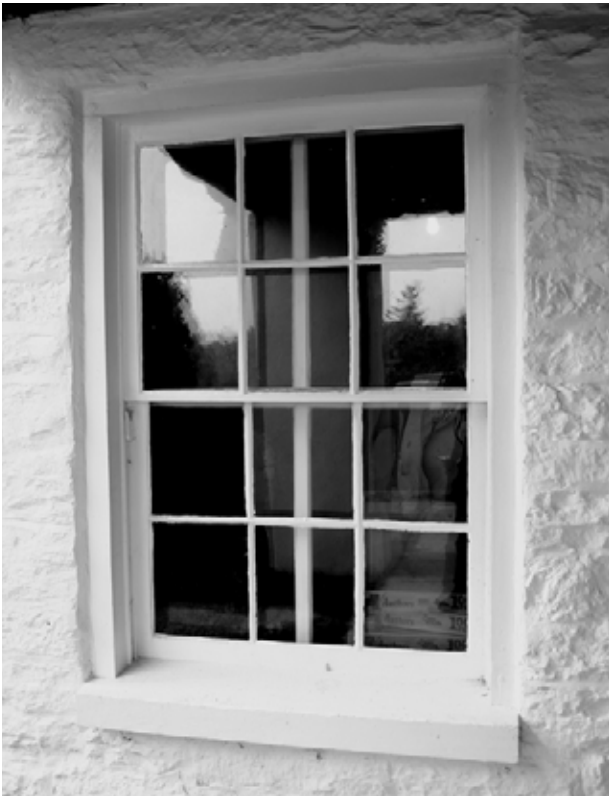
FIGURE 119. Window W-2, with original sash, in north wall of Room 001. Note wooden sash stop near upper left corner of lower sash. (T. Jones, NPS-SERO-CR, 2004)
