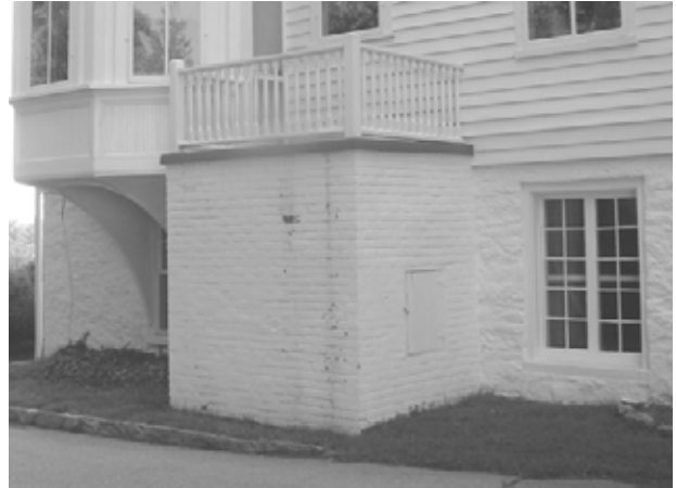
FIGURE 139. View of West Porch. (T. Jones, NPS-SERO-CR, 2004)
