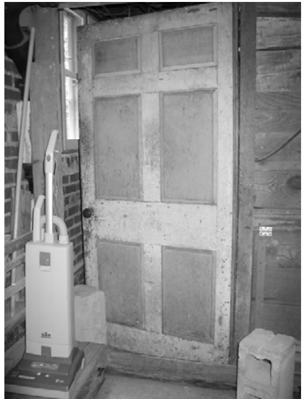
FIGURE 153. View of re-used antebellum door between Rooms 010 and 011. (T. Jones, NPS-SERO-CR, 2004)
