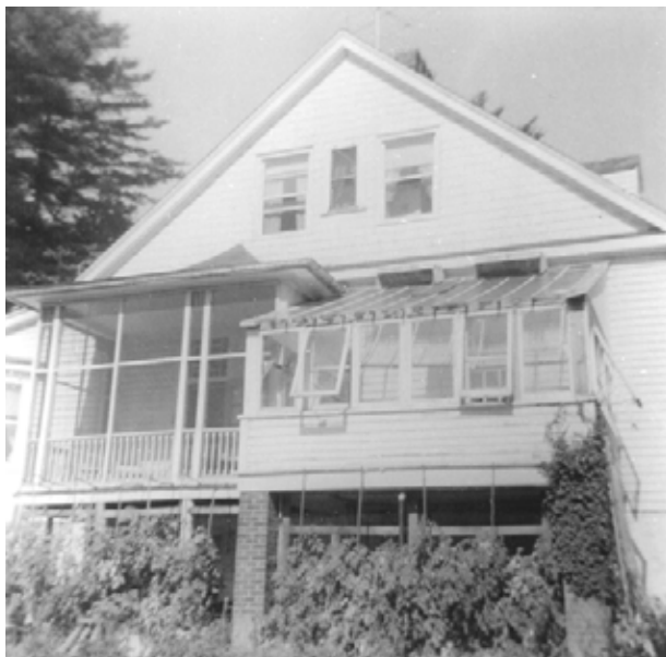
FIGURE 87. View of East Porch and Conservatory, showing window added in east gable for new bathroom on second floor. (CARL3000/15/28P)
