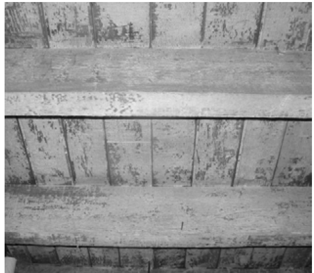
FIGURE 111. View of typical original first floor joists, as seen from Room 018. (T. Jones, NPS-SERO-CR, 2004)
