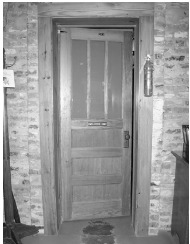
FIGURE 147. View of door from Room 001 into 005, typical of varnished fir doors installed by the Sandburgs around 1947. (T. Jones, NPS-SERO-CR, 2004)
