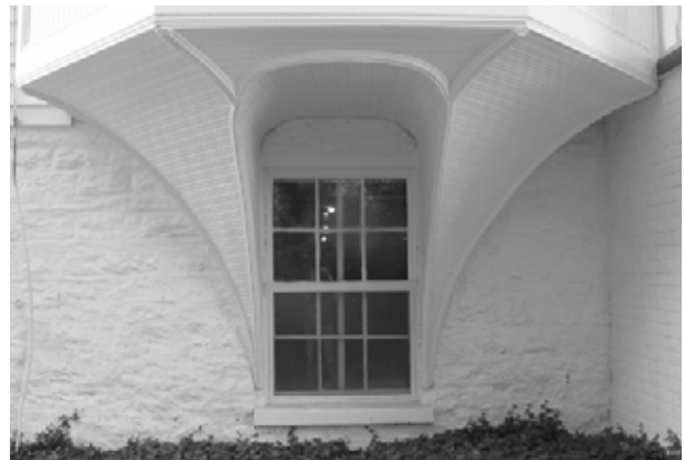
FIGURE 129. View of part of bay window on west side of house.(T. Jones, NPS-SERO-CR, 2004)
