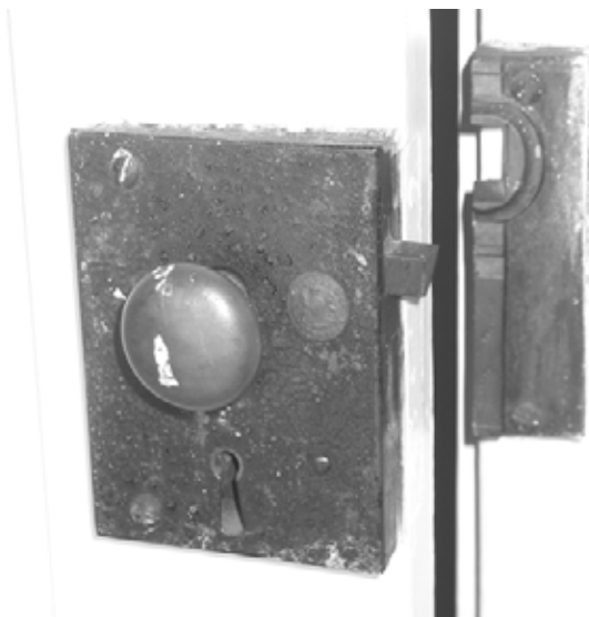
FIGURE 198. View of Carpenter & Co. rim lock, typical of original locks on second floor. (T. Jones, NPS-SERO-CR, 2004)
