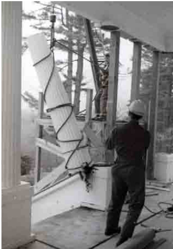
FIGURE 103. Removal of Front Porch columns in the spring of 1974. The only original column that remains intact is the one at left in this image.(CALO4008/01/048P)
