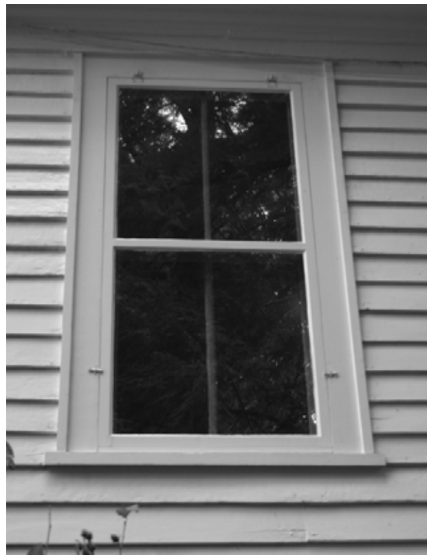
FIGURE 121. View of Window W-21, typical of rear addition (c. 1924), with two-over-two sash intact. A two-light, exterior storm sash is installed at the opening in this image. (T. Jones, NPS-SERO-CR, 2004)
