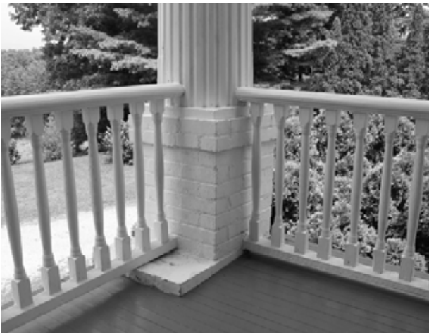
FIGURE 133. View of northeast corner of Portico showing typical balustrade (c. 1890) and brick pier (c. 1924). (T. Jones, NPS-SERO-CR, 2004)
