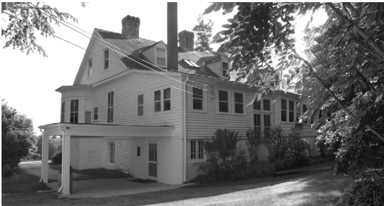
FIGURE 106. A view of the house from the southwest (T. Jones, NPS-SERO-CR, 2004)
