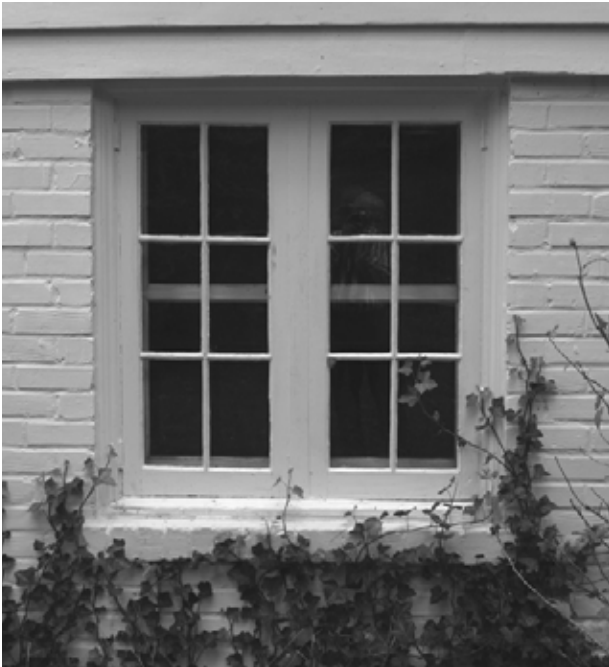
FIGURE 122. View of Window W-8, typical of ground floor windows in rear addition. (T. Jones, NPS-SERO-CR, 2004)
