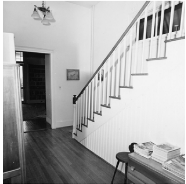
FIGURE 96. View of stair hall in 1967. (CARL4011/01-09, photograph by Cecil Stoughton)
