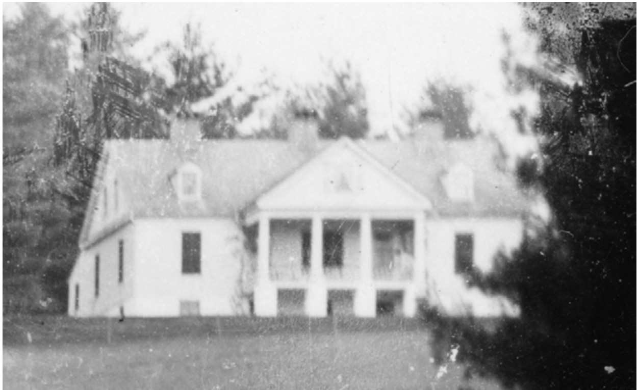
FIGURE 63. Detail from view of Rock Hill, taken prior to the late Victorian additions and alterations that were made around 1890, with Memminger’s antebellum addition partially visible at left. Note the absence of stairs to the front porch. (CARL3001/01/48P, photo by Baker Barber)
