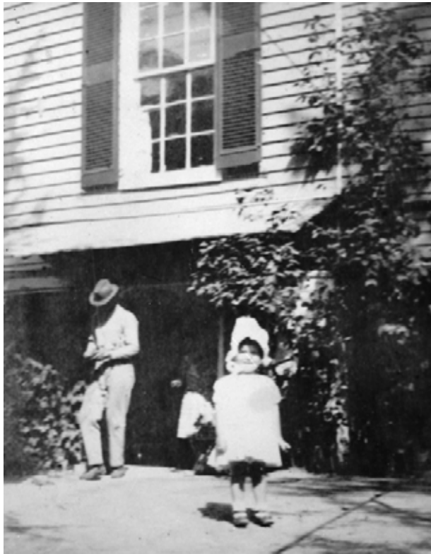
FIGURE 66. View at west end of Main House, showing window at west end of Memminger's addition, c. 1910. (CARL3001/01/30P)
