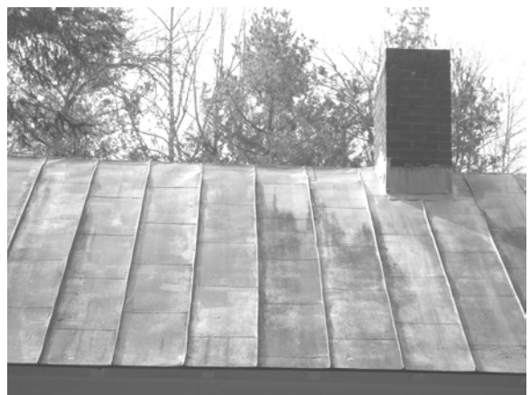
Figure C-8. Terne-coated metal roofing and stepped chimney flashing.
