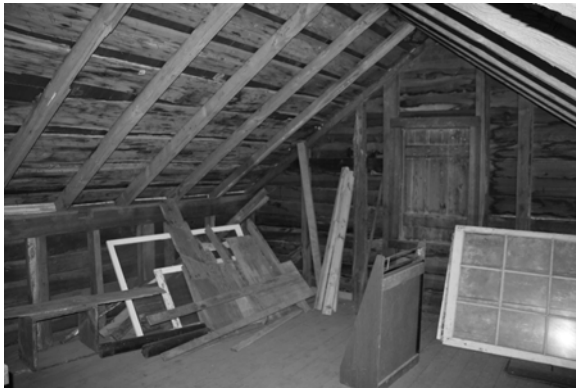
Figure C-55 Room 201A looking southeast
