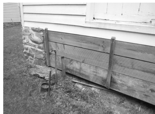
Figure C-65 Hose bib at west elevation
