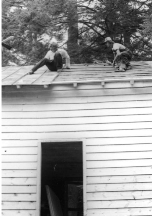
Figure B-15 Roof repairs in progress, May 1978 (CARL4008/05/46P)
