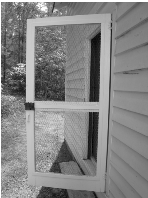
Figure C-16 Screen door at east elevation, south doorway
