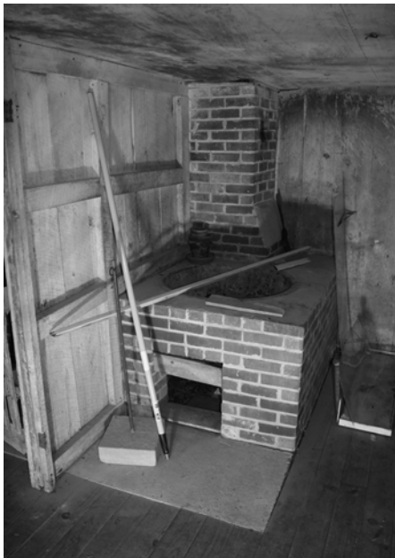
Figure C-40 Room 102A looking southeast.
