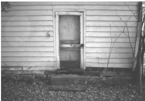
Figure B-7 North door on east elevation, Dec. 1973 (CARL4024/6/02)
