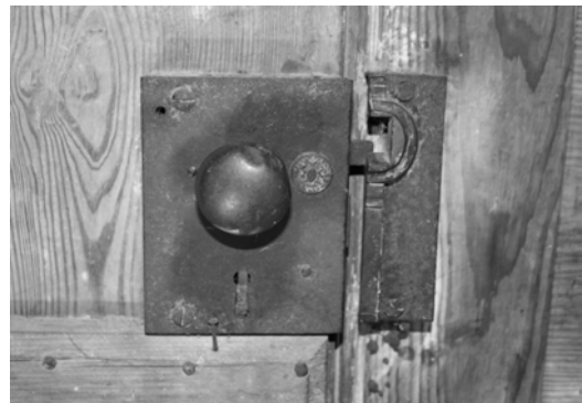
Figure C-12 Rim lock at east elevation, south doorway
