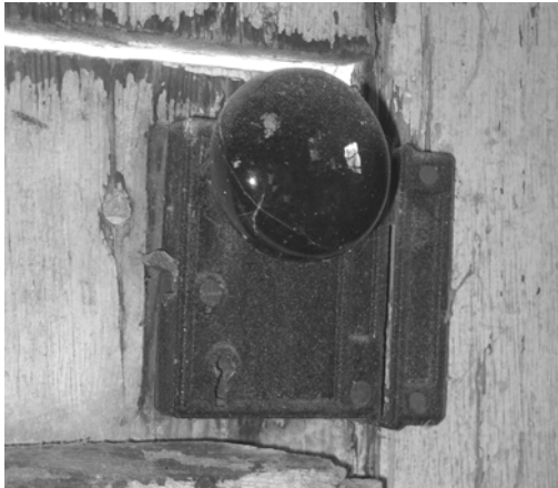
Figure C-14 Rim lock at west elevation, north doorway
