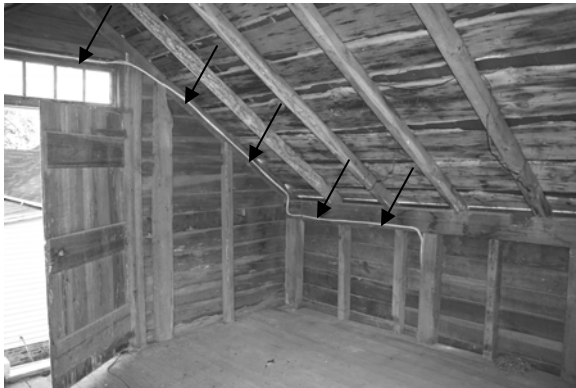
Figure C-61 Romex wiring leading from service point to disconnect box below
