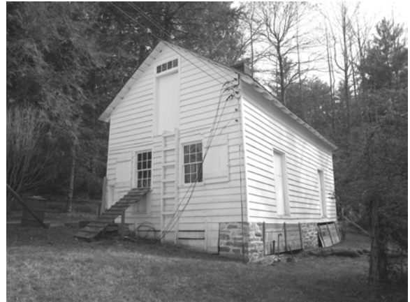
Figure C-1 Northwest oblique of Chicken House/Wash House
