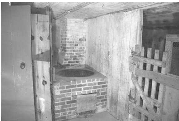
Figure C-50 Room 102B looking southwest
