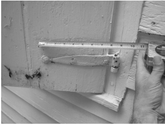
Figure C-20 Window shutter strap hinge, south elevation, east window
