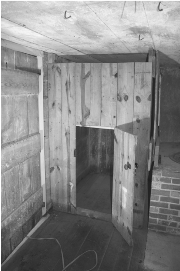
Figure C-44 Room 102B looking southeast
