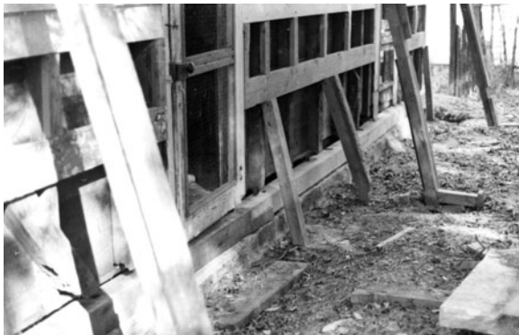
Figure B-12 Sill repairs on east elevation, summer 1978 (CARL4008/05/59P)
