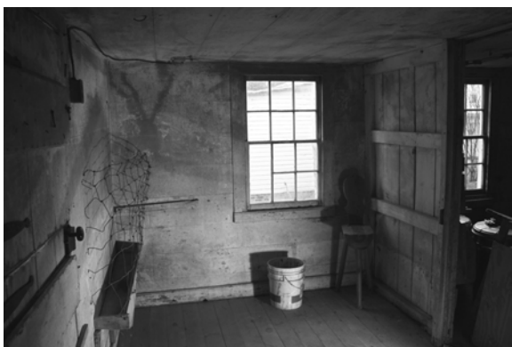
Figure C-35 Room 102A looking north
