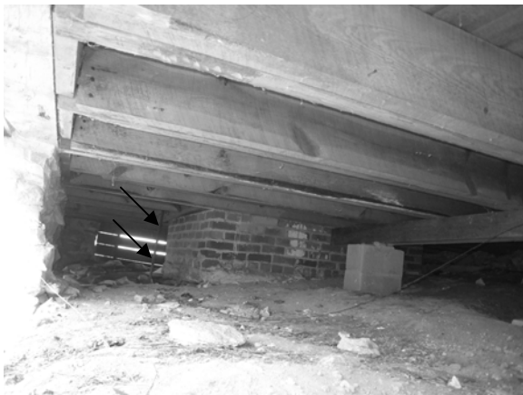
Figure C-28 Crawl space looking northeast, showing base of chimney and galvanized pipe
