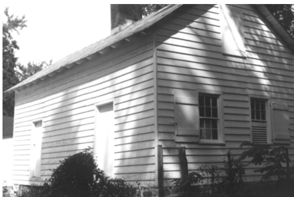
Figure B-18 Southwest oblique of Chicken House, presumably showing completed repairs, 1985 (CARL4004/21-02P)
