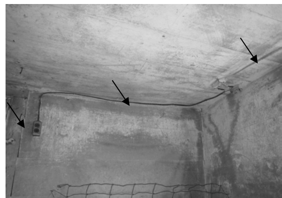
Figure C-38 Outlet and Romex along west wall, two-wire knob and tubing along north wall
