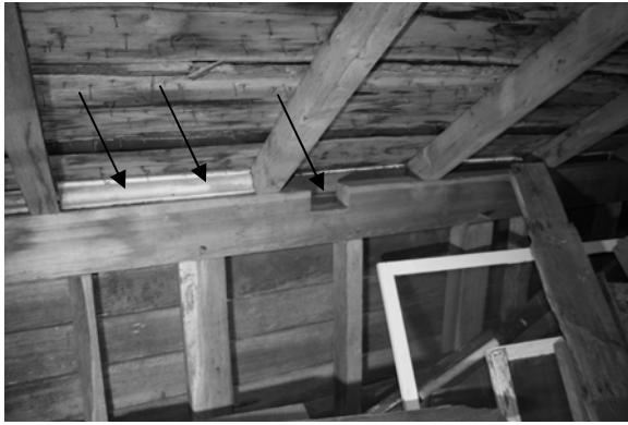
Figure C-54 Notches in top plate suggest collar ties; note painted sections of crown moulding along parts of top plate
