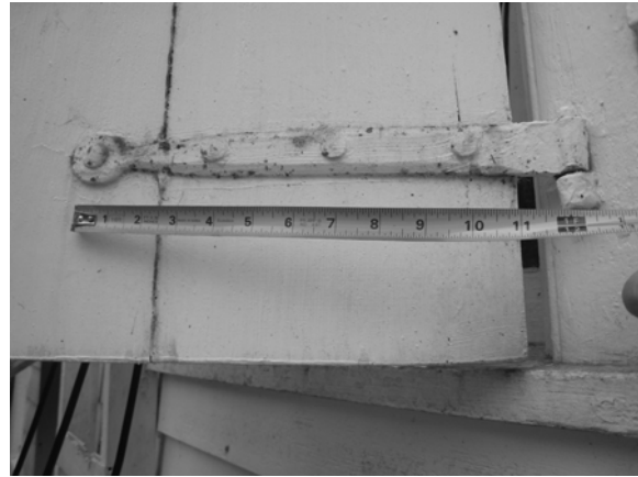
Figure C-23 Window shutter strap hinge, north elevation, west window
