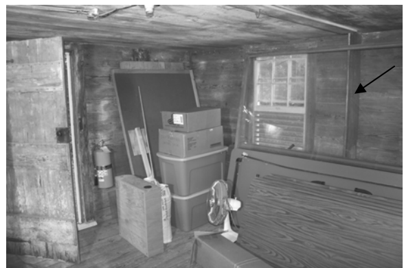
Figure C-31 Room 101B looking southeast, with section of early board wall at right.
