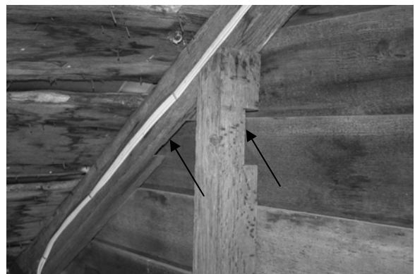
Figure C-59 Notches in studs at north gable end
