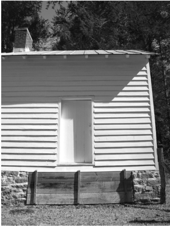
Figure C-9 Wood weatherboard siding and stone foundation walls, west elevation
