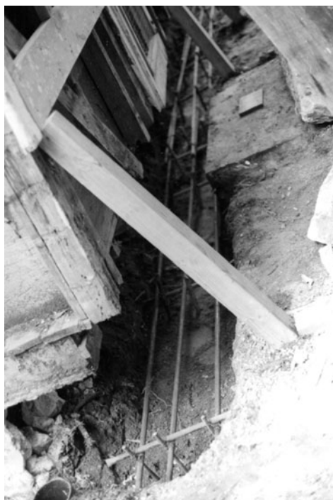
Figure B-13 New reinforced concrete footings, November 10, 1977 (CARL4008/05/35P)
