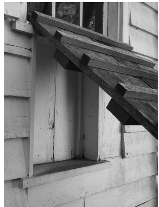
Figure C-26 Detail of ramp and goat door under window on north elevation
