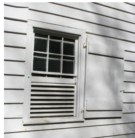
Figure C-19 East window on south elevation
