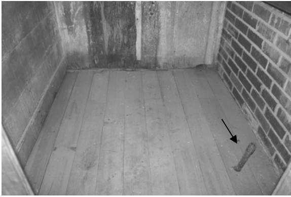
Figure C-48 Galvanized pipe and interior of closet
