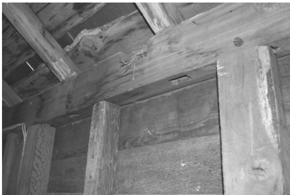
Figure C-5 Larger vertical members mortised into top plate at sides of photo, newer vertical in center toenailed, and empty mortises adjacent
