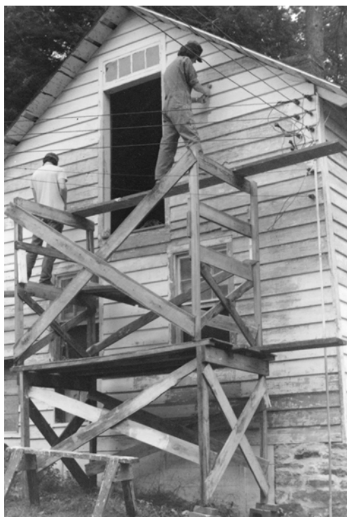
Figure B-14 North elevation being repainted, October 1979 (CARL4004/15-32P)
