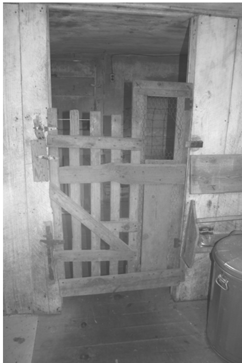
Figure C-45 Door opening with wooden gate on west wall of Room 102B
