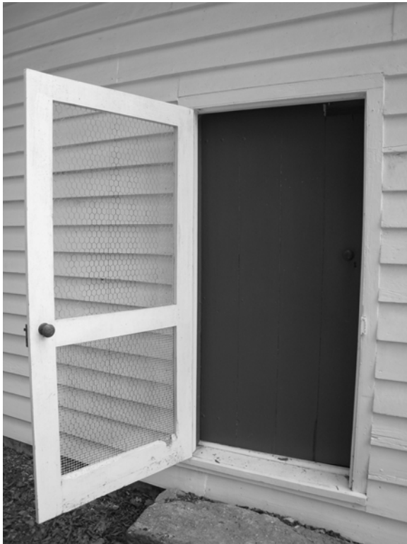
Figure C-10 East elevation, north doorway
