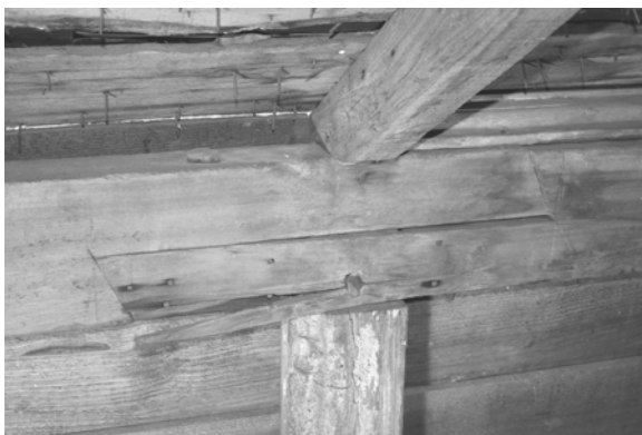
Figure C-4 Wall and roof framing visible in upper half-story
