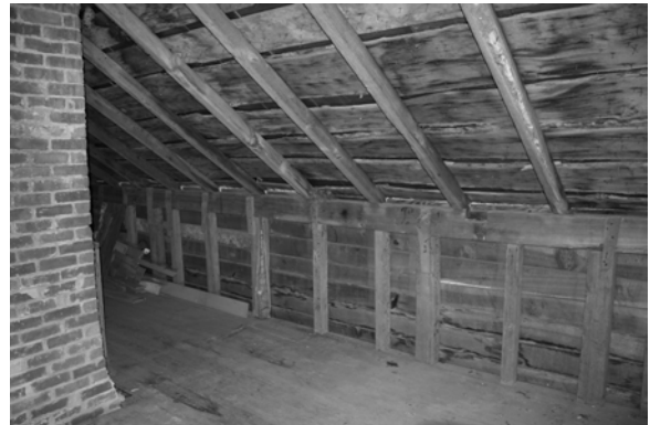
Figure C-58 Room 201B looking southwest
