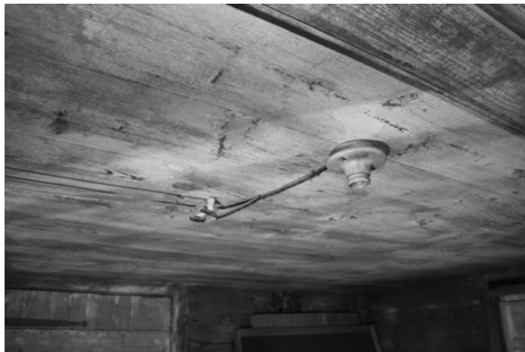
Figure C-34 Ceramic light socket in Room 101B
