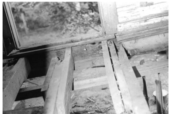
Figure B-10 Flooring removed in Kid room to facilitate joist repairs, Haynes, 1977 (CARL4007/35/09P)
