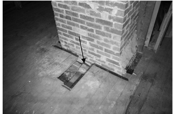
Figure C-63 Painted sections of baseboard discarded in floor cavity
