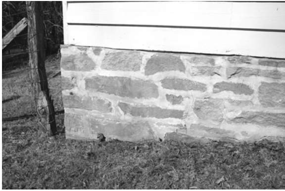
Figure C-3 Stone foundation near west corner of south elevation
