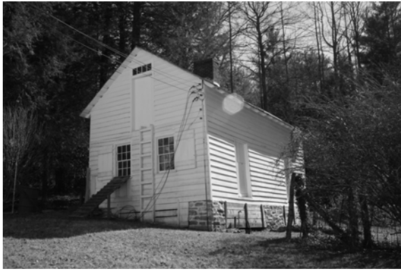
Figure B-1 Northwest oblique of Chicken House/Wash House, February 2007
