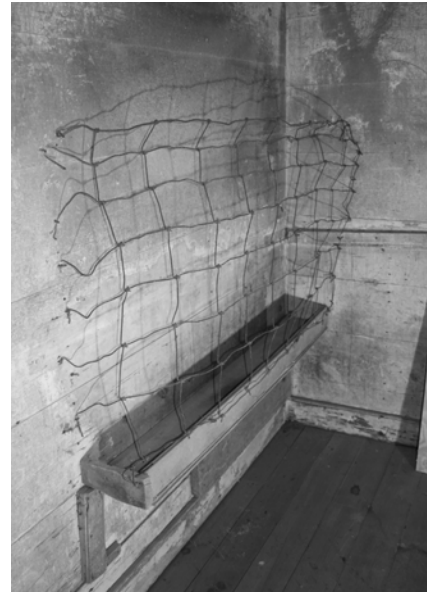
Figure C-42 Wooden trough with wire on west wall
