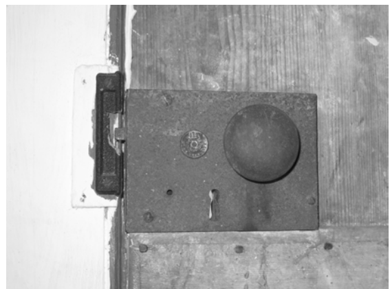
Figure C-13 Rim lock at east elevation, north doorway
