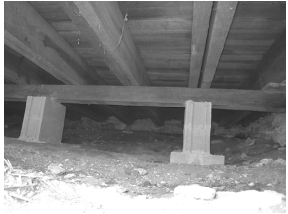
Figure C-6 Floor framing with modern sistered joists and CMU supports
