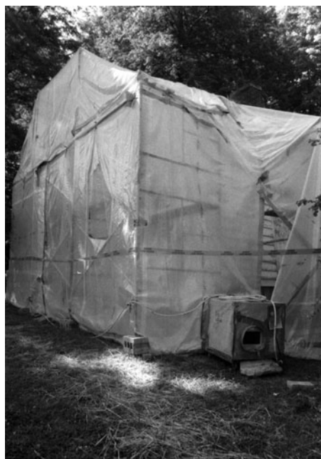
Figure B-19 Northwest oblique, showing tent for lead abatement, 2001 (CARL4018/2-116P)
