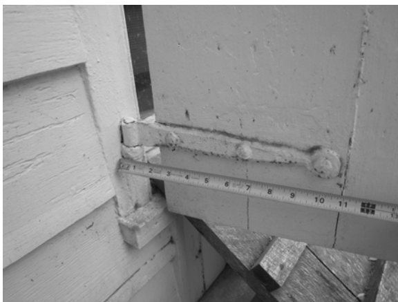
Figure C-22 Window shutter strap hinge, north elevation, east window
