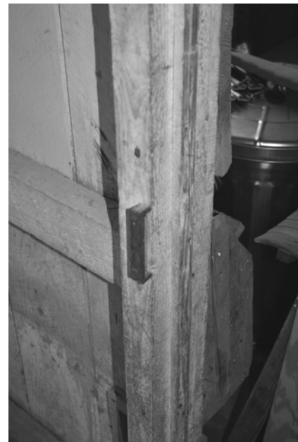
Figure C-37 North jamb of door opening in east wall
