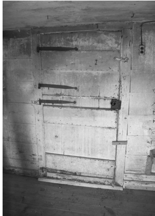
Figure C-11 West elevation, north doorway interior
