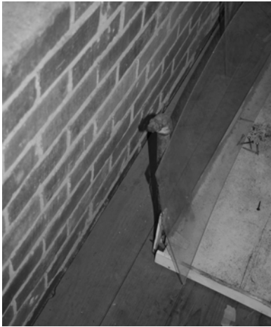
Figure C-39 Galvanized pipe adjacent to wash tubs
