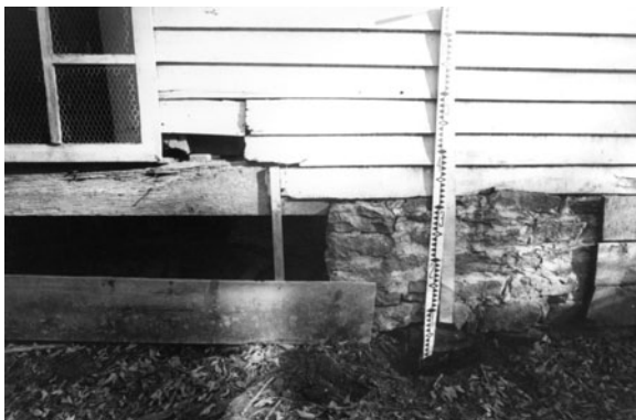
Figure B-8 Partial west elevation, Dec. 1969. (CARL4012/3)
