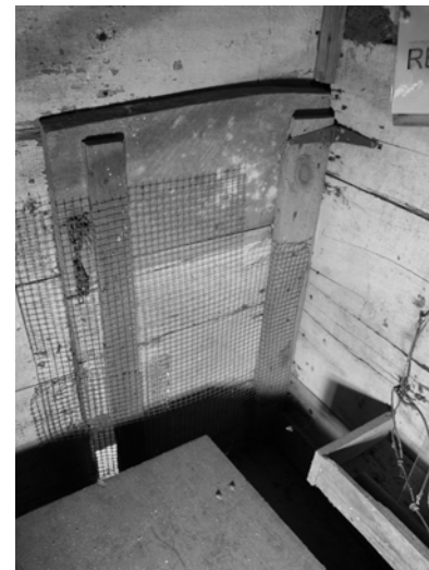
Figure C-53 Hinged goat door on north wall of Room 102B with adjacent feed trough
