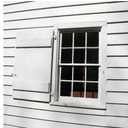
Figure C-18 West window on south elevation
