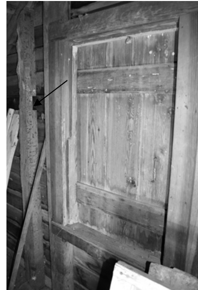
Figure C-57 Window opening at south wall of Room 201A, with shutter closed and stud notch indicated
