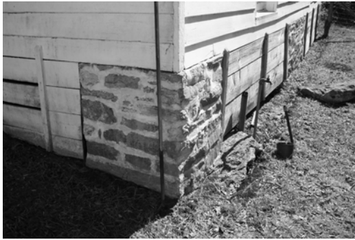
Figure C-27 Northwest corner of building showing wooden panels at foundation level
