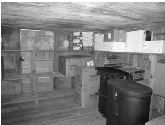
Figure C-29 Room 101A looking northwest, showing modern wood shelving
