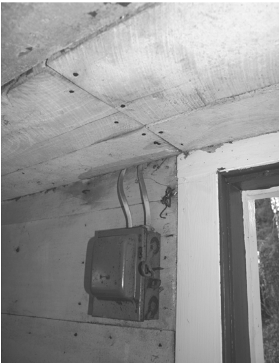
Figure C-49 Disconnect box on east wall of Room 102B, with adjacent replacement ceiling boards
