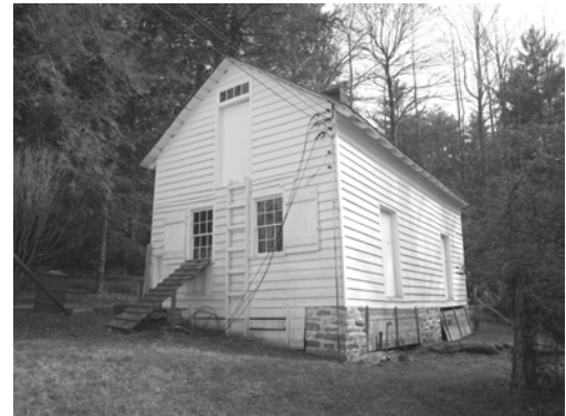
Figure C-25 Northwest oblique, showing ladder and ramp on north elevation of building
