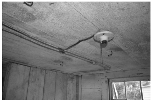
Figure C-47 Ceramic light socket and knob-and-tube wiring in Room 102B
