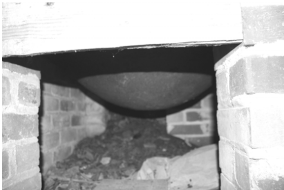
Figure C-41 View inside firebox under wash tub
