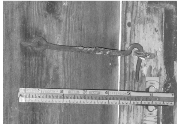
Figure C-24 Wrought-iron hook at upper-story window shutter
