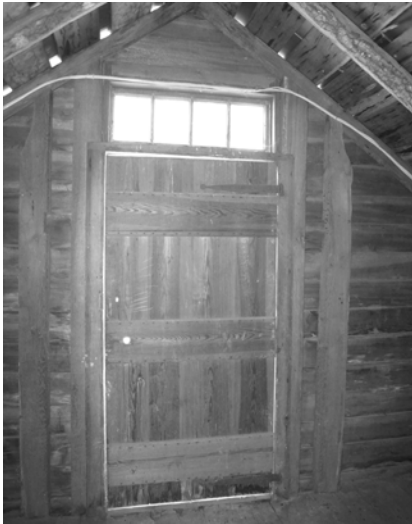
Figure C-60 Door opening and transom on north wall of Room 201B
