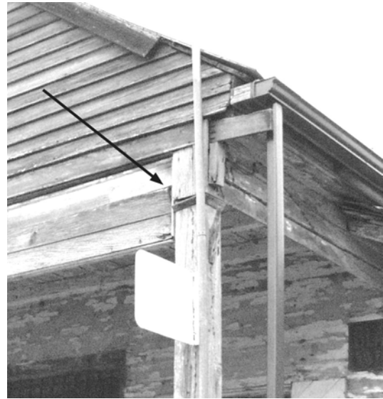
Figure 27 View of northeast corner of building, showing mixture of exterior finishes. Arrow notes original detail of post top. (NPS-SERO-CRS, 2001)
