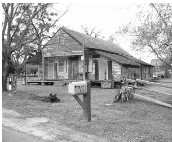
Figure 13 View of Store from northeast. (NPS-SERO-CRS, 2001)
