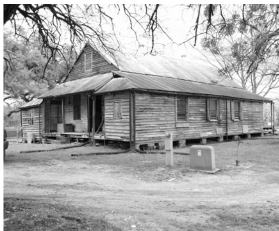
Figure 14 View of Store from southwest. (NPS-SERO-CRS, 2001)
