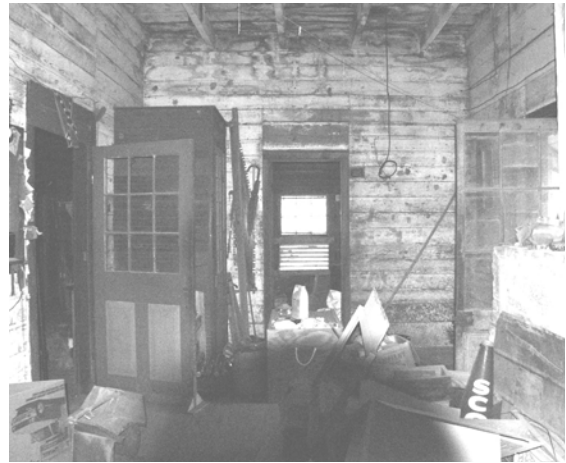
Figure 41 View south in office (006). (NPS-SERO-CRS, 2001)
