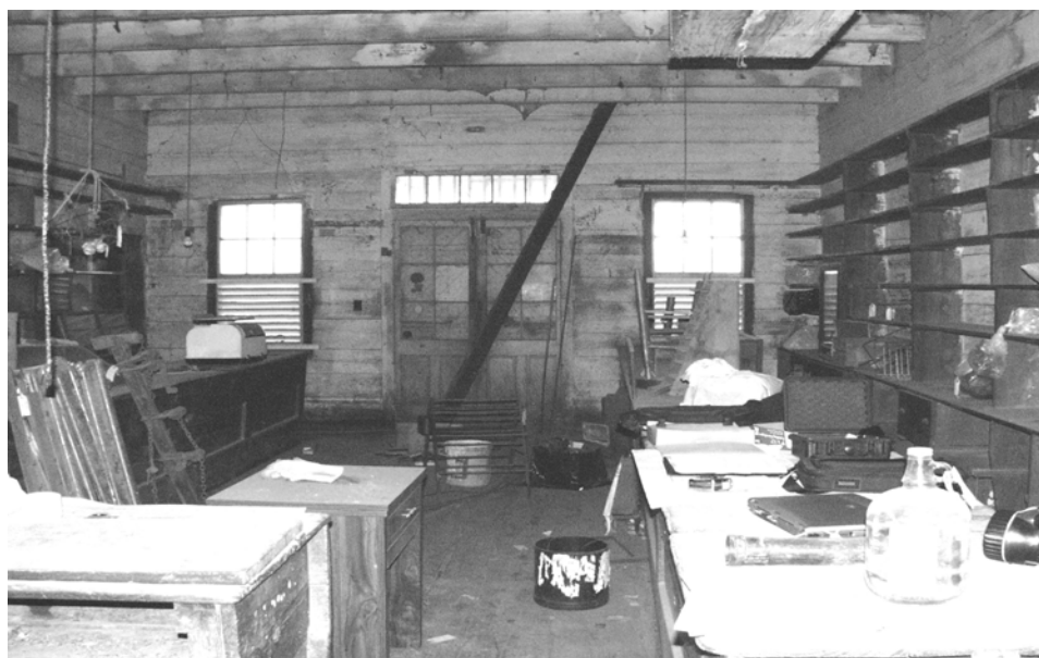
Figure 31 View east in 002. (NPS-SERO-CRS, 2001)
