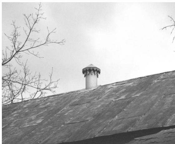
Figure 20 View of south shed of roof with original ventilator (c. 1900). (NPS-SERO-CRS, 2001)
