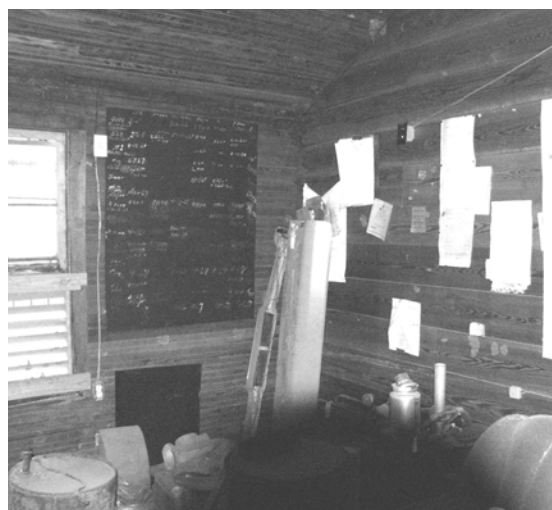
Figure 45 View southwest in record room (007). (NPS-SERO-CRS, 2001)
