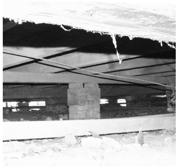
Figure 18 View of floor framing beneath original building. (NPS-SERO-CRS, 2001)
