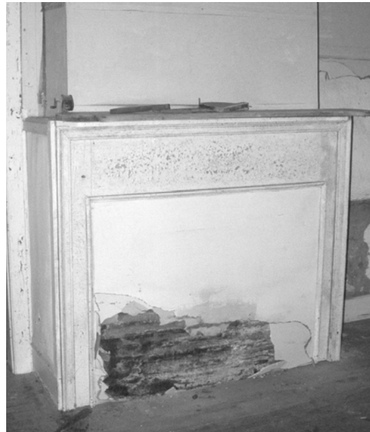
FIGURE 55. Fireplace #2 in Room 103.
