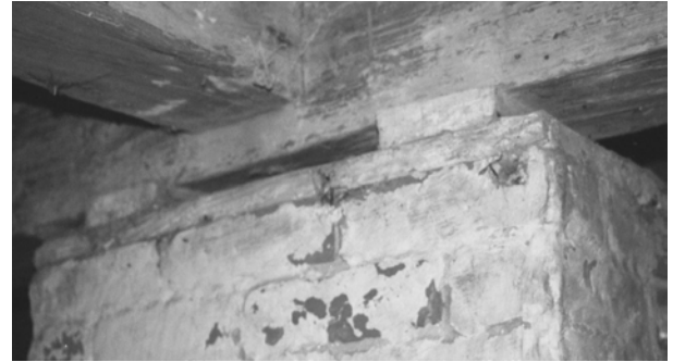
FIGURE 8. Detail of wood blocking between pier and floor framing.
