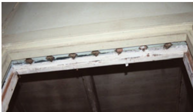
Evidence of original bars Window 11, Room 103
