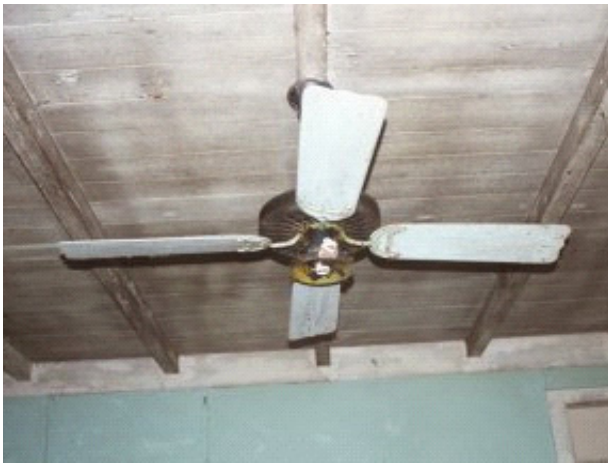
FIGURE 52. Ceiling in Room 103.
