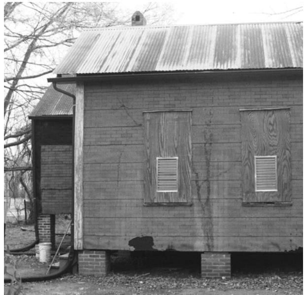
FIGURE 32. Room 110 wing, northwest elevation.
