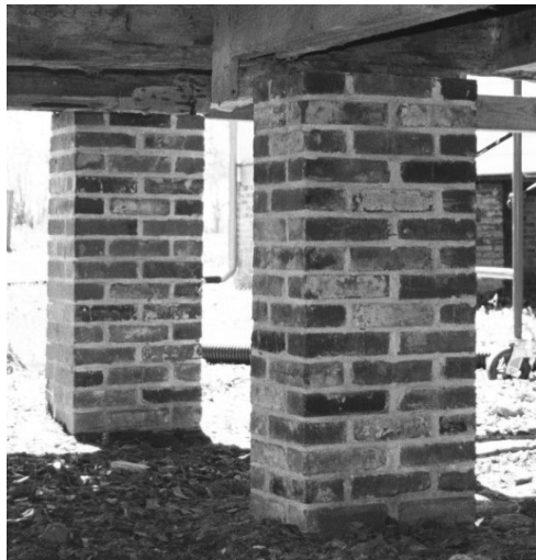
FIGURE 3. Foundation piers beneath Room 111 addition.
