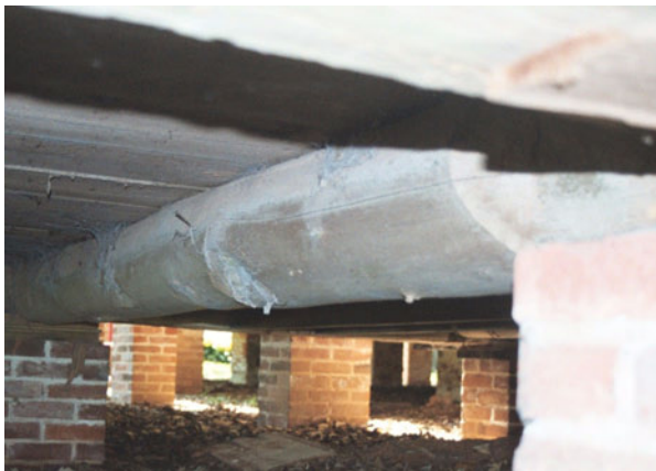
FIGURE 17. Log joist in floor framing of Room 110 addition.
