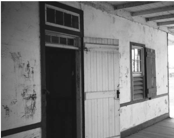
FIGURE 30. Southwest exterior walls at Rooms 103 and 104.
