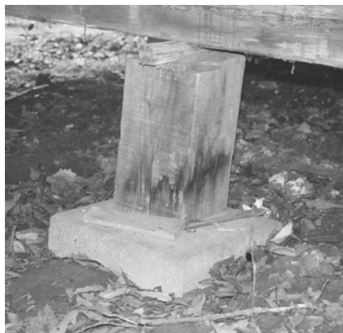
FIGURE 4. Odd pier beneath southwest sill of Room 110 addition.
