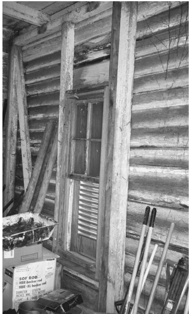
FIGURE 65. Northwest wall, Room 110.
