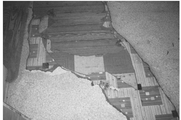
FIGURE 54. Floor in Room 105.
