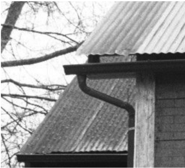
FIGURE 34. Corrugated roofing on additions (Rooms 110 and 111).
