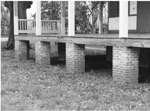
FIGURE 2. Foundation piers beneath southeast sill of southeast gallery.
