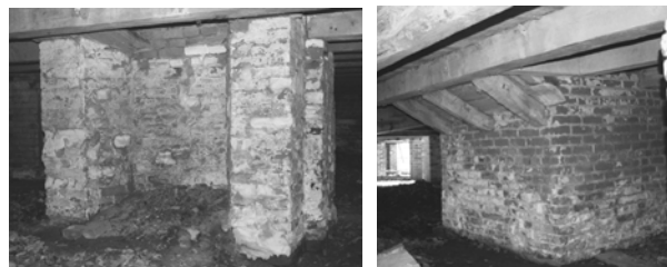
FIGURE 12. Left, brick foundation of Fireplace 1, Room 104; right, brick foundation of Fireplace 2 (Room 103) and 3 (Room 102).
