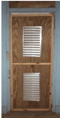
Door 4, Temporary Interior
