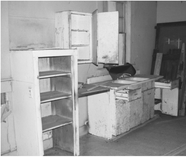
FIGURE 56. Cabinets and sink in Room 105.
