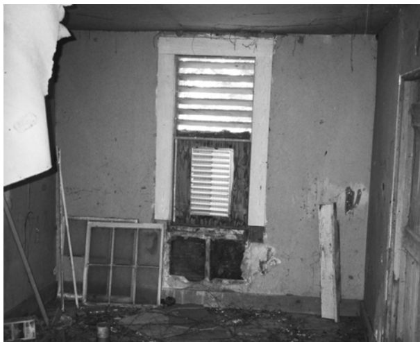
FIGURE 67. Northeast wall, Room 111.
