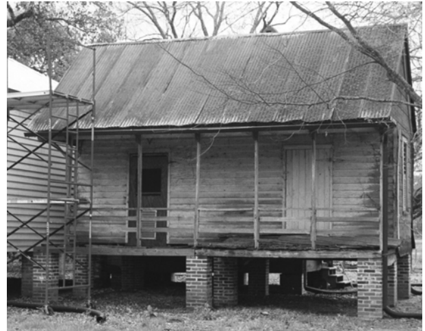
FIGURE 31. Room 111 wing, southeast elevation.
