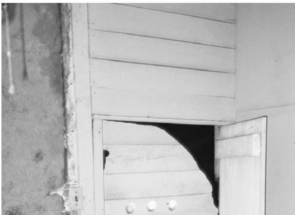
FIGURE 58. East corner of Room 106.
