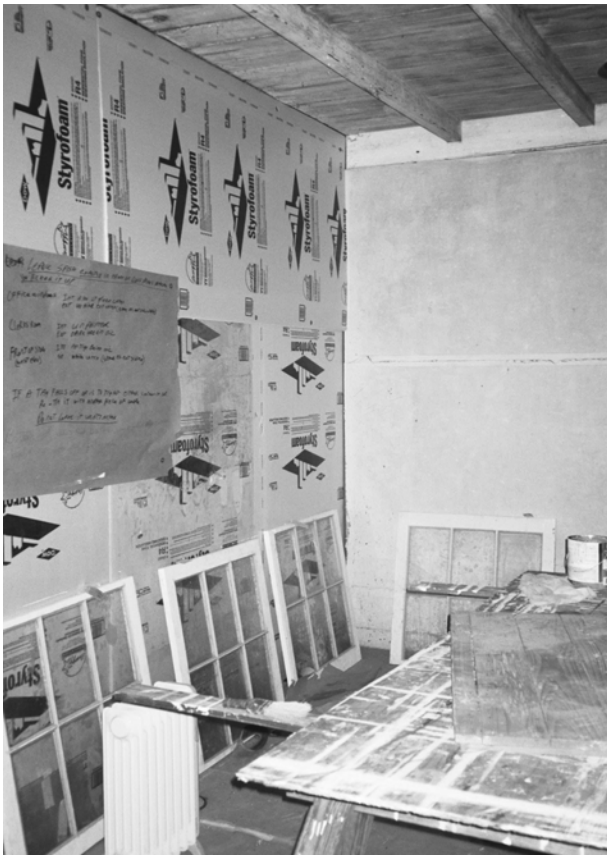
FIGURE 48. Room 102, looking north.
