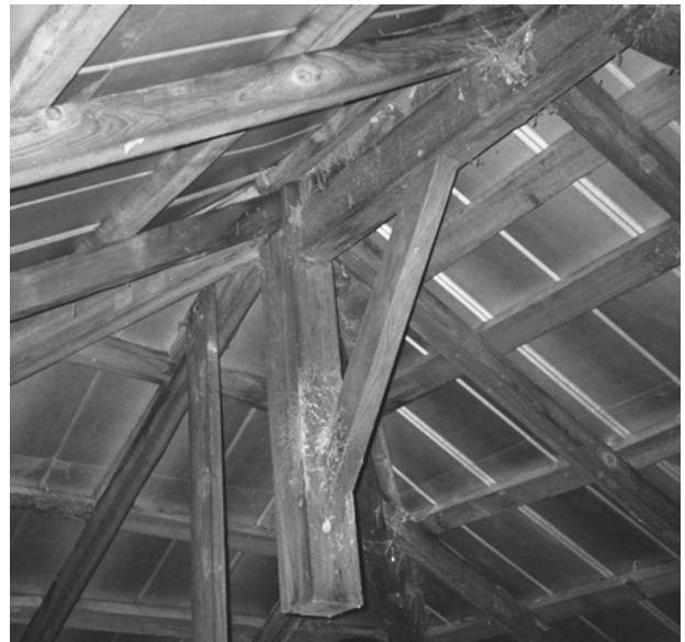
FIGURE 21. Framing at hip in roof. Note difference in end of king post.
