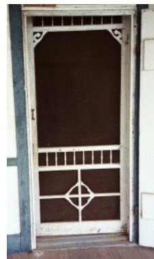
Door 5, Interior Screen Door
