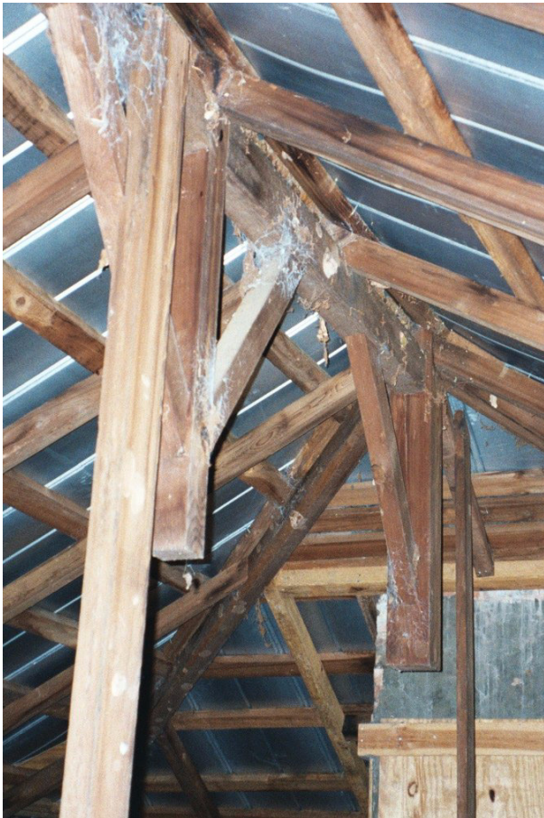
FIGURE 23. King post in center of attic supporting ridge beam.
