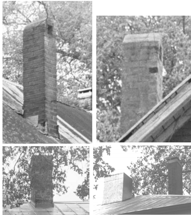
FIGURE 9. Chimneys for stove in Room 111, upper left; for stove in Room 110, upper right; fireplace in Room 104, lower left; and for fireplaces in Room 101, Room 102, and Room 103.
