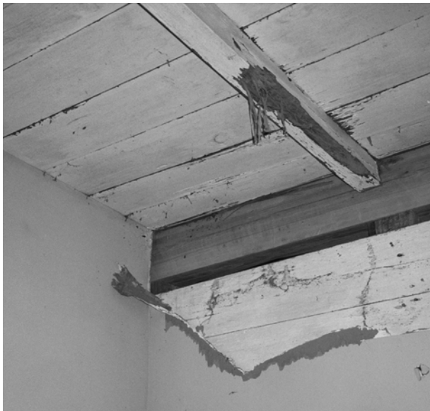
FIGURE 45. Room 101 ceiling and southwest wall.
