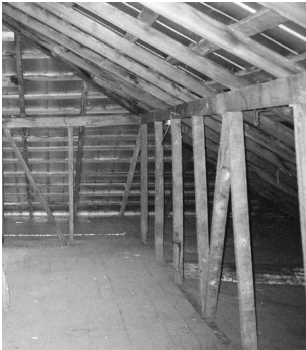
FIGURE 24. Knee walls in attic, looking northwest.
