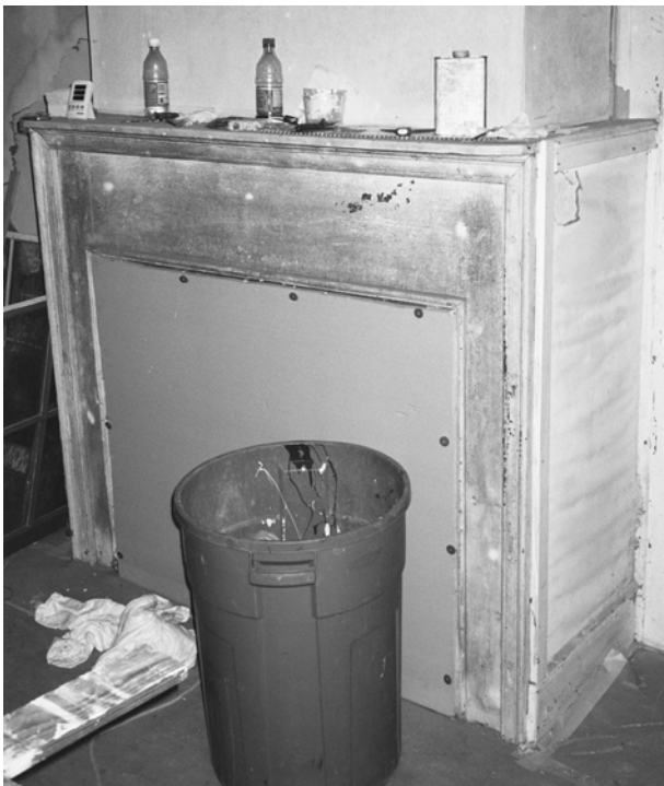
FIGURE 47. Fireplace #3 in Room 102.
