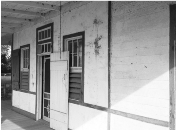
FIGURE 29. Southwest exterior walls at Rooms 104 and 105.
