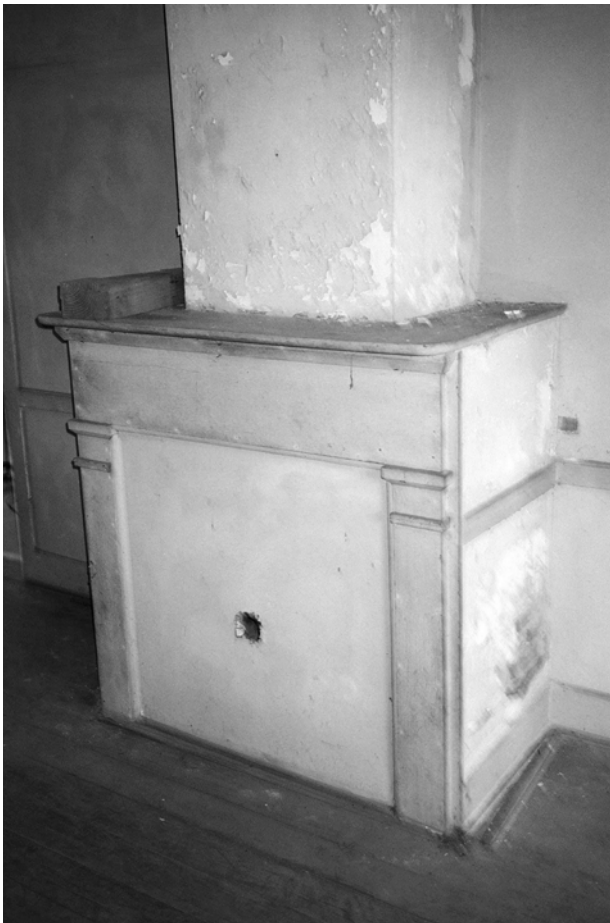
FIGURE 43. Fireplace #4 in Room 101.
