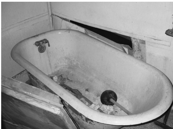
FIGURE 63. Room 109, bath tub.
