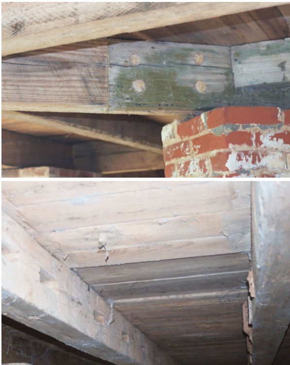
FIGURE 15. Above, pegged connections in historic floor framing; below, recycled joist in northwestern section of floor framing.
