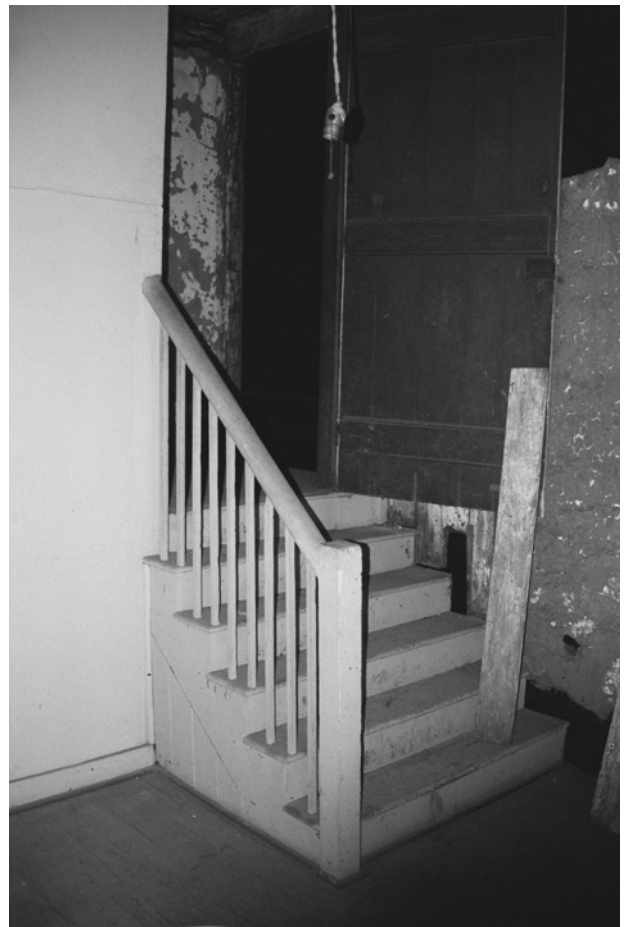
FIGURE 59. Attic stairs in Room 106.
