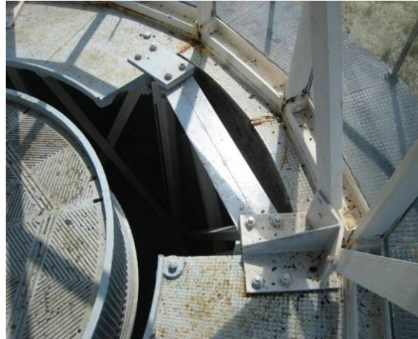
Figure C-102 Access to stairs to Watch Level partially blocked by 1989 reinforcing steel.
