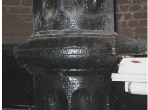
Figure C-14 Bolted connection between column sections.
