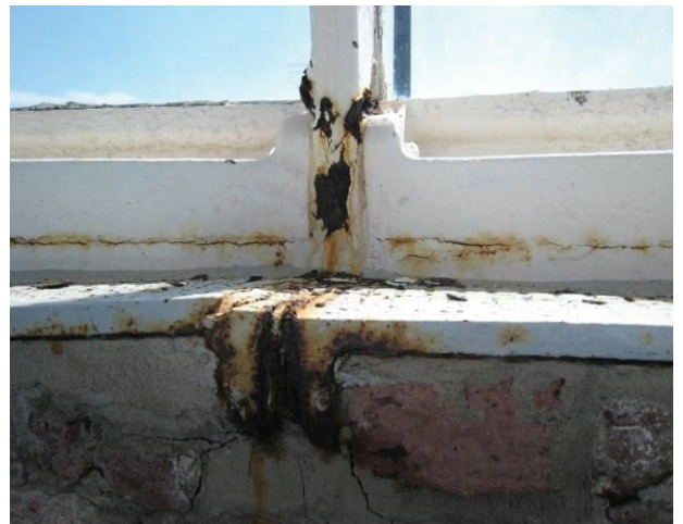
Figure C-104 Extensive corrosion of cast-iron framing.
