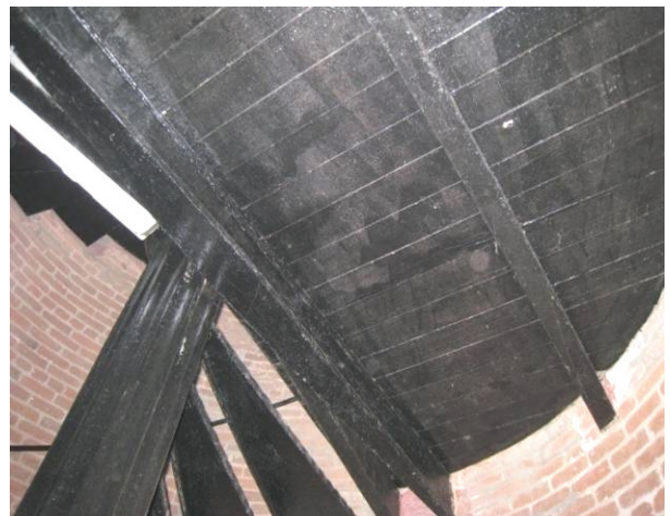
Figure C-66 Third Floor wood Landing.
