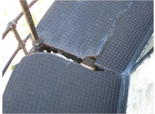
Figure C-23 Broken floor plates of Lantern Gallery.
