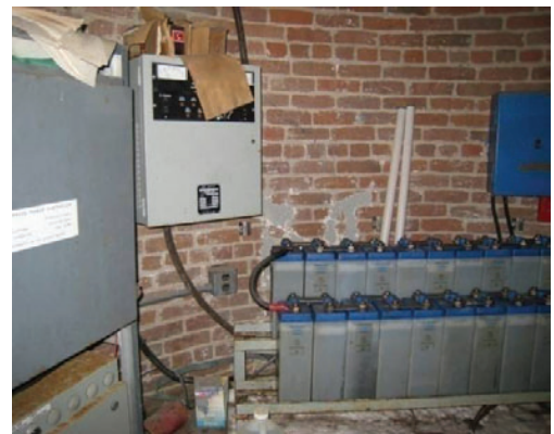
Figure C-58 Abandoned power controller and fuel cells.
