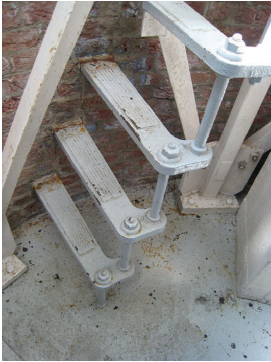
Figure C-90 Close-up view of ship's ladder to Lantern.
