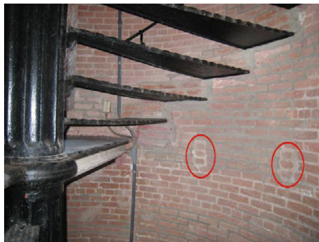
Figure C-68 Two masonry patches presumably associated with the 1864 framing for temporary stairs.
