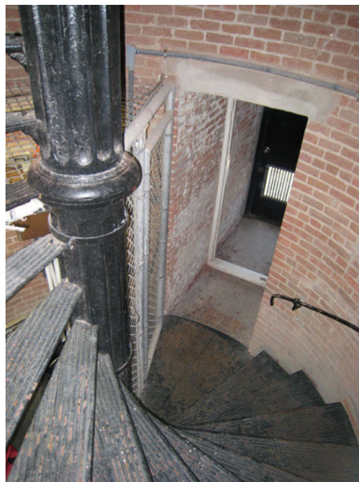
Figure C-64 Second Floor entrance passageway, spiral stairs, and modern steel fence enclosure.
