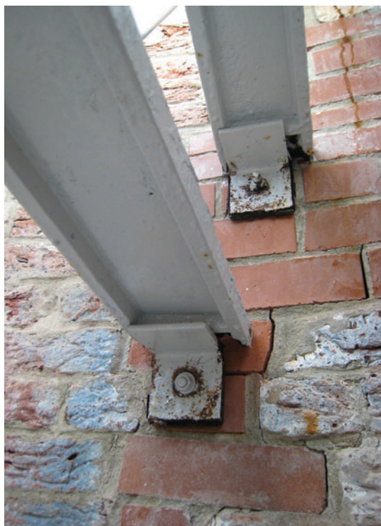
Figure C-8 Modern masonry repairs in Watch Room.
