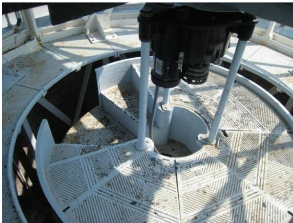
Figure C-97 Center cast-iron platform for beacon.
