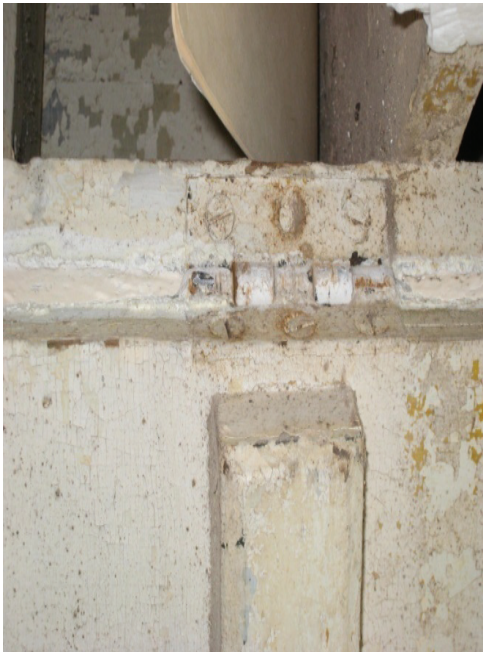
Figure C-94 Cabinet's five-knuckle hinge and batten.
