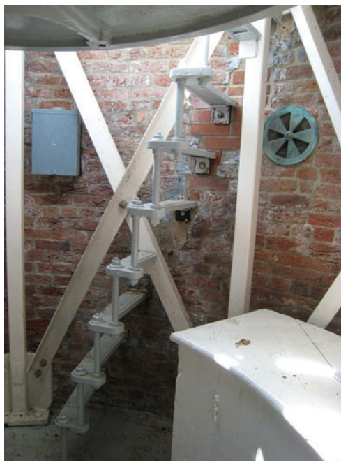
Figure C-89 Original cast-iron ship's ladder to Lantern.
