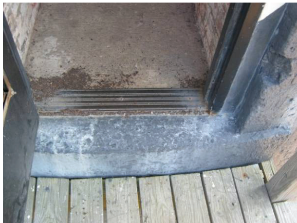
Figure C-40 Granite doors sill at Second Floor entrance. Note modern infill, door frame, and door.
