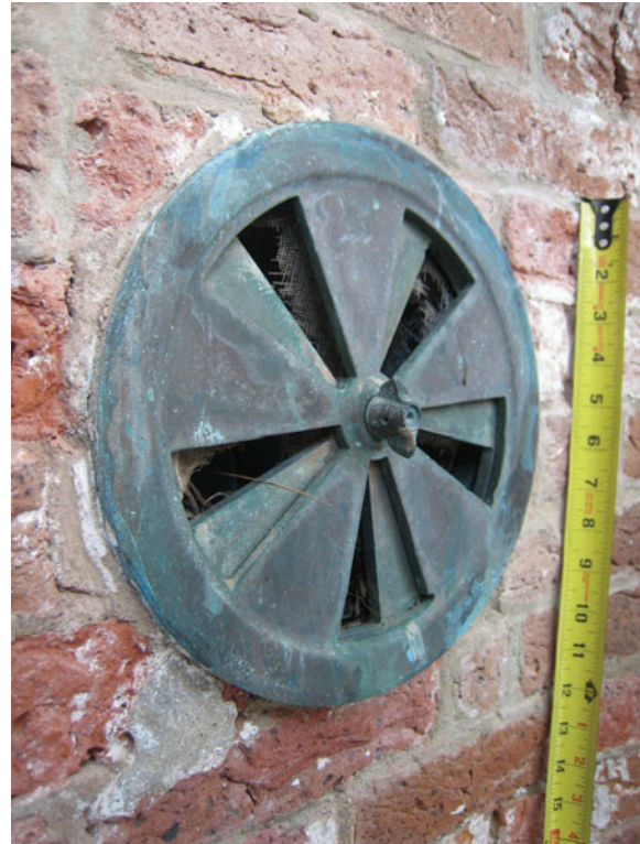
Figure C-95 Brass manual control for adjusting air flow.
