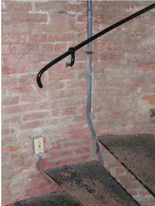
Figure C-46 Original iron handrail of 1-inch diameter.
