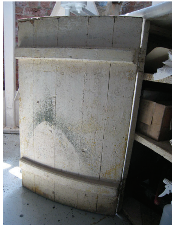
Figure C-92 Curved interior face of board-and-batten cabinet door.
