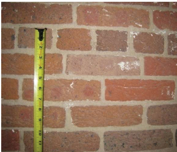
Figure C-9 Brickwork of interior face of core wall.
