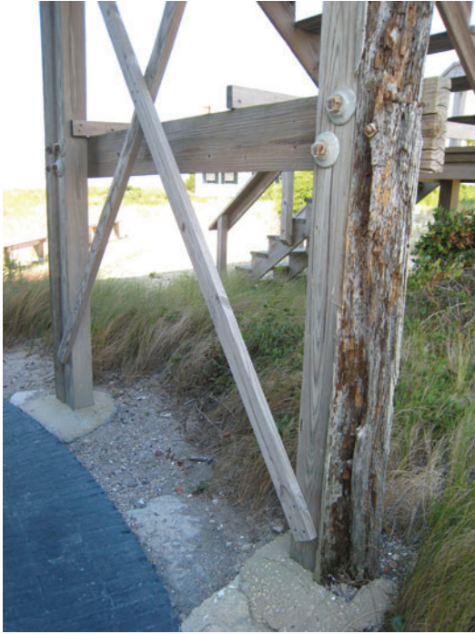
Figure C-34 Two earlier but twentieth-century and severely deteriorated wood posts and one cross beam
