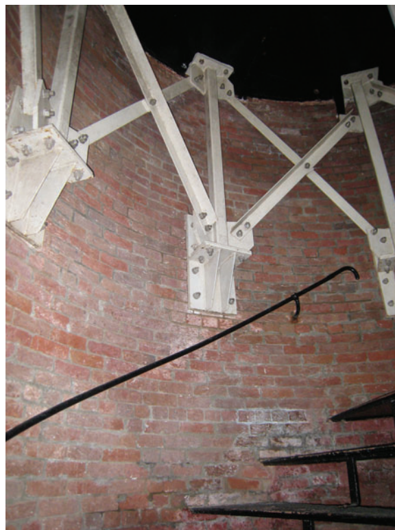
Figure C-16 1989 steel framing at Seventh Floor.
