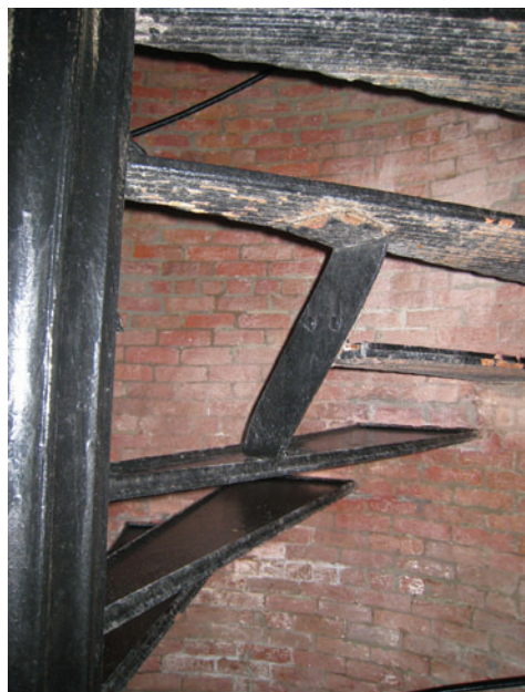
Figure C-73 1914 tread modification to accommodate the weight for occulting mechanism.
