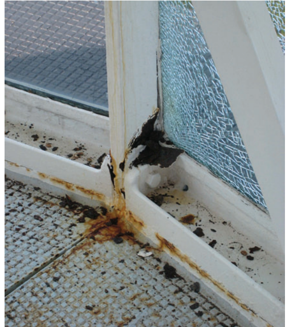
Figure C-98 Deteriorated iron framing.
