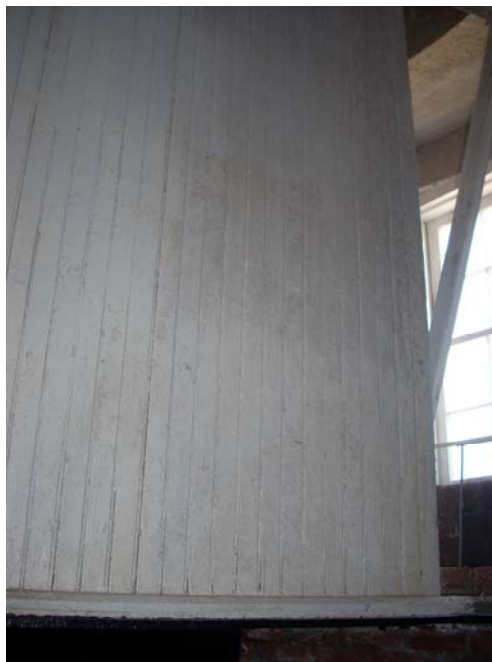
Figure 5 – Bracing Interrupting Partition Wall at Storage Area
