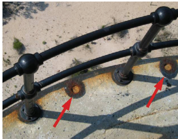
Figure C-25 Remnants of 1914 stanchion anchors and replacement railings of unknown date.
