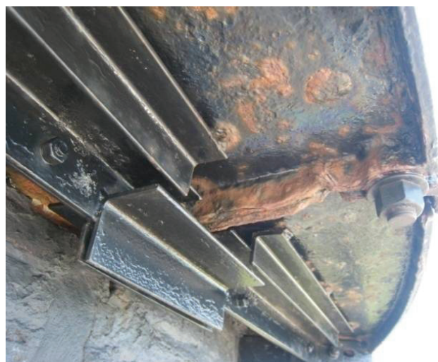
Figure C-106 Underside of Lantern Gallery reinforced in 1989.
