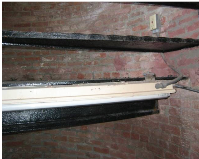
Figure C-19 Typical shop-type utility lighting at spiral stairs floor landing.
