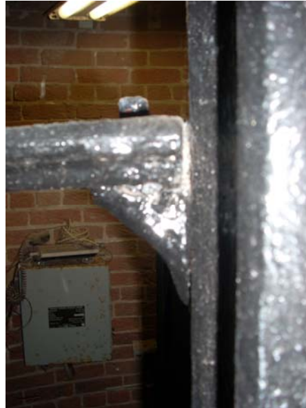
Figure 3 – Pin Connection at Interior Support Column
