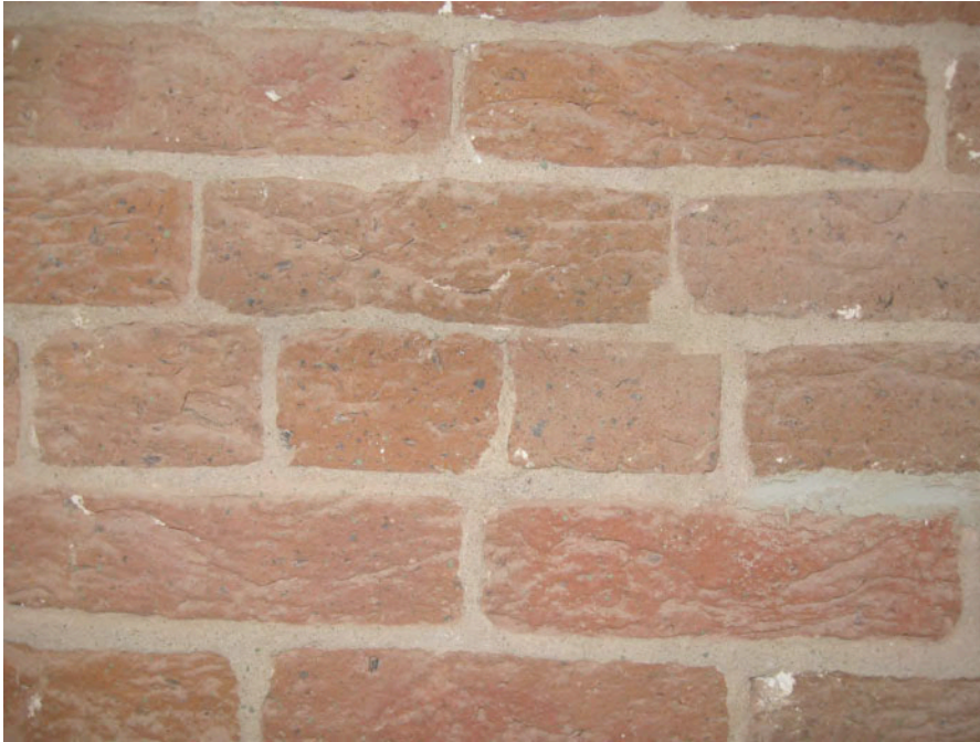
Figure 19. Cape Lookout Lighthouse, September 2008. Area of typical interior brickwork showing the brick's hand-pressed, low-fired quality and appearance. Photograph by author.
