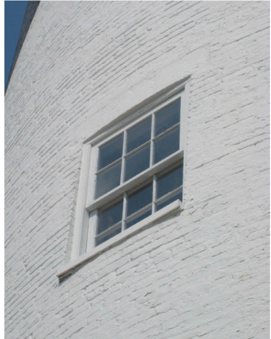
Figure C-32 Typical replacement window unit.
