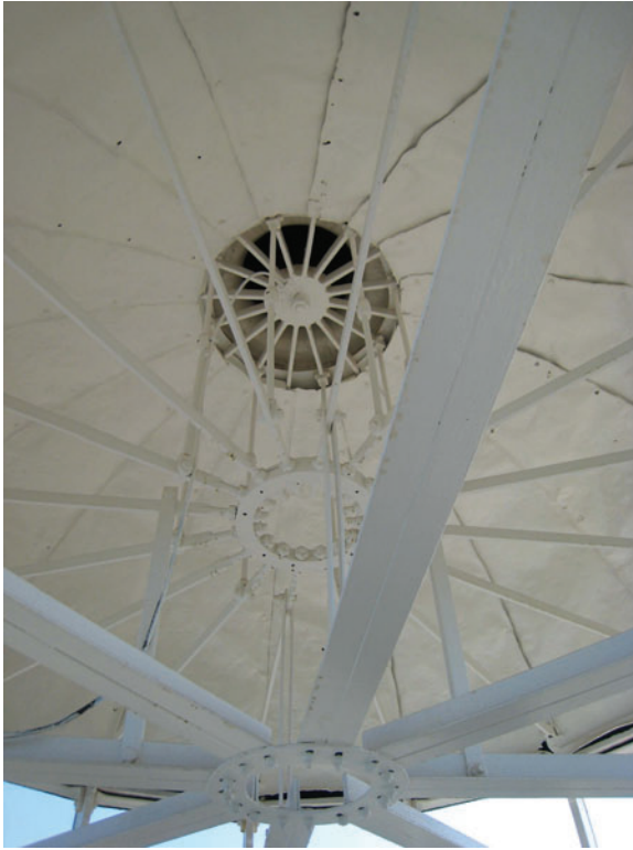
Figure C-17 Structural supports and central ventilator of dome.
