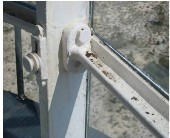
Figure C-99 Close-up view of horizontal framing of a cast copper-based metal.
