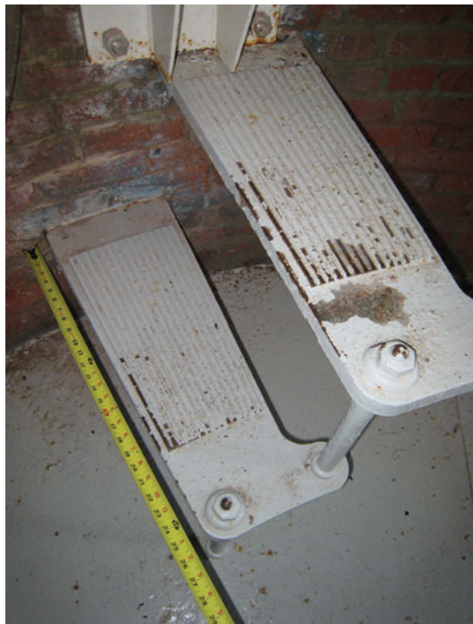
Figure C-82 Original cast-iron ship's ladder stairs connecting Seventh Floor Service Room to Eighth Floor Watch Room.
