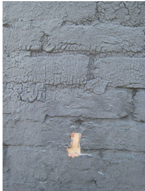
Figure C-108 Non-breathable coating on exterior masonry.
