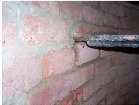
Figure 2 – Stair Connection at Exterior Masonry Wall
