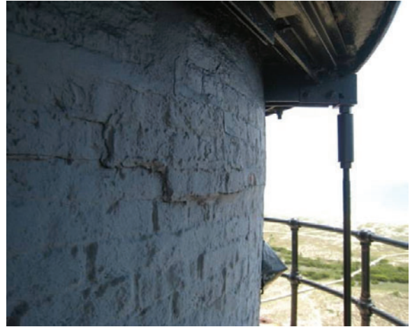
Figure C-107 Displaced masonry and supplemental tie rods.
