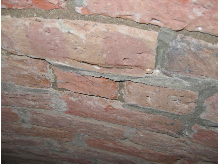
Figure 20. Cape Lookout Lighthouse, September 2008. An area where inappropriate Portland cement based re-pointing mortar has caused the original brick to spall and the original mortar to deteriorate. Photograph by author.
