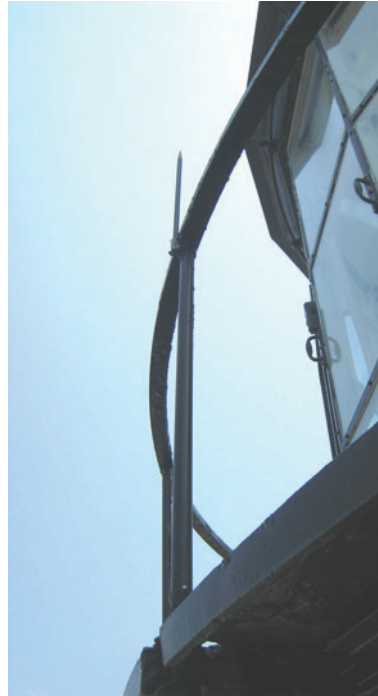
Figure C-36 Modern lightning rod at Gallery railing.
