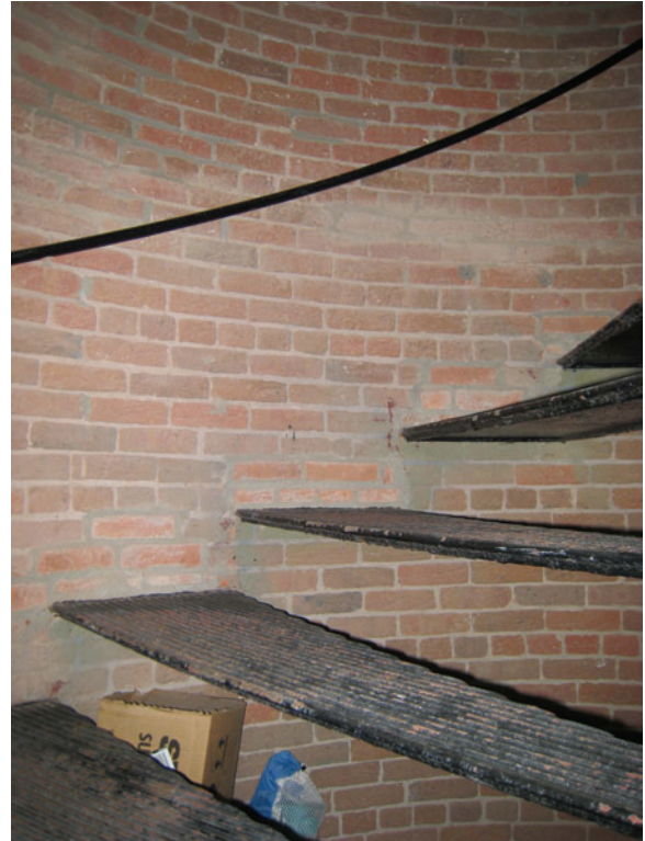
Figure C-62 Typical cast-iron treads of Spiral Staircase.
