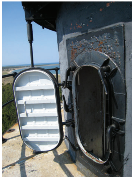
Figure C-30 Ship's Hatch at Observation Deck
