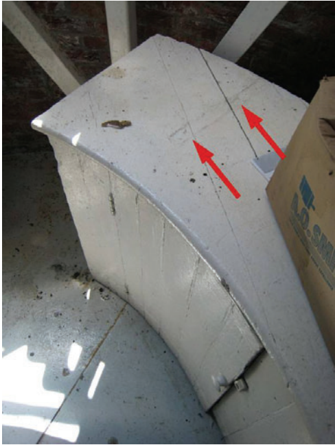
Figure C-93 Ghost marks of missing shelving supports.
