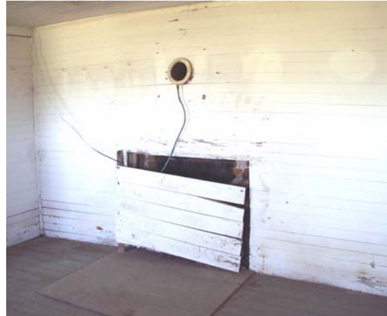
Figure 18 View of fireplace opening in Room 101. (NPS-SERO-CRS, 2001)
