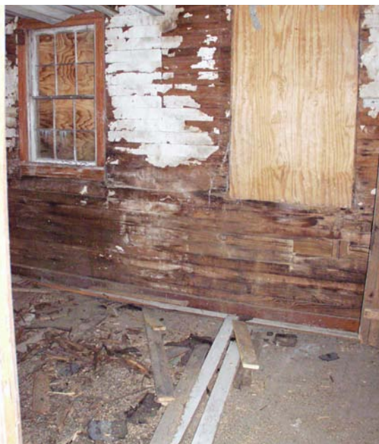
Figure 24 View south in Room 201. (NPS-SERO-CRS, 2001)
