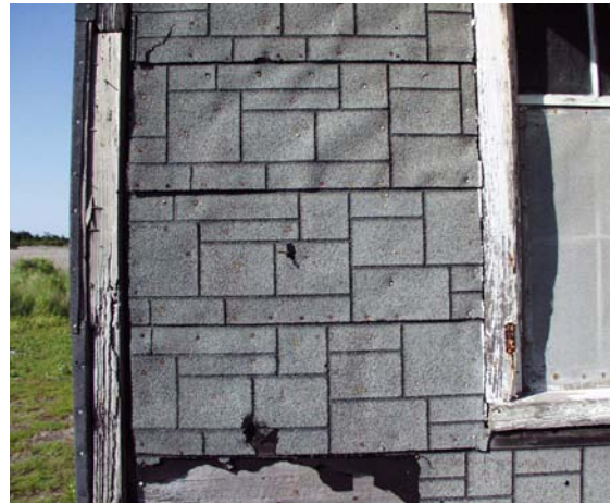
Figure 14 View of added asphalt siding. Note part of shutter hinge on adjacent window casing, which is original. (NPS-SERO-CRS, 2002)
