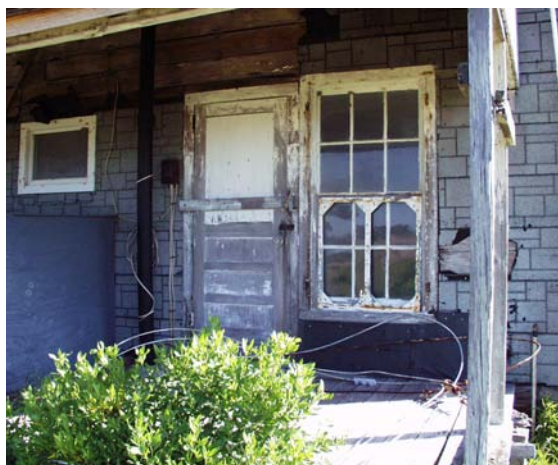
Figure 13 View of original, 6/6 window with typical wood frame for screening. Original location for back door opening was at window at extreme left in this image. (NPS-SERO-CRS, 2002)
