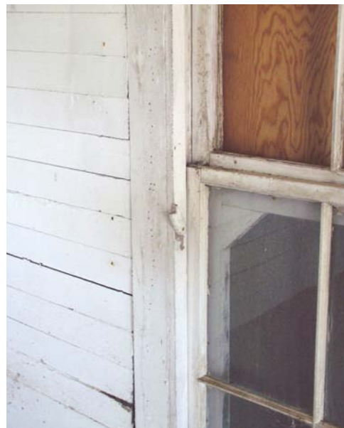
Figure 19 View of typical window casing and wall paneling. Note pivoting sash stay at center, typical of original windows. (NPS-SERO-CRS, 2001)
