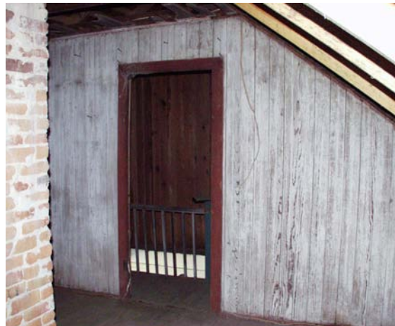
Figure 27 View south in Room 202. (NPS-SERO-CRS, 2002)
