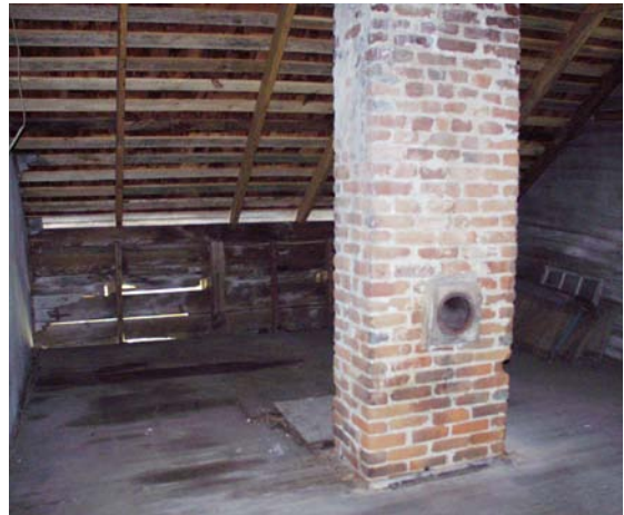
Figure 26 View west in Room 202. (NPS-SERO-CRS, 2002)
