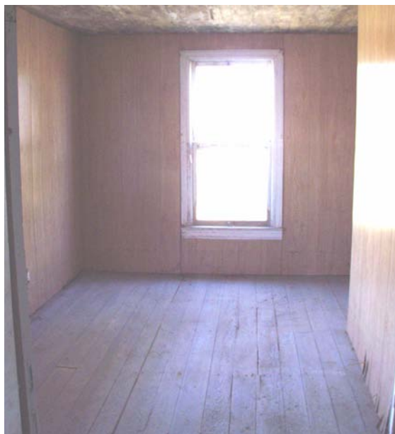
Figure 20 View north in Room 101, showing window that infills earlier door to now-missing kitchen wing. (NPS-SERO-CRS, 2002)
