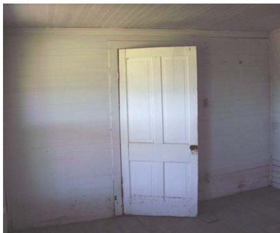
Figure 17 View of south wall of Room 101, showing typical door in house. (NPS-SERO-CRS, 2002)
