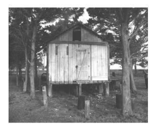
**Figure 5** View of southwest end of house; note piers in foreground which supported the modern addition that was removed after 1984. (NPS-SERO-CRS, 2001)
