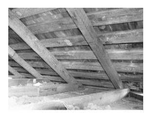
**Figure 9** View of southeast shed of roof; note wood shingles still in place. (NPS-SERO-CRS, 2001)
