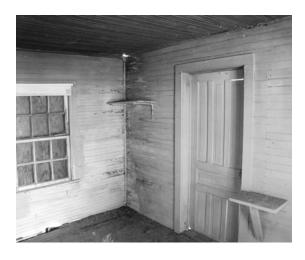
**Figure 17** View south in Room 101. Door to right was originally a window opening, converted into a door to the addition in the 1950s. (NPS-SERO-CRS, 2001).
