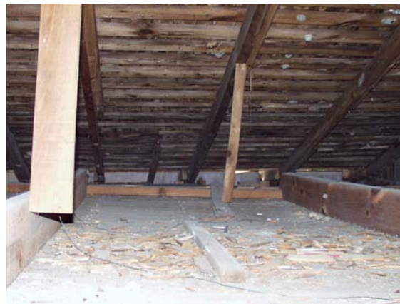
Figure 22 View to southeast in attic of original house. (NPS-SERO-CRS, 2002)
