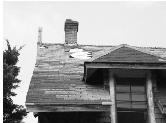
Figure 49 View of existing roofing. White “hurricane” asphalt shingles installed in early 1950s are exposed just below the chimney. (NPS-SERO-CRS, 2002)
