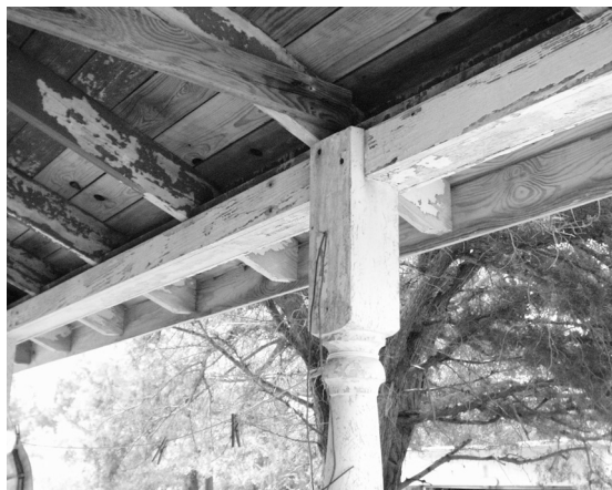
Figure 58 View of typical post, header and roof framing on rear porch. (NPS-SERO-CRS, 2002)
