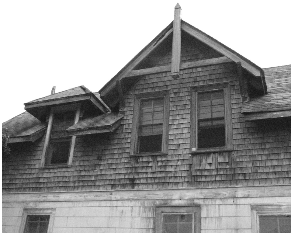
Figure 54 View of typical exterior sidings, with wood shingles at second floor and asbestos over drop siding at first floor. (NPS-SERO-CRS, 2002)
