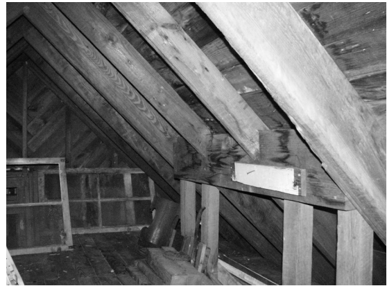
Figure 48 View of roof framing at northeastern end of the building. Rafter at upper right is original; the next two, which are smaller, infill the original opening for the lookout. (NPS-SERO-CRS, 2002)
