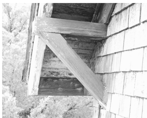
Figure 55 View of typical gable eave bracket. (NPS-SERO-CRS, 2002)
