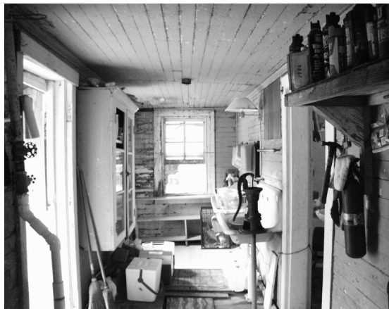
Figure 64 View south in Room 100, showing location of original entry porch. Door opening at left replaced a window in the original configuration of the space. (NPS-SERO-CRS, 2002)
