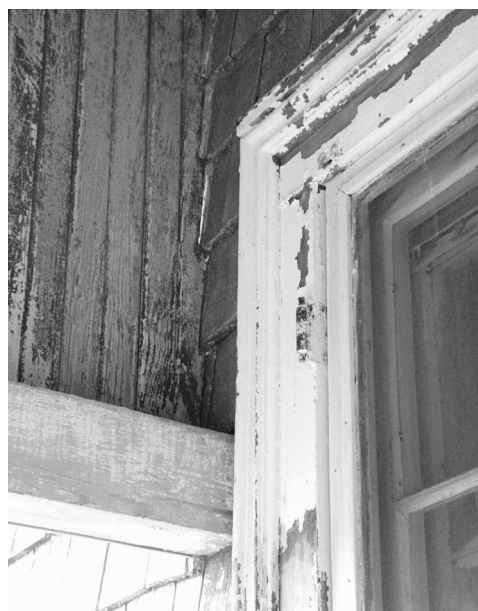
Figure 56 Typical second-floor window casing with added backband. (NPS-SERO-CRS, 2002)
