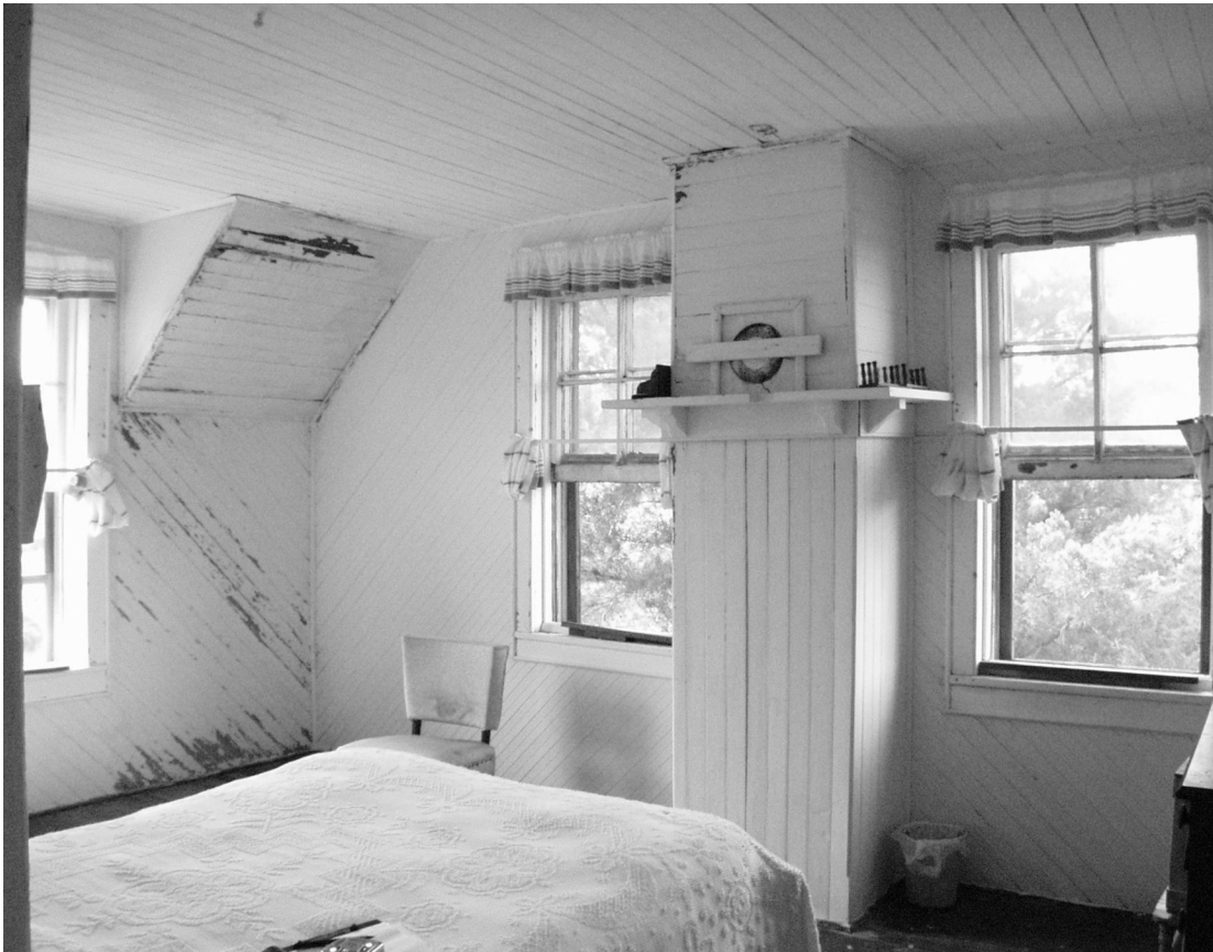
Figure 76 View to south in old keeper's room (Room 202). Note original paneling and plate rail around chimney rising between the two windows on the south wall. (NPS-SERO-CRS, 2002)
