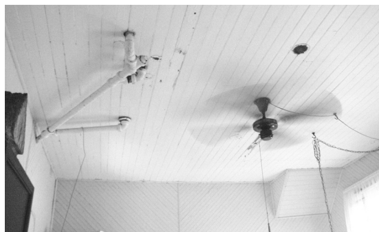
Figure 70 View of ceiling in Room 102, showing cast-iron waste lines (c. 1920) from upstairs bathroom. (NPS-SERO-CRS, 2002)
