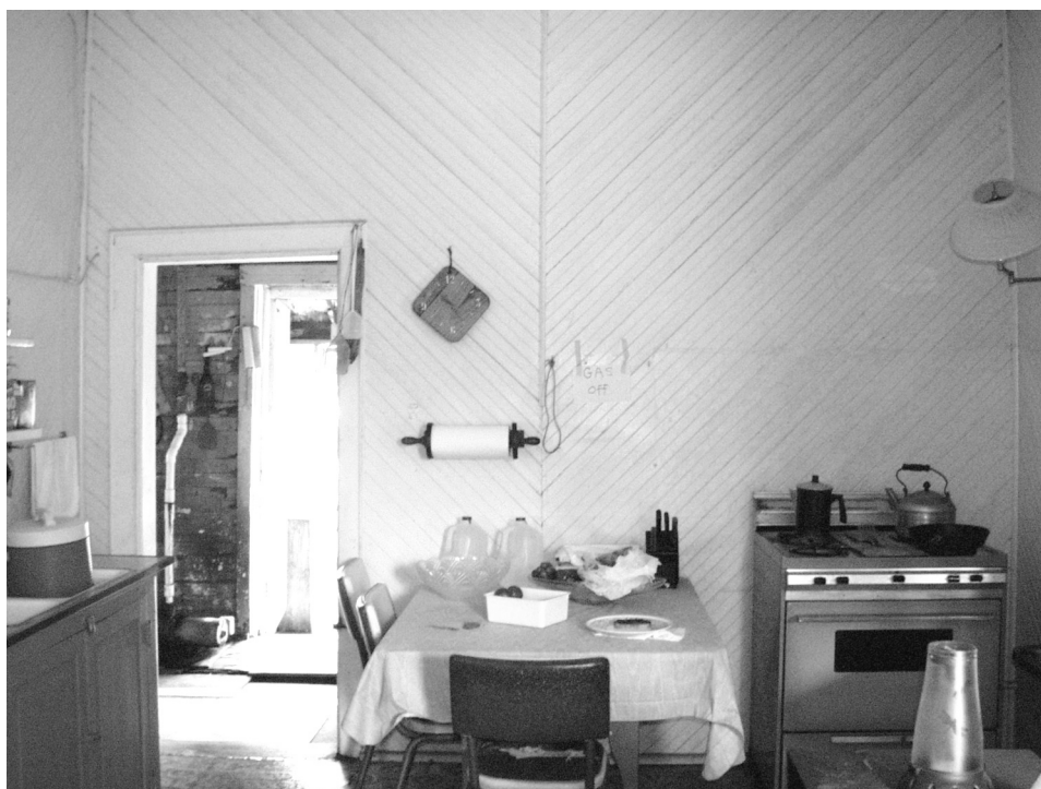
Figure 66 View to east in Room 101, showing original door opening to Room 106 and typical diagonally-laid paneling added in the early twentieth century. (NPS-SERO-CR, 2002)
