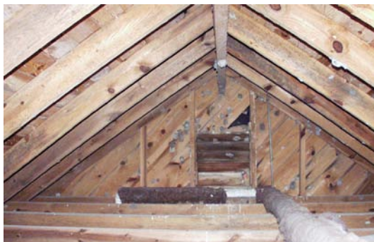
Figure 7 View southeast in attic. (NPS-SERO-CR, 2002)
