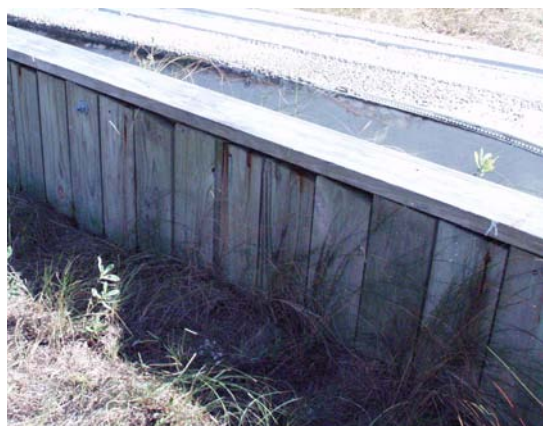
Figure 2 View of flood wall surrounding house. (NPS-SERO-CR, 2002)
