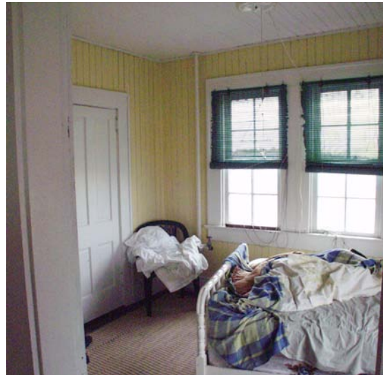
Figure 31 View south in Room 201. (NPS-SERO-CR, 2002)
