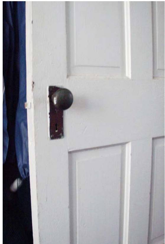
Figure 21 Detail of closet door in Room 101. (NPS-SERO-CR, 2002)
