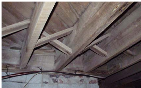
Figure 6 View of typical floor framing. (NPS-SERO-CR, 2002)
