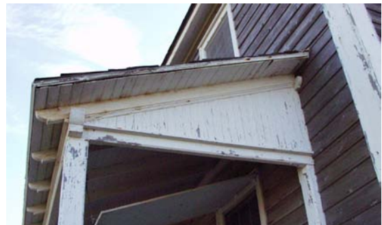
Figure 12 View of west end of front porch. (NPS-SERO-CR, 2002)
