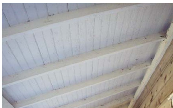
Figure 16 View east of front porch ceiling. (NPS-SERO-CR, 2002)
