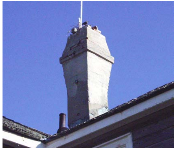
Figure 4 View of chimney. (NPS-SERO-CR, 2002)
