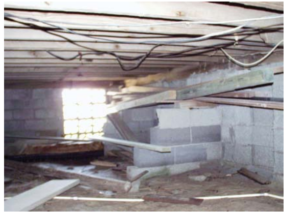
Figure 3 View north in crawl space, showing lattice block used to allow floodwater to pass through the building. (NPS-SERO-CR, 2002)
