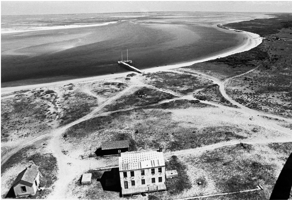
Figure 13 View from lighthouse to the north in June 1973. The summer kitchen is at lower left and the 1873 house is at lower center with the coal and wood shed behind. (CALO Coll. D-25)
