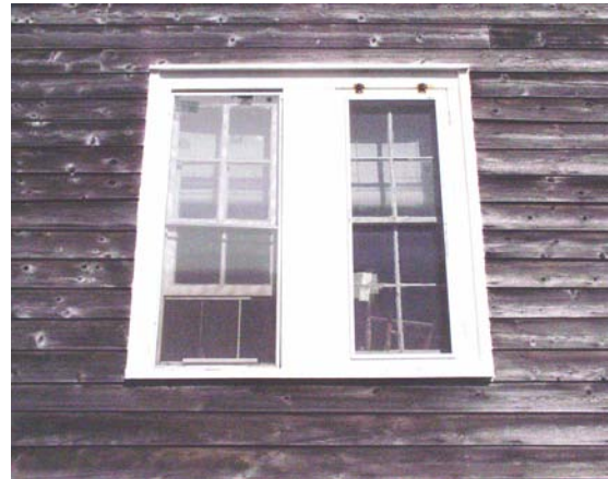
Figure 9 View of typical double windows. (NPS-SERO-CR, 2002)
