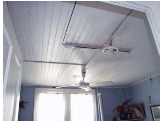
Figure 24 View of ceiling in Room 102. (NPS-SERO-CR, 2002)
