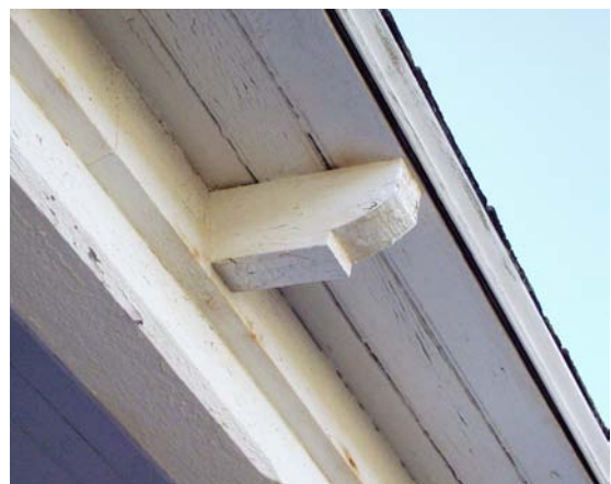
Figure 13 View of front porch eave bracket. (NPS-SERO-CR, 2002)
