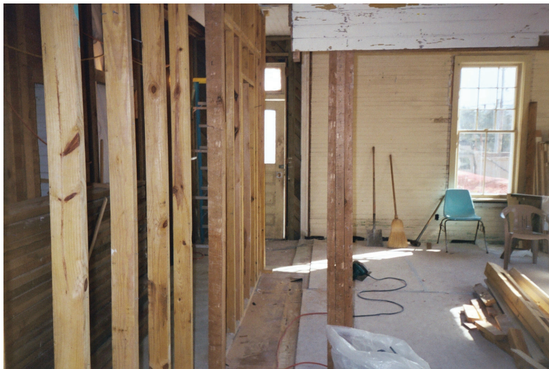
Hatteras Weather Bureau, Photo: National Park Service, 2001
