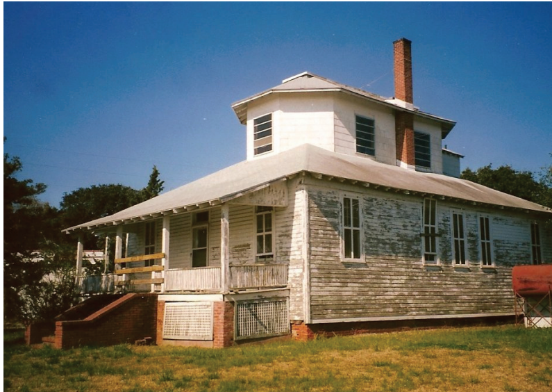
Hatteras Weather Bureau, Photo: National Park Service, 1990
