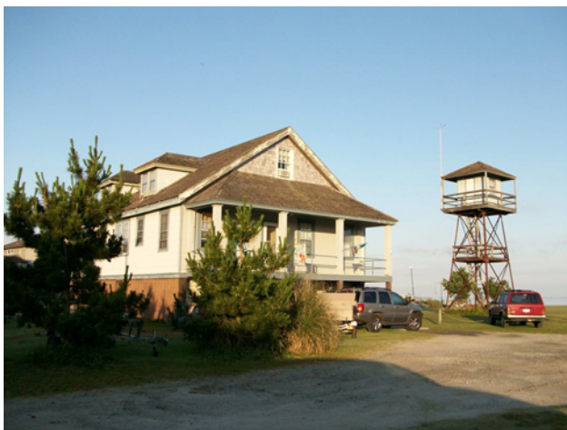
Pea Island Main House and Tower, Salvo, NC. 2008 Photo: Doug Stover
