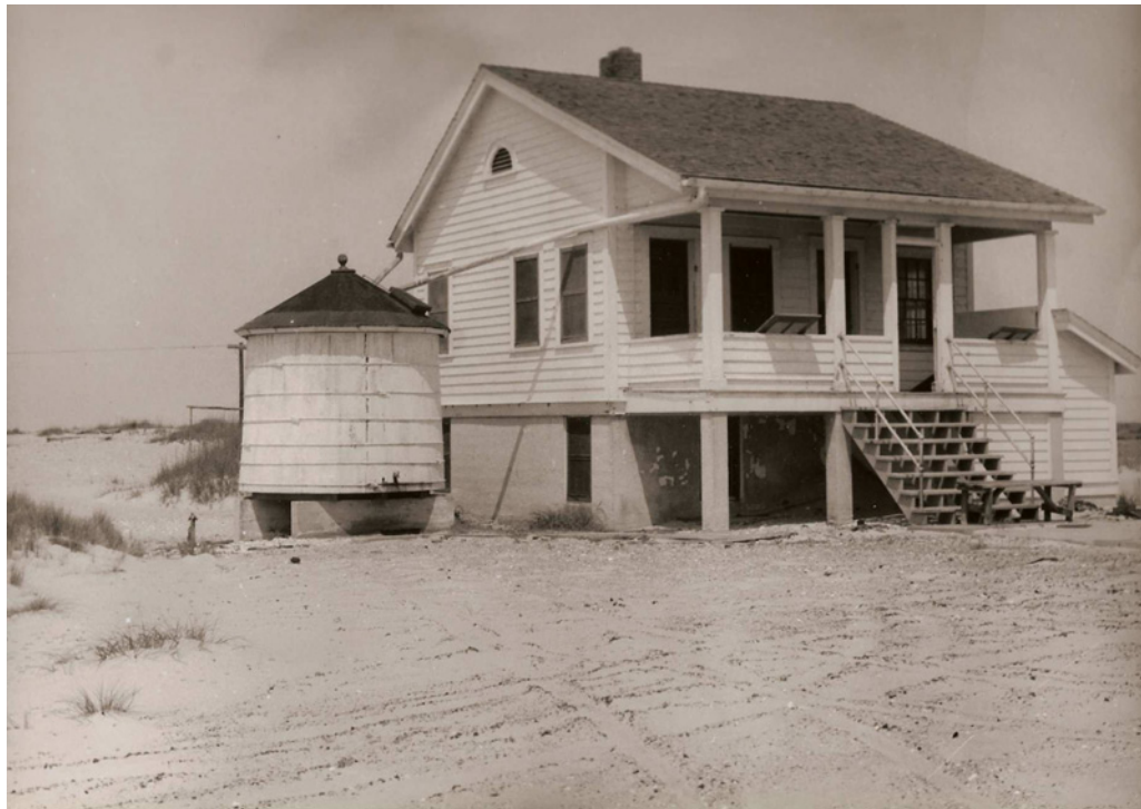
Photo: Pea Island LSS Cookhouse, (1960), Cape Hatteras National Seashore
