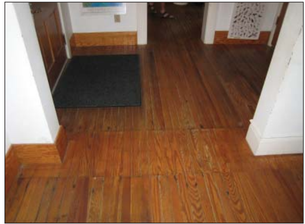
Figure 56, Floor patch at original dividing wall between Room 109 (foreground) and Room 108.
