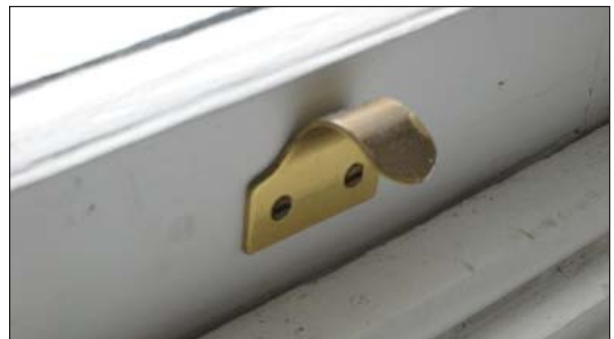
Figure 37, Typical sash lift.
