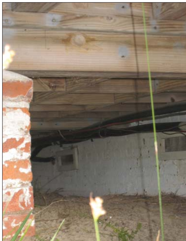
Figure 18, Replacement floor joists at West Porch.
