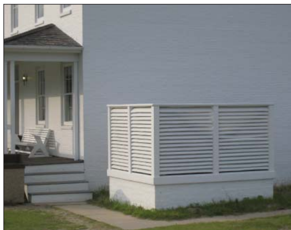
Figure 77, Enclosure for heat pumps.
