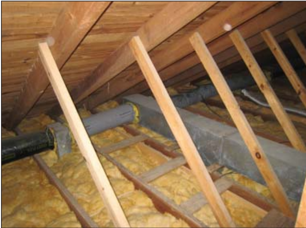
Figure 8, Diagonal bracing added in 1954 in attic to help support new oil heater.
