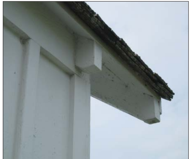
Figure 81 , Exposed rafters, the 1920 Storage Shed.
