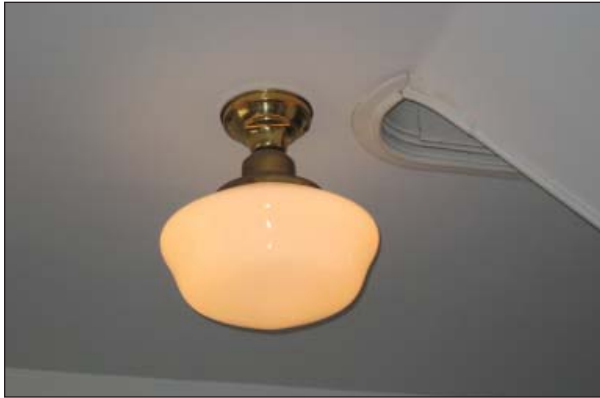
Figure 14, Typical, Interior 12-inch diameter, reproduction "schoolhouse" ceiling light.
