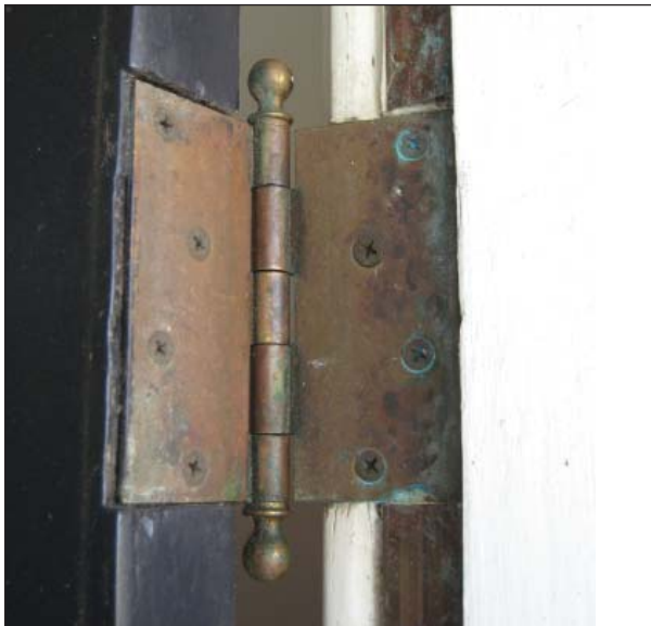
Figure 27, Early brass door hinge, East Porch.
