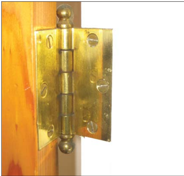
Figure 34, Reproduction ball-pin door hinge.
