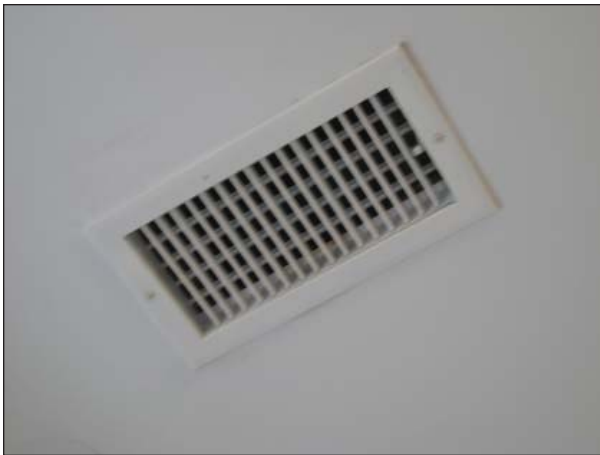
Figure 11 , Typical, 1990s era, 10-inch, metal ceiling register.
