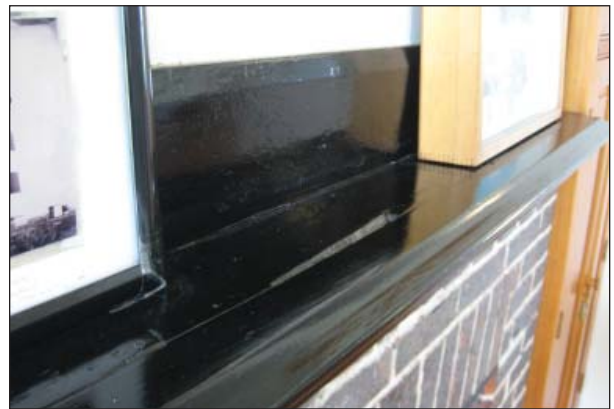
Figure 43, Dutchman repair (1990s) to mantel shelf, Room 101.
