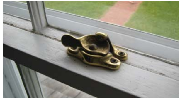
Figure 36, Typical sash latch.
