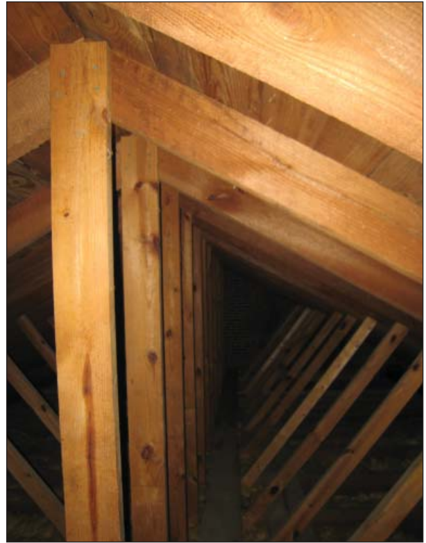
Figure 9, Vertical brace added at unknown date to apparently help support the 1954 oil heater.
