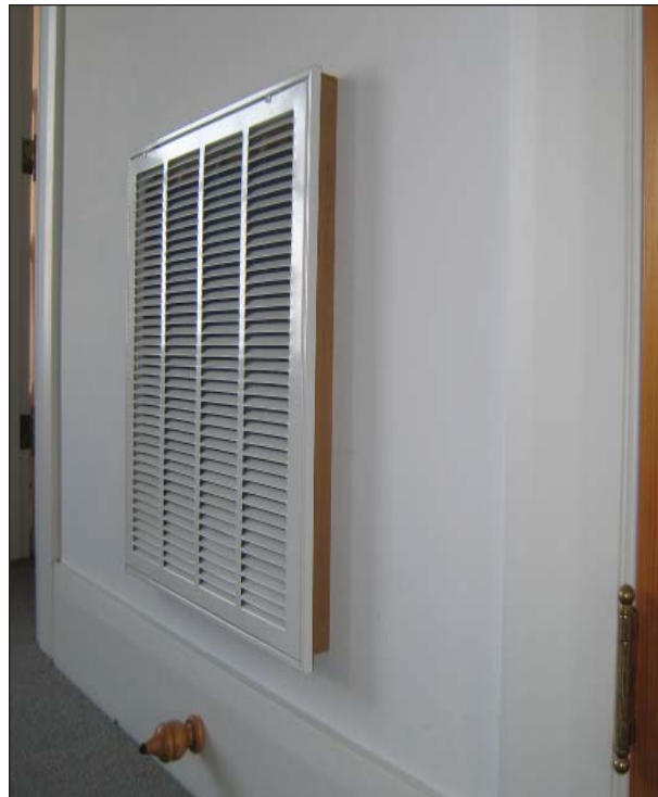
Figure 12 , Typical, 1990s, 1'-10" by 1'-10" metal return grill.
