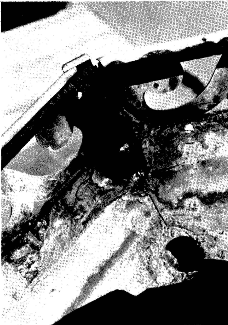
OLD POINT LOMA LIGHTHOUSE, 1977. DETAIL OF BACK OF LANTERN CORNICE. NOTE CONDITION OF CORNICE BRACKETS. National Park Service Photograph, Cabrillo National Monument.
