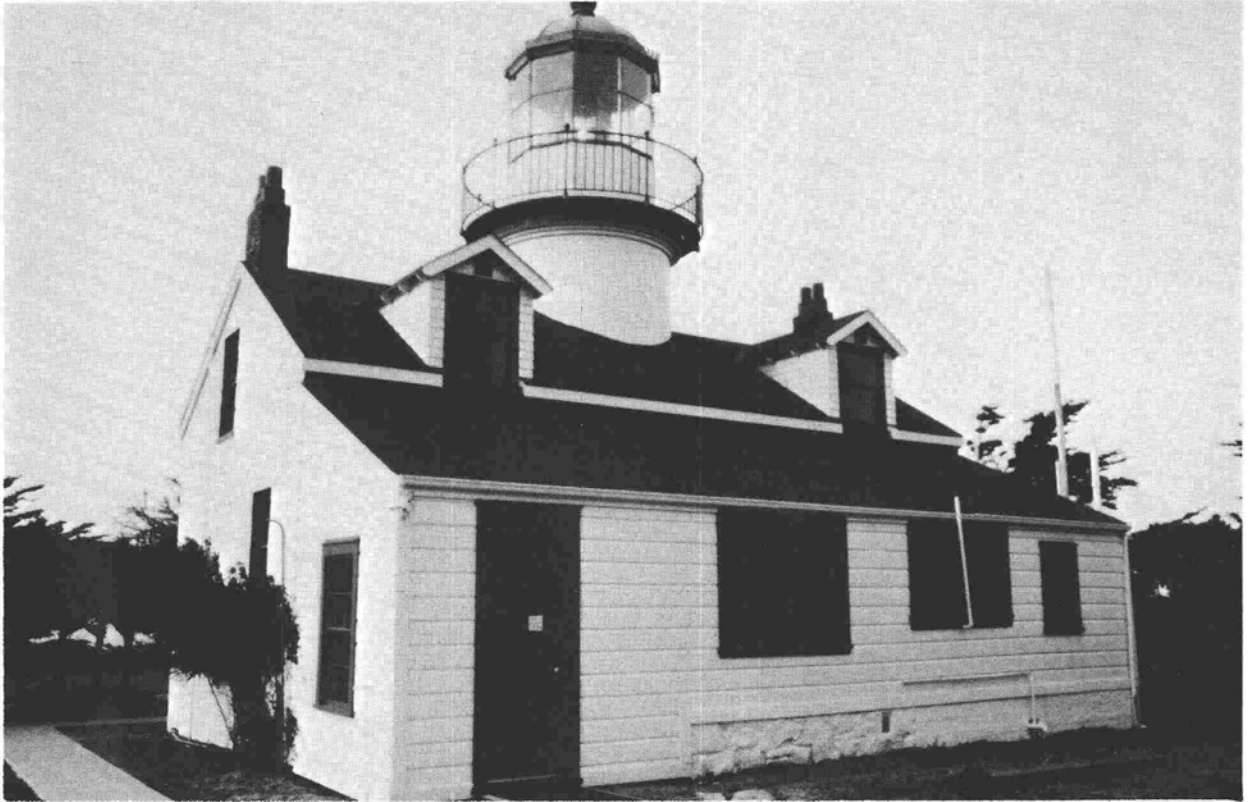
POINT PINOS LIGHTHOUSE, EAST (REAR) ELEVATION, 1979. NOTE STONE FOUNDATION WHERE ORIGINAL LEAN-TO WOULD HAVE BEEN. THE EARLY SHINGLE ROOF OF THE LEAN-TO EXISTS INTACT UNDER THE LARGER EXISTING LEAN-TO ROOF. National Park Service photograph by H. G. Law
