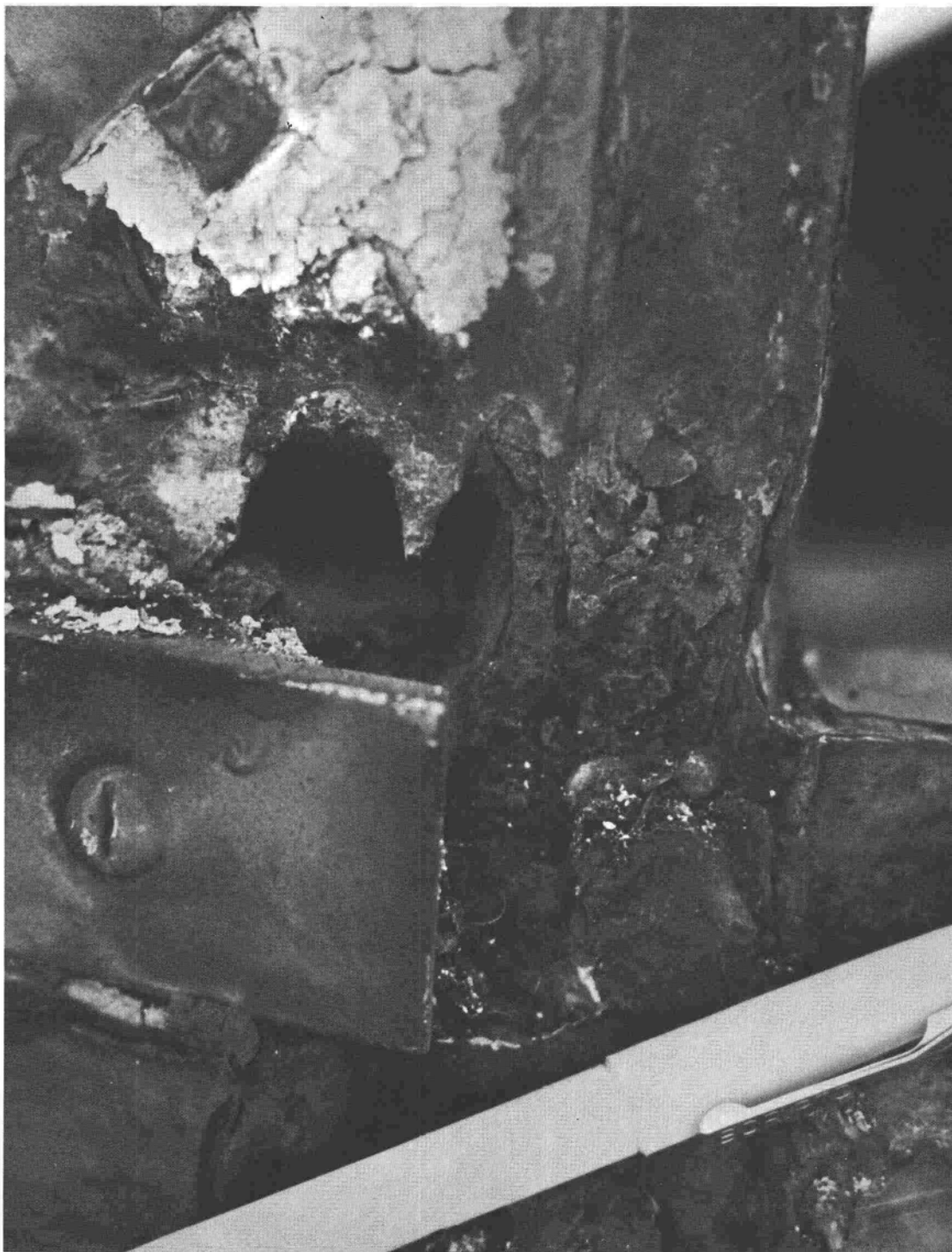
OLD POINT LOMA LIGHTHOUSE, 1977, DETAIL AT BASE OF LANTERN SHOWING DETERIORATED CONDITION OF A PANEL CORNER AND ADJACENT ASTRAGAL. National Park Service photograph Cabrillo National Monument.
