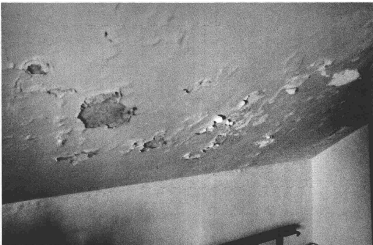
OLD POINT LOMA LIGHTHOUSE, SECOND STORY CEILING OF THE DWELLING, 1979. NOTE DETERIORATED CONDITION OF THE PLASTER. National Park Service photograph by H. G. Law
