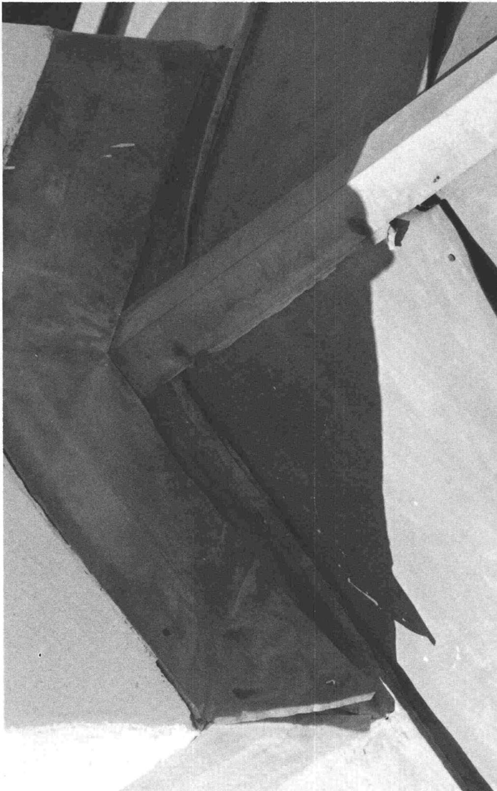
OLD POINT LOMA LIGHTHOUSE, EXISTING FLASHING DETAIL ON ONE OF THE CHIMNEYS, 1977. NOTE THE CONDITION OF THE ROOFING. National Park Service photograph by H. G. Law
