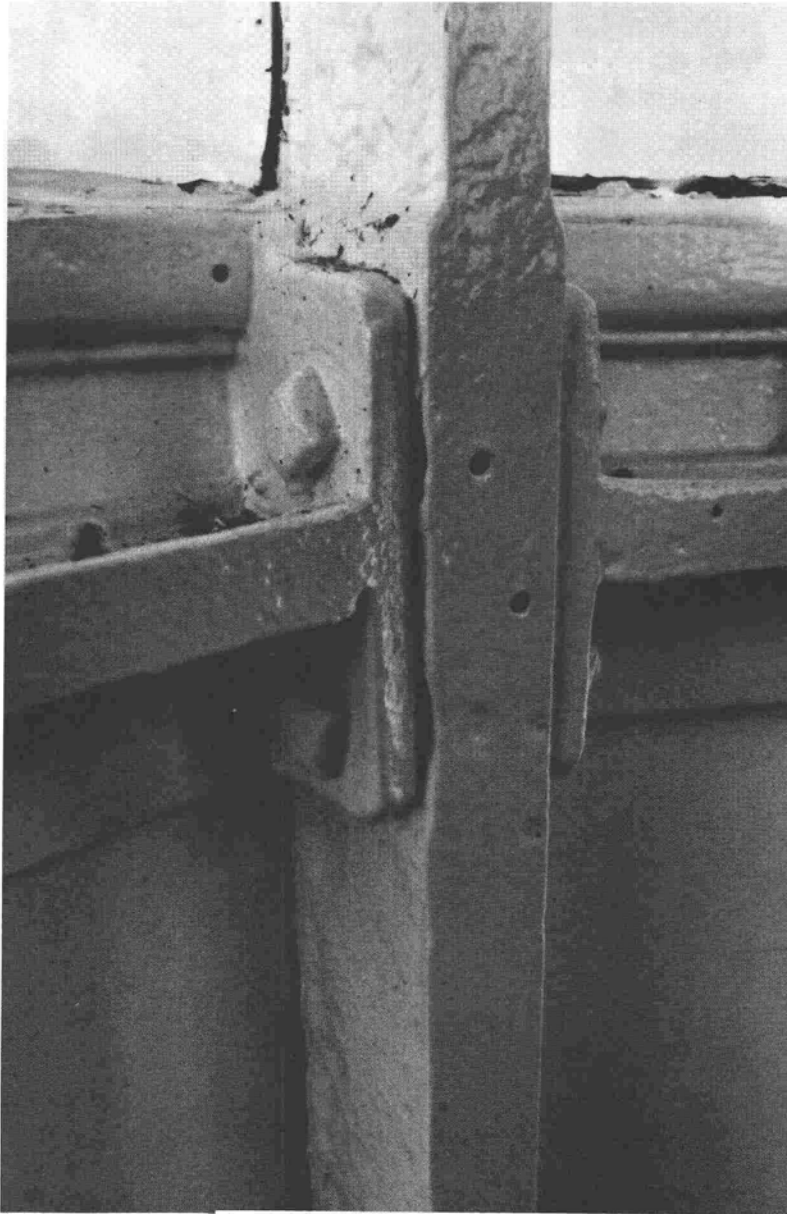
OLD POINT LOMA LIGHTHOUSE, 1979. TYPICAL DETAIL OF WINDOW SILL/ GUTTER CONNECTED TO THE VERTICAL ASTRAGAL. NOTE THE GAPS LEFT FROM PIT CORROSION. THESE GAPS ARE IDEAL FOR THE CREATION OF MORE PIT CORROSION. National Park Service photograph by H. G. Law
