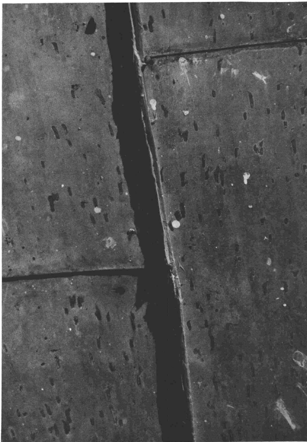
OLD POINT LOMA LIGHTHOUSE, DETAIL OF STANDING SEAM ON THE EXISTING COPPER ROOF, 1977. NOTE CAULKING IN CRACKED SEAM National Park Service photograph by H. G. Law
