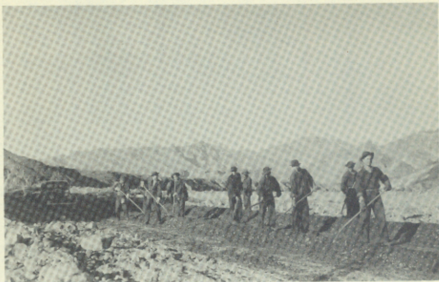
ROADS ARE EASILY BUILT AND SCARIFIED
