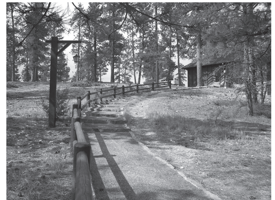
Photograph A/18. The existing path to the side entry to the Male Dormitory.
