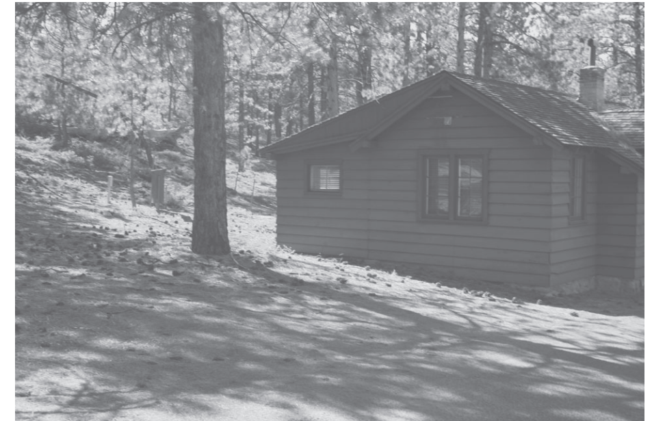
Photograph A/1. Small scale parking area near one of the historic cabins in the Old NPS Housing Study Area.
