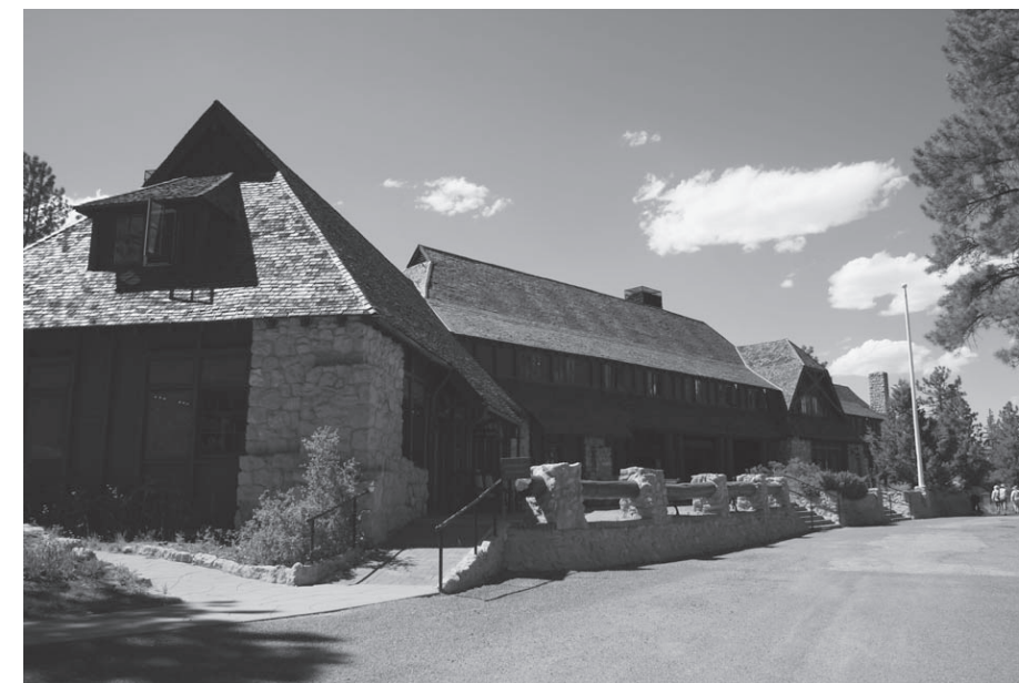
Photograph A/16. The front of the Lodge today from a similar angle with the prominent trees missing.
