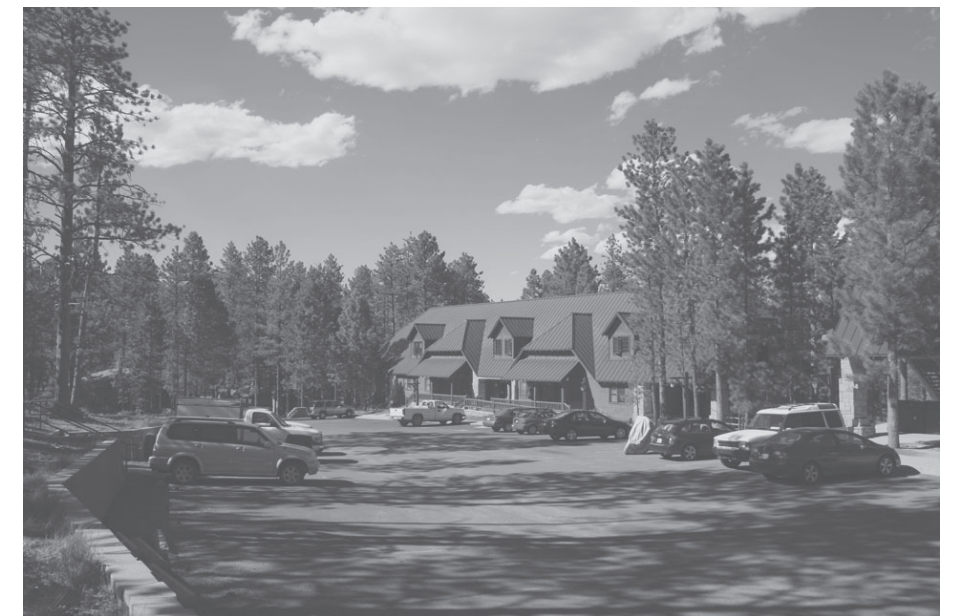
Photograph A/2. The large scale parking area in front of the new Concessionaire Dormitories in the Old NPS Housing Study Area.
