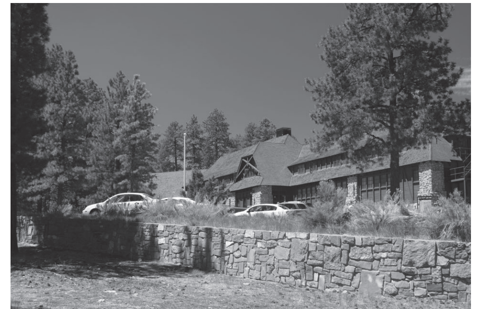
Photograph A/9. The retaining wall between the Lodge and the Sunrise Motel Unit which creates the space for the Registration Parking Area.
