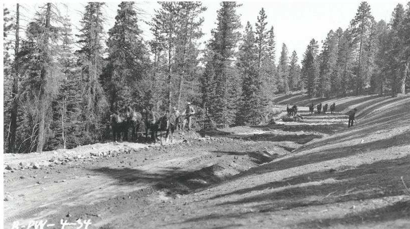
Photograph 21. Rough grading, Bryce Rim Road ; PWA project under B.P.R. supervision (BRCA Archives: ACC#350 Photo#1)
