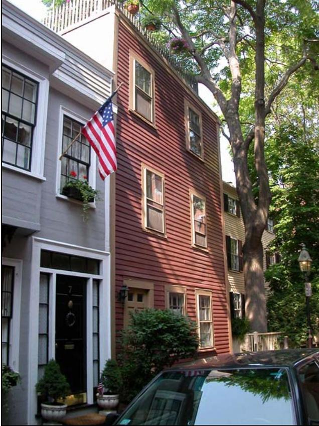
5 Smith Court is a three-story, two-bay vernacular Federal clapboard structure constructed circa 1825-35. Wood planks surround the 6/6-light windows. There is a one-step run to the sidehall entry on the façade. Narrow cornerboards edge the building. The upper stories of the façade have two bays, while the first story is three bays. The east elevation is three bays with a door entry on the first story. The roof of the building is not gabled but has a slight pitch toward the façade.
