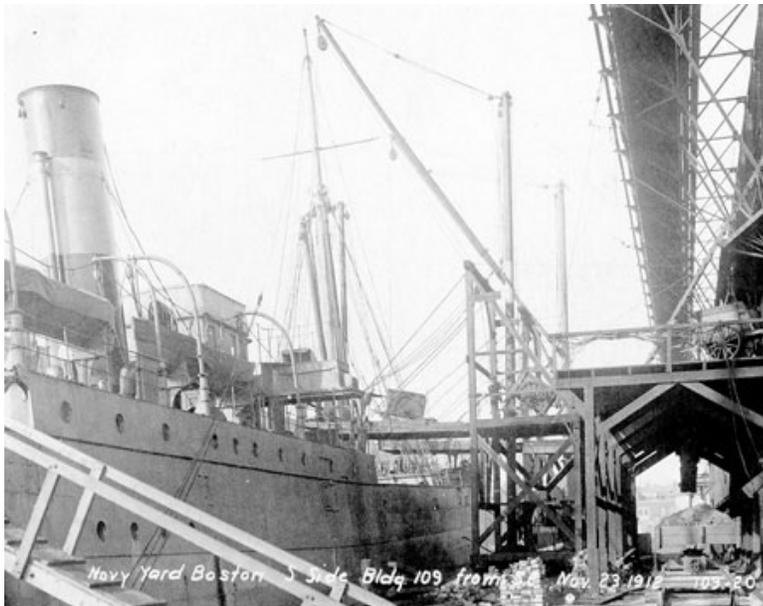
**Figure 5.20: 1912 view of the Coaling Plant (Building 109) in operation with a rail line and one of the yard's thirteen dump cars for coal in the foreground (BOSTS-9807,9808).**
