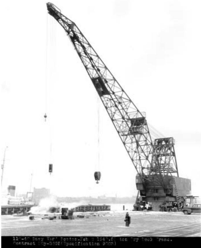
**Figure 6.4: A portal crane in 1940 (BOSTS-15673).**
