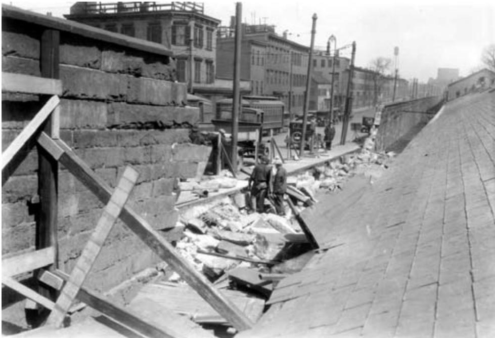
**Figure 5.48: Removal of the rubble-filled granite boundary wall between the Ropewalk (Building 58) and Chelsea Street in 1929 (BOSTS-8951).**
