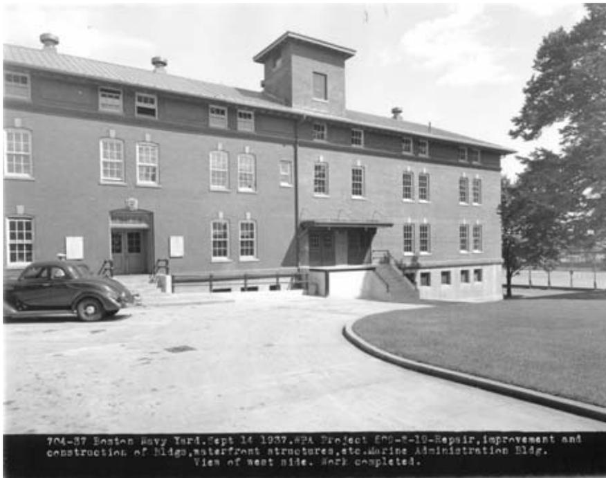
Figure 6.12: The Marine Corps Administration Building (Building 136) in 1937 after being enlarged to the south by the WPA (BOSTS-9883).
