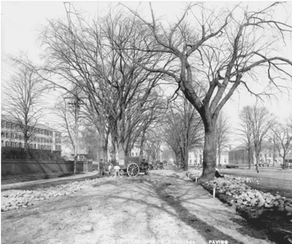
**Figure 5.1: Second Avenue repaving project in 1904. Quiet woodblocks paved the street with cobblestone side gutters. Note the mature elm trees lining the road (BOSTS-8656).**
