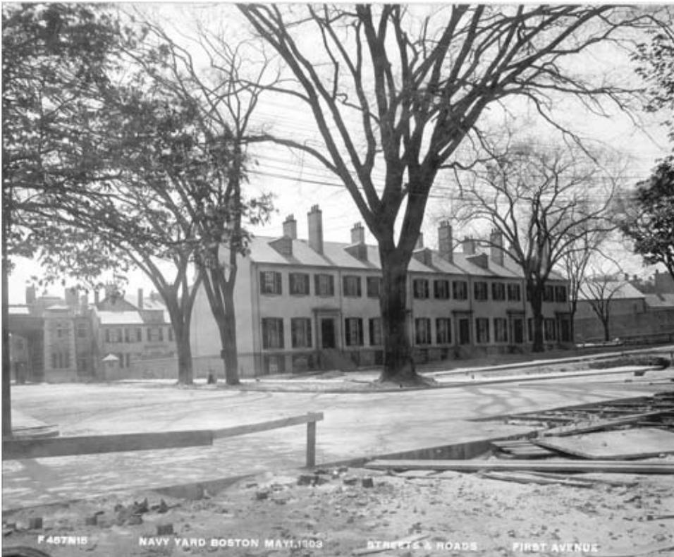
**Figure 5.2: Paving of First Avenue by the Officer's Quarters (Building 265) in 1903. Note the mature elm trees and the Main Gate (Building 97) on the left (BOSTS-9168).**
