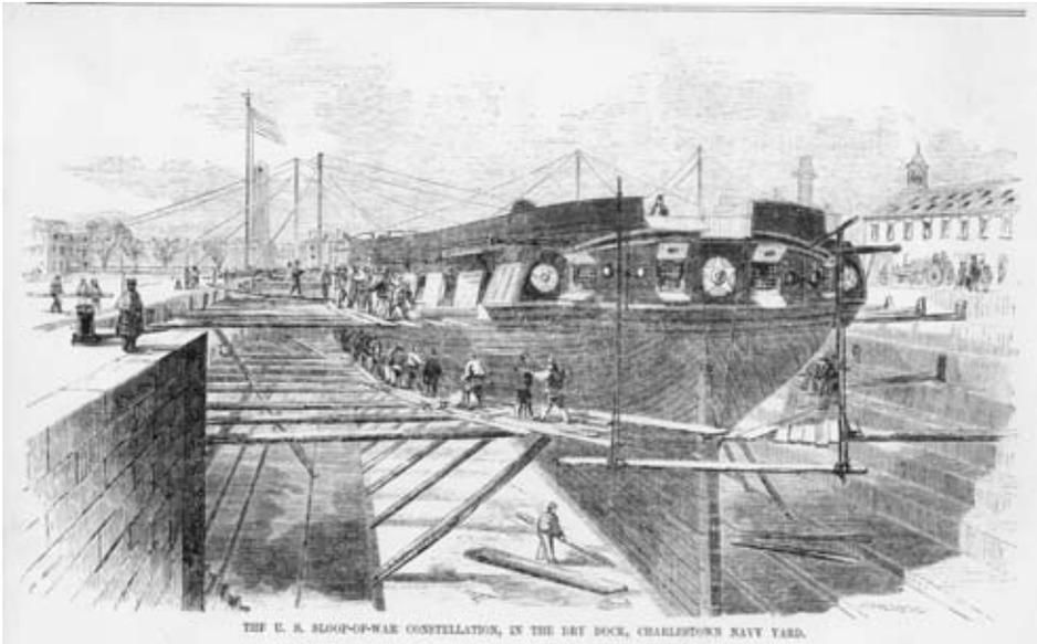
**Figure 3.5: Engraving from c. 1859 of Dry Dock 1, which was completed in 1833. Staging installed in the dry dock allowed workers to work on the hull of USS *Constellation* at two levels from Gleason’s *Pictorial Drawing-Room Companion* (BOSTS 10721).**
