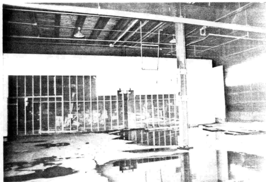
Illustration 28. Stud partition with wire mesh and particle board between Rooms 102 and 104. Taken from Room 104. Garage door at right, Room 103 at left.
