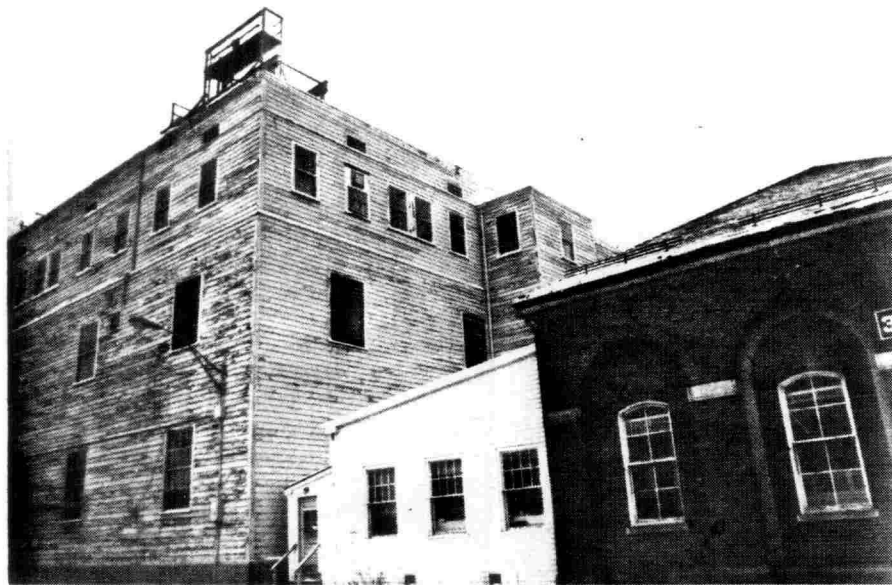
Illustration 13. Southeast corner showing missing sash at second floor, structure on roof for lights, relationship to adjacent Building 32. Note also one added vent replacing a window sash at the third-floor level.
