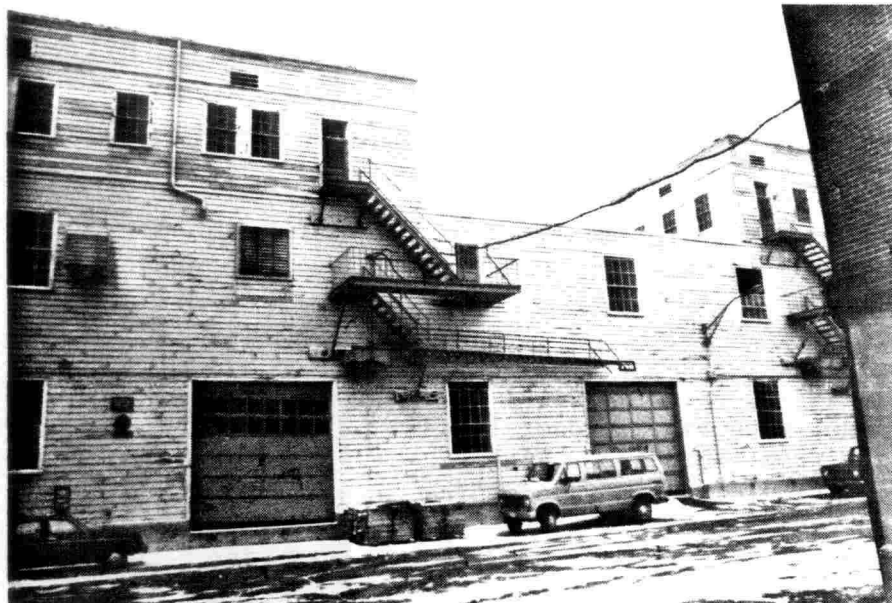
Illustration 4. The eastern fire escape on the north facade. The door on the second-floor opening onto the fire escape was an eight/eight light window before the third floor and fire escape were added. Vents on the second floor were added where and when needed.
