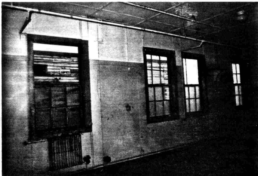
Illustration 52. Room 328 - Low partitions have been removed - some sash missing.
