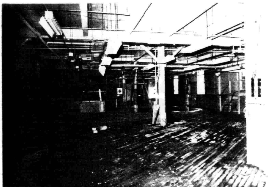
Illustration 38. Room 201 looking west. Note northern windows, stair access to fire escape door, diagonal floorboards, exposed framing ceiling, and flourescent lights.
