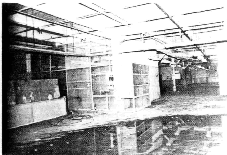
Illustration 37. Room 201 looking west at caged area. Note the standing water on the diagonal floor boards. Also note the exposed framing ceiling.
