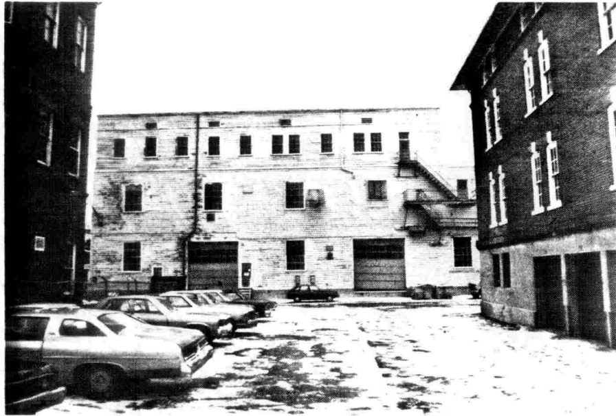
Illustration 7. North facade eastern half. Note the small window and door at the first-floor level. These are later additions. Building 136 is on the right, the Muster House is on the left.
