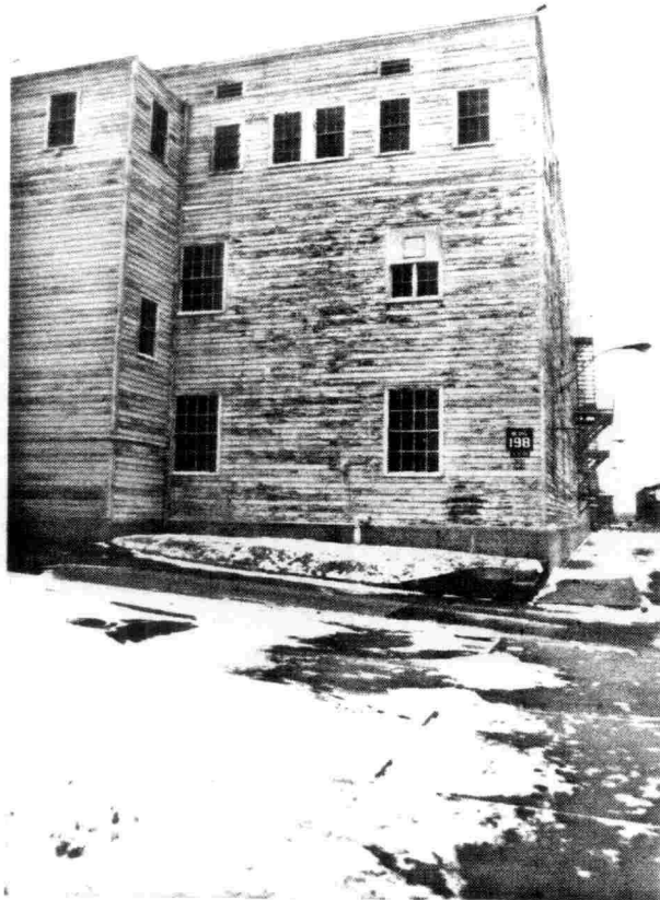
Illustration 19. West facade, southern portion. Note the difference in heights of the main building and the stair tower. Also note the vent and replaced sash in one window on the second floor.
