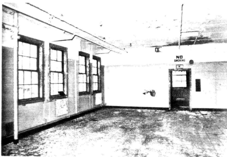
Illustration 56. Room 347 - low partitions removed. Door leads to Room 348. Windows fairly intact, preventing severe water damage.
