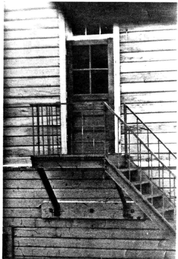
Illustration 6. Typical four light wood paneled door leading from third-floor eastern addition to north facade fire escape.
