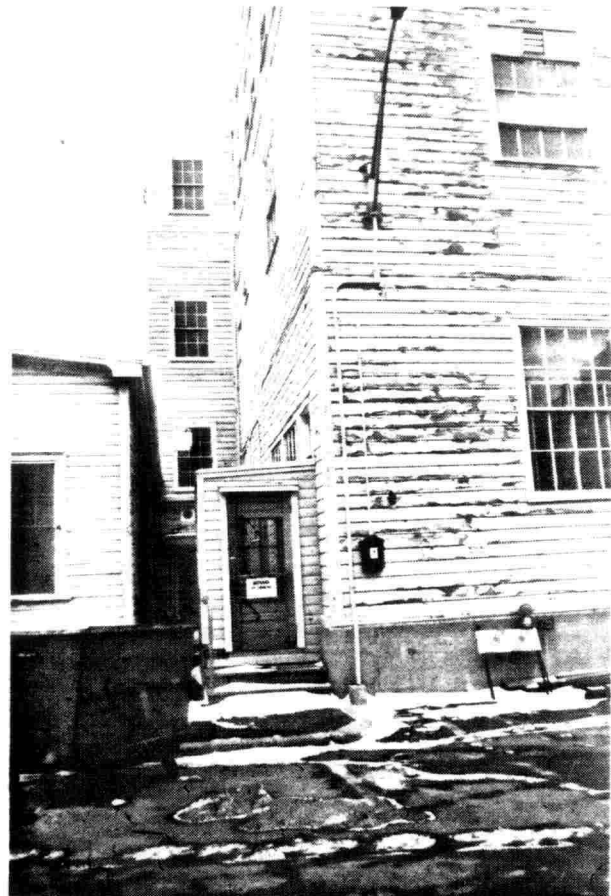
Illustration 7. North facade eastern half. Note the small window and door at the first-floor level. These are later additions. Building 136 is on the right, the Muster House is on the left.
