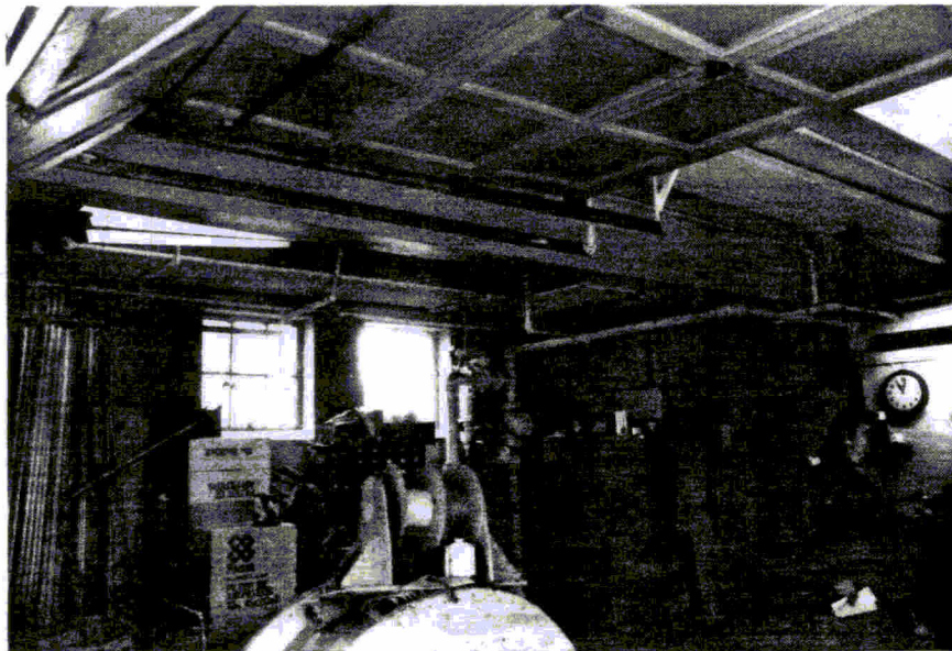
30. Room 009 - note sliding garage door overhead. Also concrete and steel framing system on ceiling.
