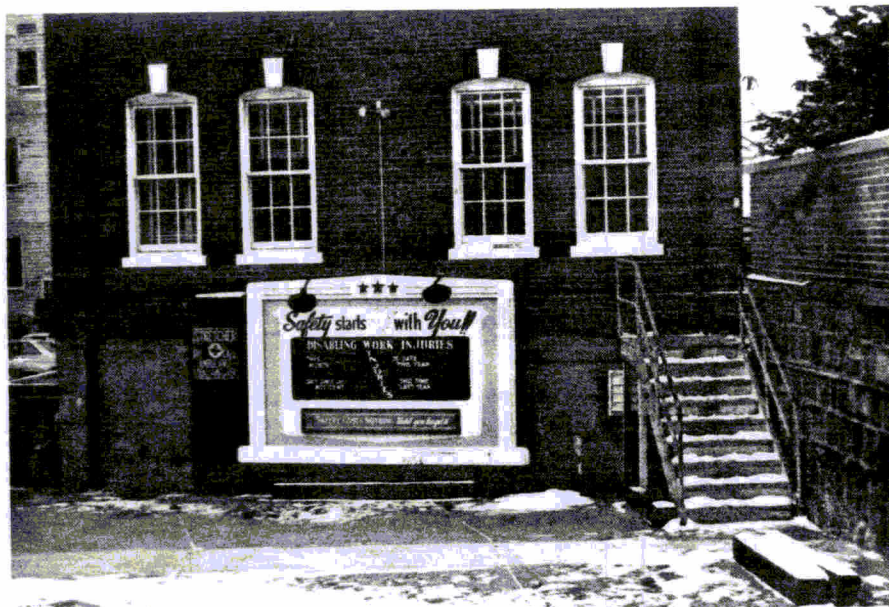
24. North facade - note vent under stairs on right is location of original window. Remaining three windows at basement level blocked-in.
