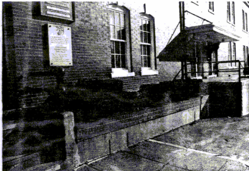
16. West facade, entrance to southern addition on right, entrance to original structure on left. New planter build over former areaway. Original window sash.
