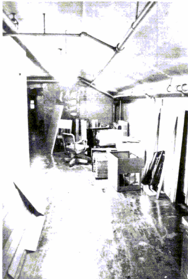
55. Room 304 looking north next to Room 112. Note the ceiling configuration conforming to the rafters and collar beams.
