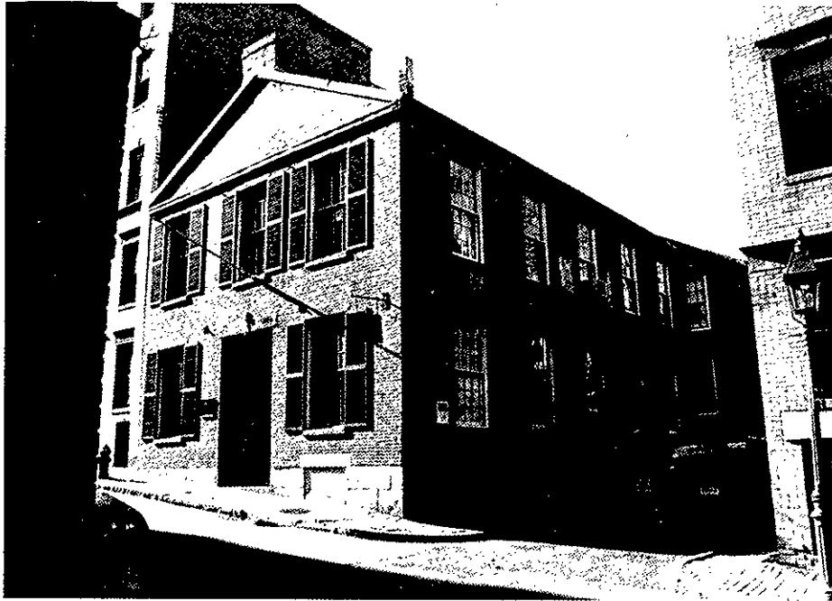
Figure 24. Smith School House: East (front) and north elevations (1990).
