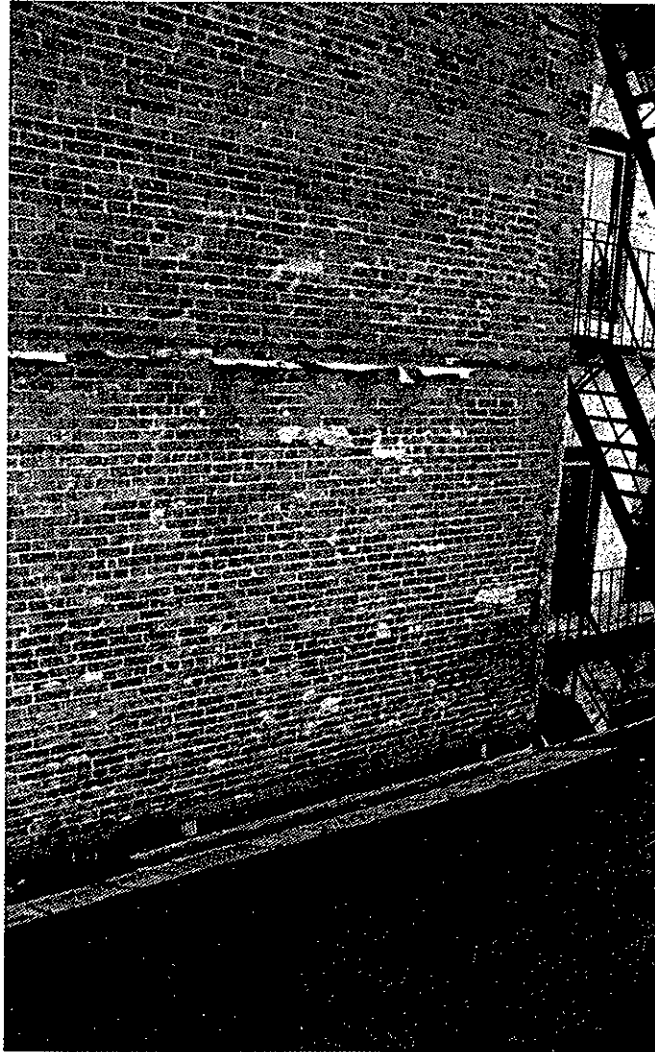
Figure 34. Smith School House: Junction of roof with adjacent south building, showing flashing line remaining from circa-1910 roof alteration (1990).
