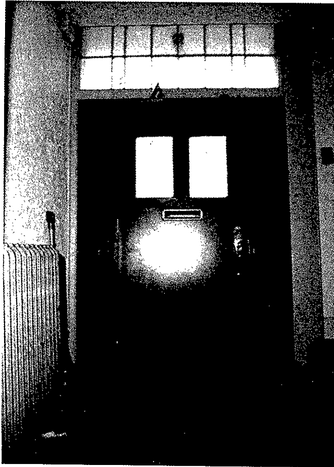
Figure 50. Smith School House: First-story entry, looking east (1990).
