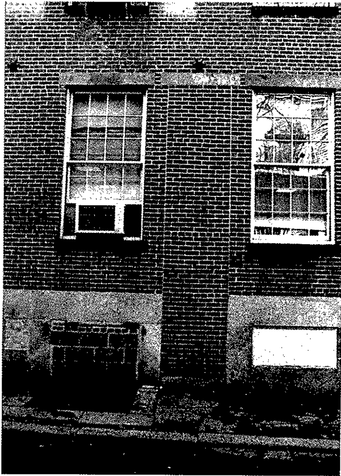
Figure 28. Smith School House: North elevation, infill of two former doorways (1990).
