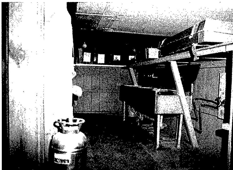
Figure 38. Smith School House: Cellar, meeting room, area behind west counter (1990).
