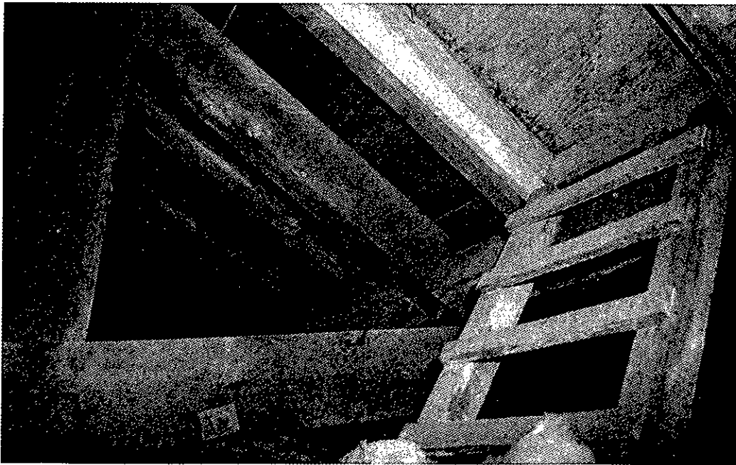
Figure 77. Smith School House: Attic, looking southeast at roof hatch (1990).
