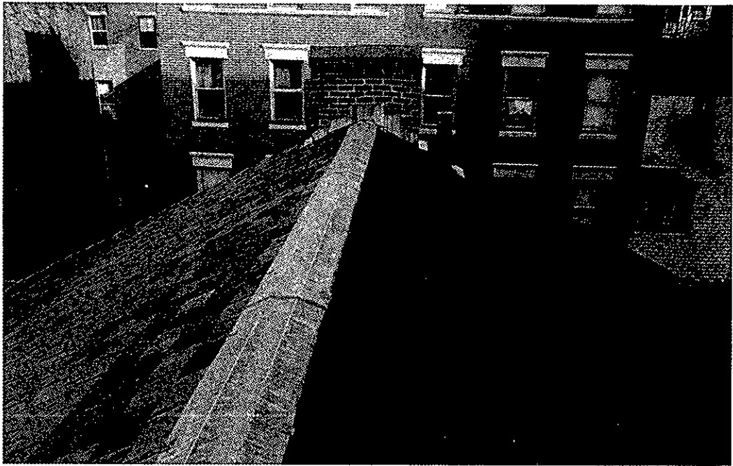
Figure 32. Smith School House: Roof, looking east (1990).
