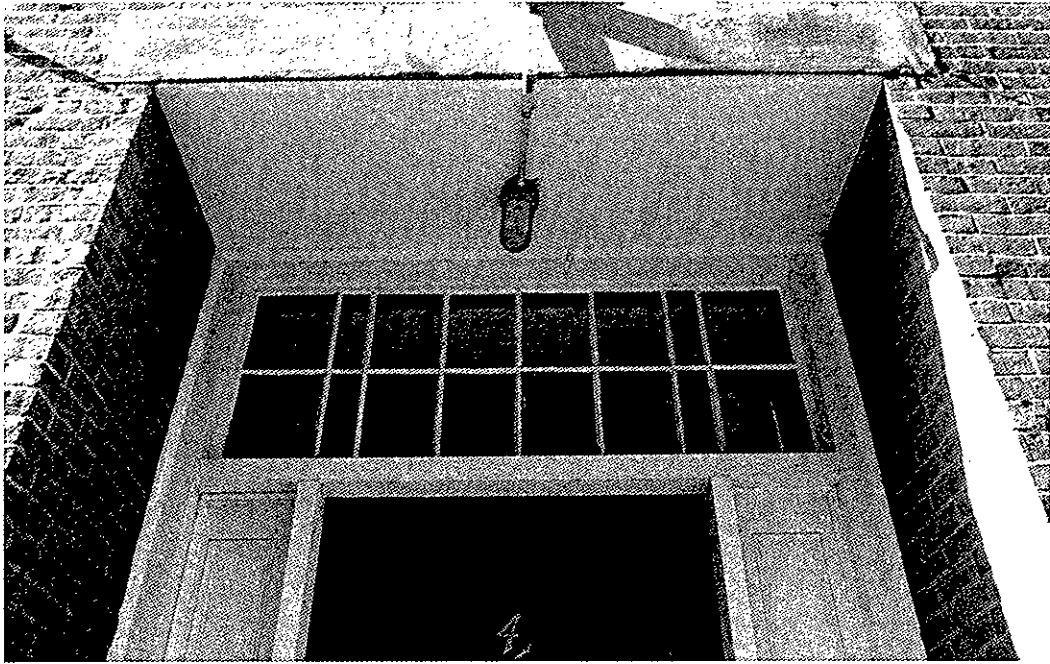
Figure 26. Smith School House: East elevation, doorway transom (1990).
