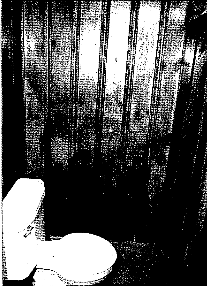
Figure 46. Smith School House: Cellar, men's toilet enclosure (1990).
