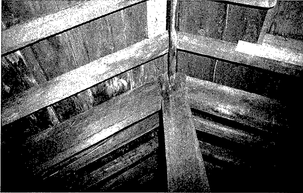
Figure 76. Smith School House: Attic, looking up at the ridge board (1990).
