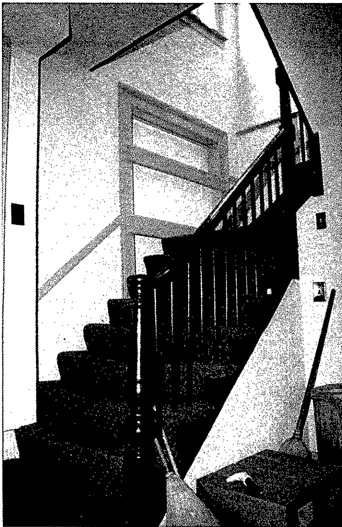
Figure 53. Smith School House: First-story entry, stairway to the second story (1990).
