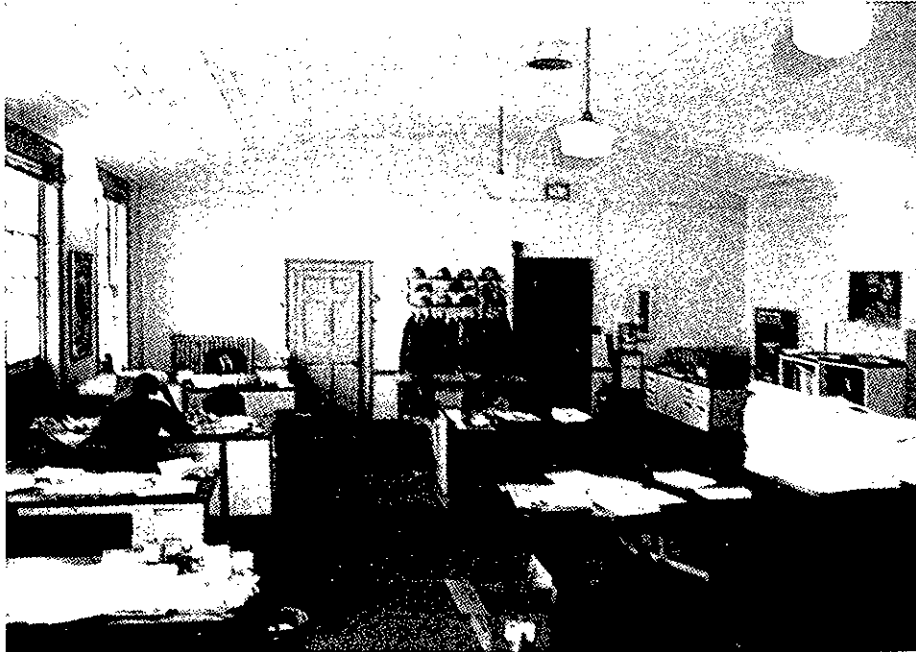
Figure 63. Smith School House: Second story, NPS office, looking east (1990).
