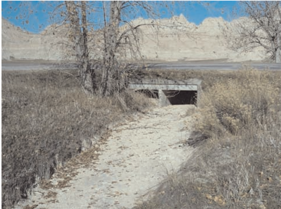
Figure 3-99: (C-10) Concrete box culvert.
