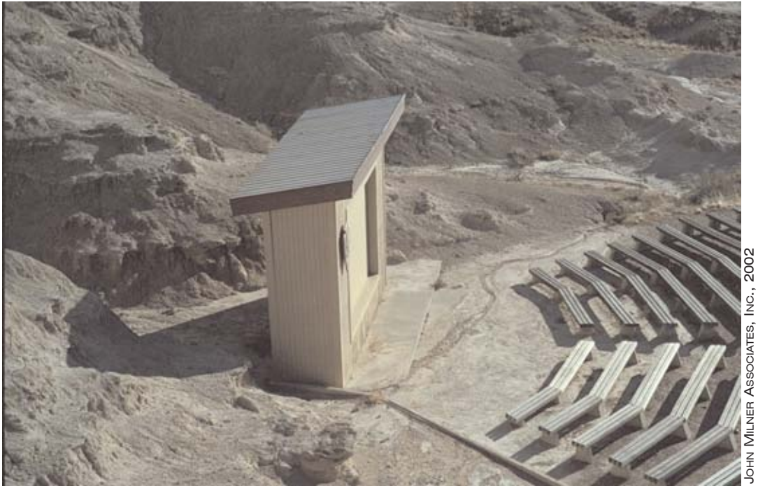
Figure 4-17 View of amphitheater screen, wood benches on concrete supports, and concrete retaining wall along the perimeter in 2002.
