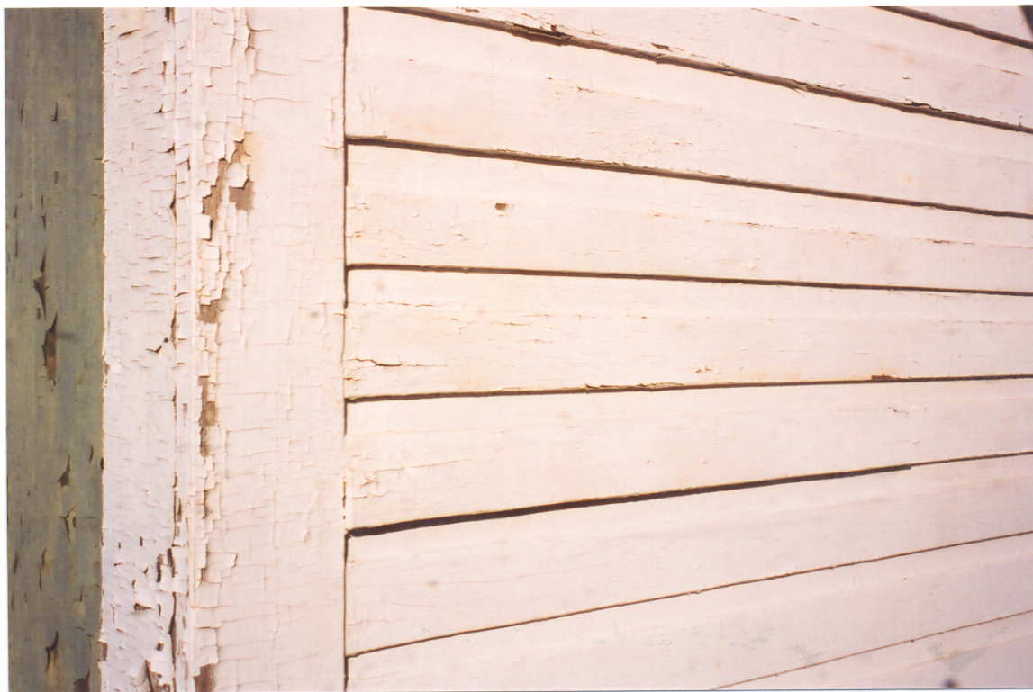
Figure 80. Garage: North elevation, detail of novelty siding (1999).
