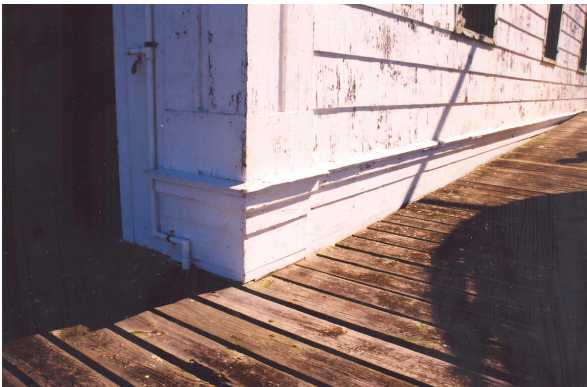
Figure 101. Boathouse: Northwest corner, water table detail (1999).
