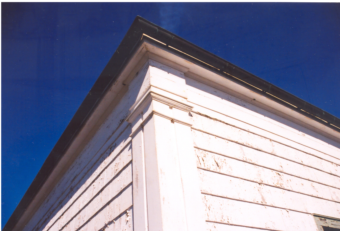
Figure 100. Boathouse: Southeast corner, architrave and pilaster detail (1999).
