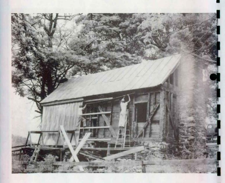
Completed Stabilization Work on Up-Hill Elevation, "Sweeney Prizery," June 16, 1959.
