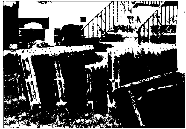
FIGURE 41. Two of seven historic cast iron radiators were permanently removed from the Cemetery Lodge to increase interior space.
