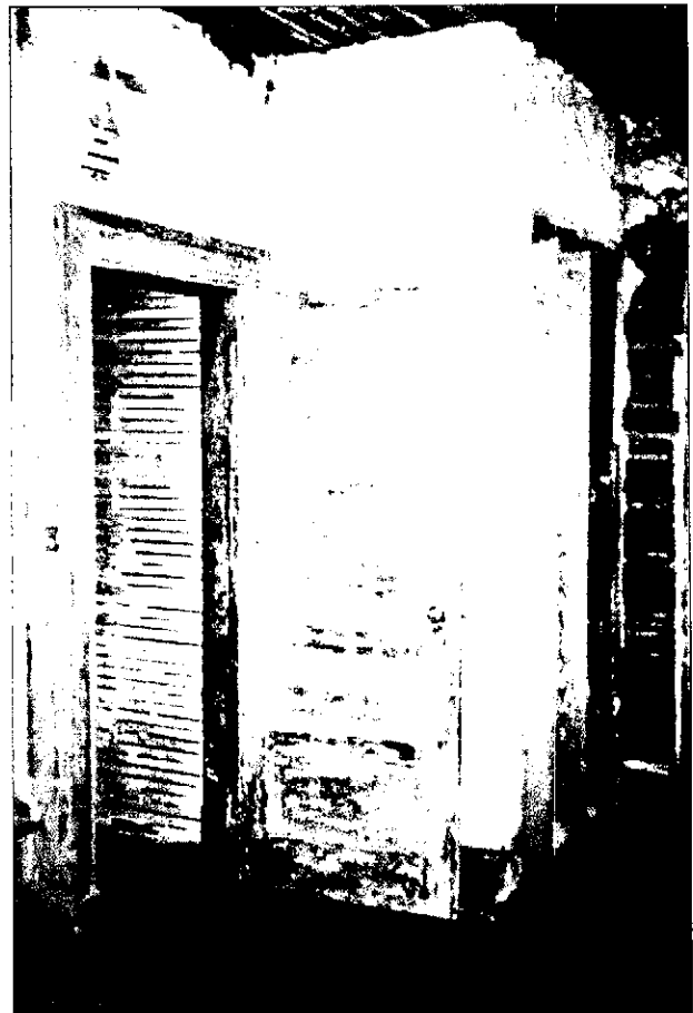
FIGURE 39. Woodwork was stripped of paint and deteriorated plaster removed.
