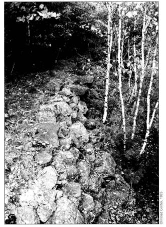
Fig. 81 The Gurnee Path, between Bar Harbor and Hulls Cove, was funded by Augustus Gurnee and endowed with a maintenance fund by his three daughters. Completed in 1926, path construction included extensive retaining walls and rubble fill to create a level walking tread. A wooden railing and benches were placed along a high ledge overlooking Frenchman Bay. The path is no longer marked but easy to follow.
