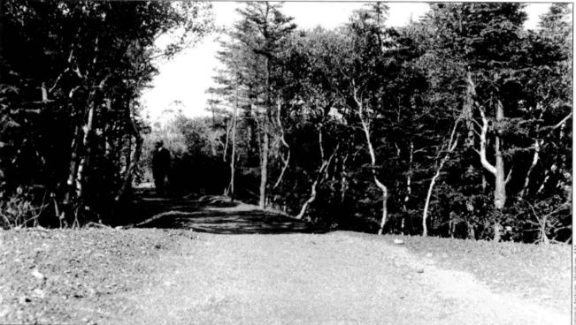
Figs. 100, 101 CCC photographs from circa 1937. The upper photograph shows the trail surface after it has been "swamped out," plants and roots removed, and the rough grade set with stone rubble. The lower image shows the path after it has been surfaced with screened gravel.
