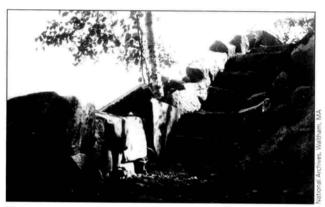
Fig. 115 A circa-1934 photograph of the Perpendicular Trail illustrating the large stone used for steps and coping to prevent heaving by ice and frost. The steps and coping are still in good condition.
