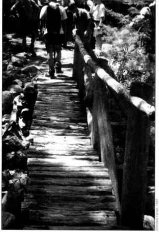
Figs. 133, 134 NPS Crew Leader Gary Stellpflug rebuilt the footbridge at the northern end of Jordan Pond in 1983 (above). He duplicated the previous design for the bridge using 2-inch instead of 1-inch planking and larger cedar logs. Stellpflug and the trails crew also rebuilt the footbridge on the Great [Long]Pond Trail (lower photograph) using Appalachian Mountain Club specifications for footbridges. Stellpflug recalled that the preexisting CCC bridge was wide enough for a fire vehicle.
