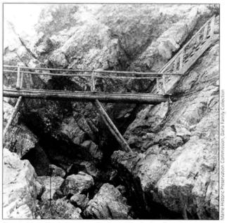
Fig. 64 Circa-1908 photograph of a bridge built of cut boards and rough-hewn logs along the rocks near Seal Harbor.
