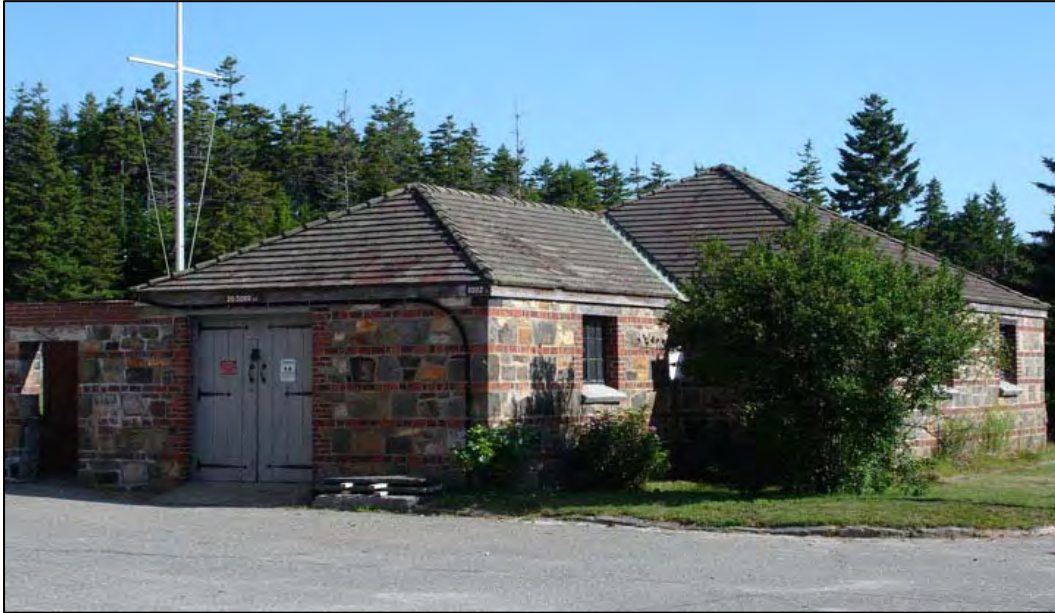
Figure 71. Power House adjacent to the Apartment Building, SW and SE elevations looking north, 2008.
