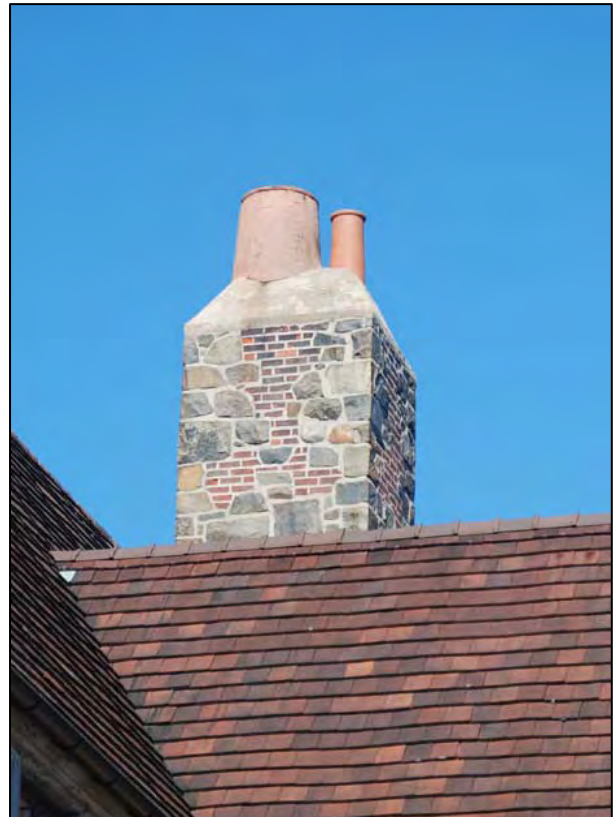
Figure 55. Apartment Building, SW chimney, 2008.
