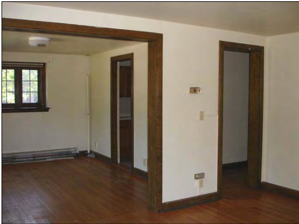
Figure 67. Apartment Building typical apartment interior elements, Apartment No. 9 looking NE from Living Room to Dining Room, 2008.
