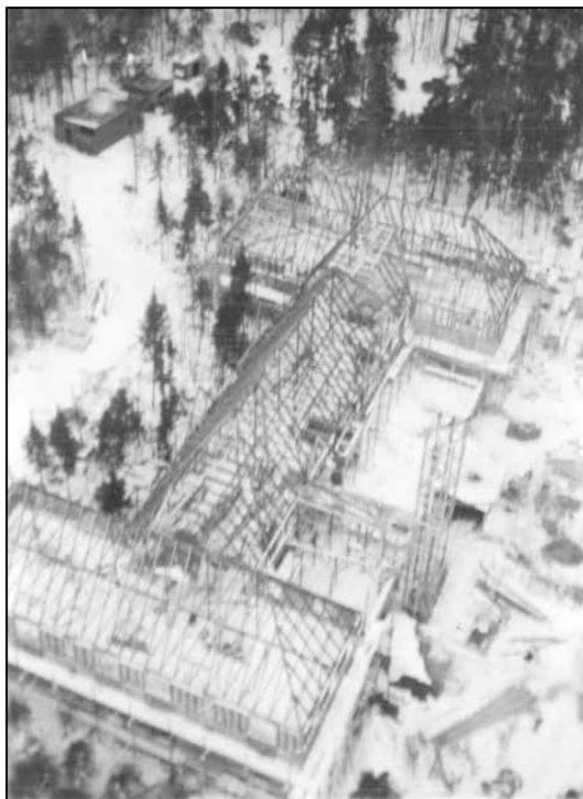
Figure 29. Apartment Building roof framing, view from SW tower.
