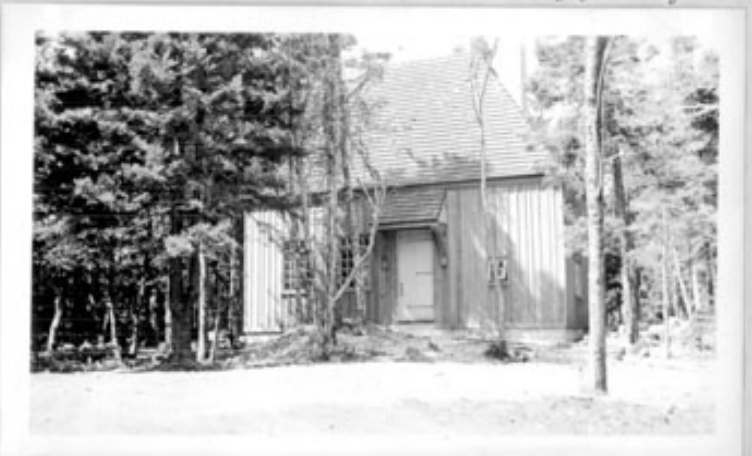
Intercept Bldg from S. E.
