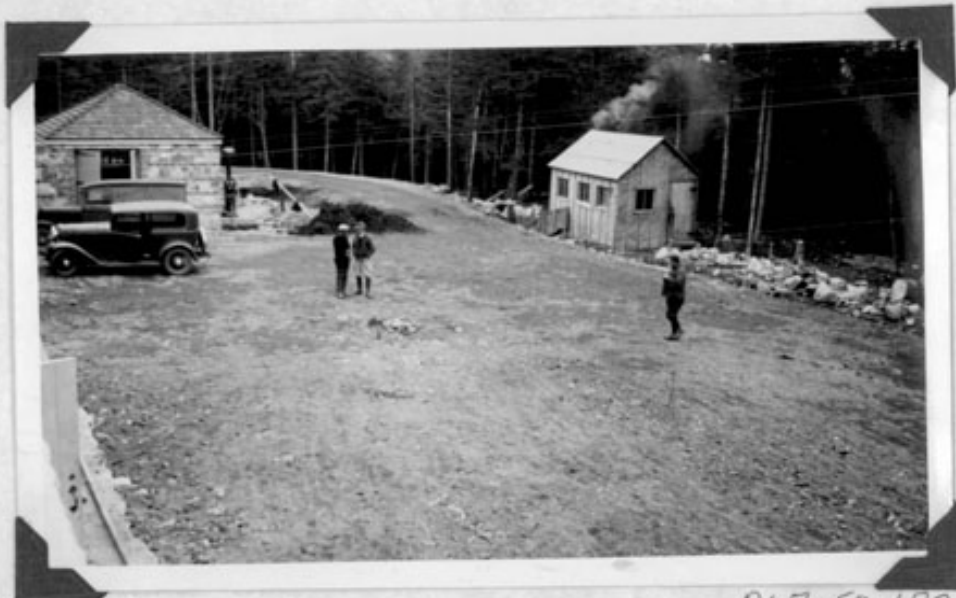
The service court after drainage and sub-grade had been completed in November, 1934.
