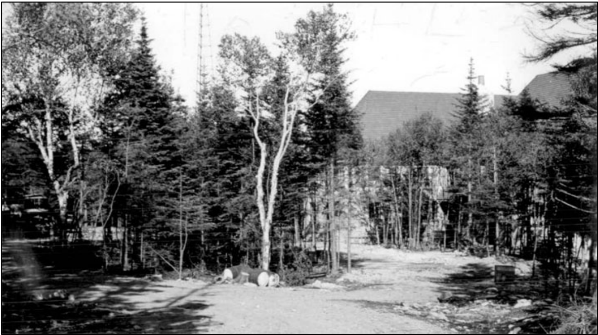
Figure 15. Apartment Building, NW elevation and courtyard, looking NE, before selective tree cutting and landscaping, October 1934.
