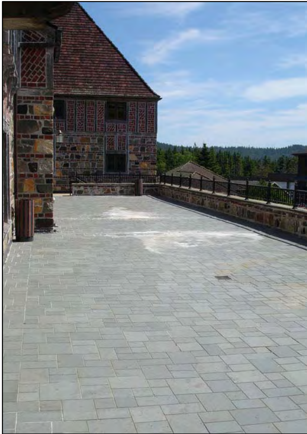
Figure 51. Apartment Building, SE elevation, terrace, 2008.
