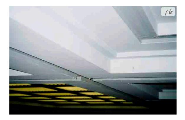
Figure 6. View across ceiling showing drips ("stalactites") of sprayed-on recent thick coating.
