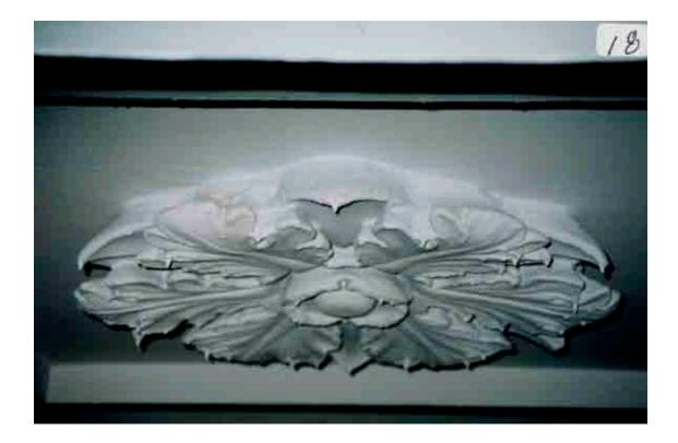
Figure 7. View of ceiling rosette showing drips of sprayed-on thick coating. Typical of all ceiling rosettes.
