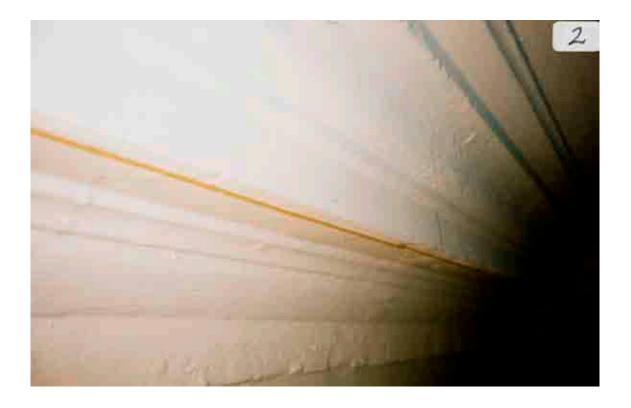
Figure 2. Cornice repair work along the north wall. Again, note poor repair of moulding profile.
