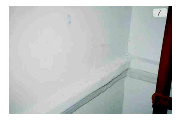
Figure 1. View of picture moulding repair work in the northeast corner. Note poor resolution of profile.
